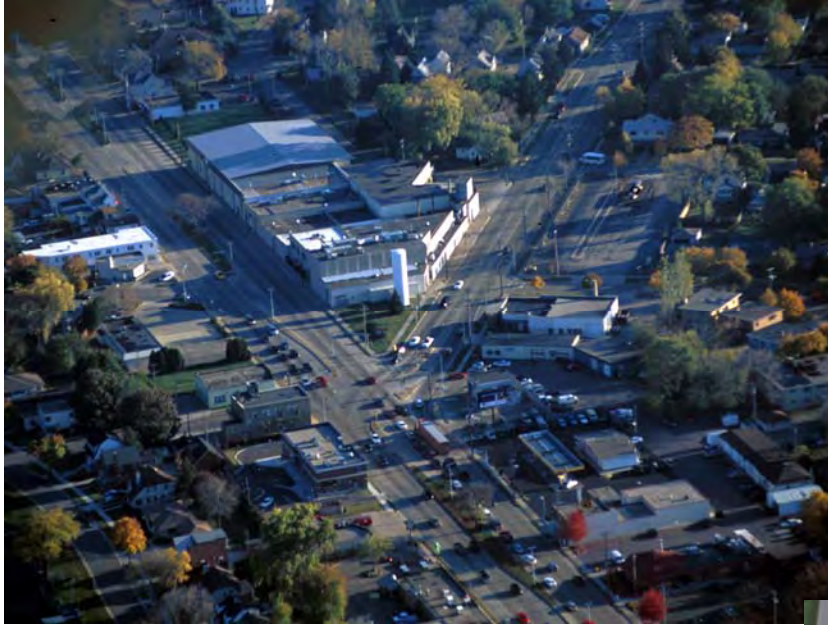
View of Dean/Morningstar Dairy site (looking south) at the intersection of South Park Street and Fish Hatchery Road. The building has been vacant since June 2004. Manufacturing equipment and other mechanicals have been removed from the building/site.
