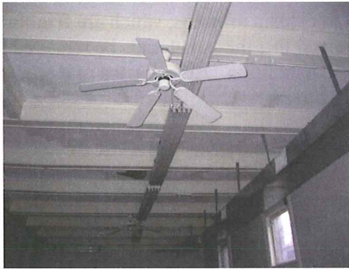
First floor lights.
