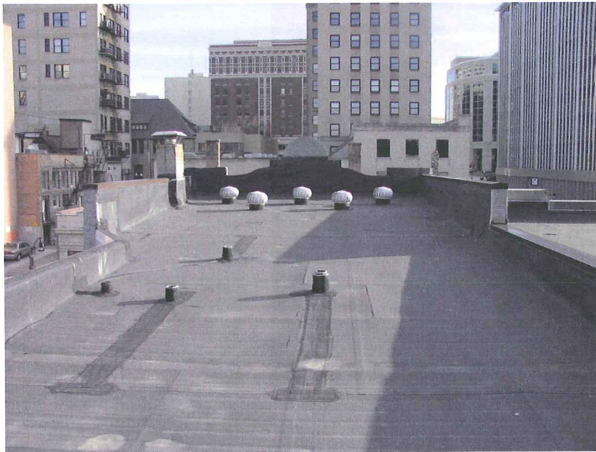
Figure 10. Overview of the roof.
