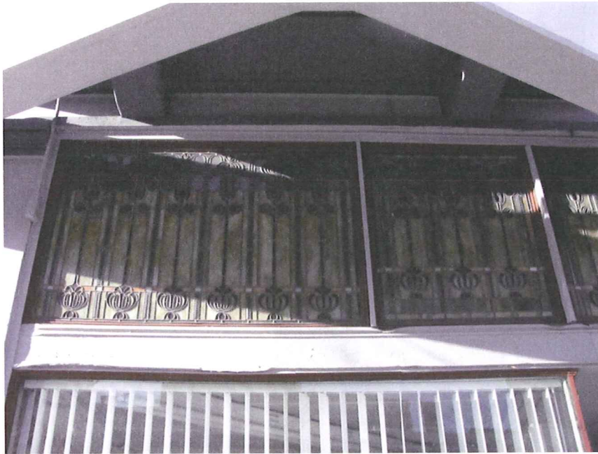
Figure 4. The first floor storefront includes a three-part leaded art glass transom.
