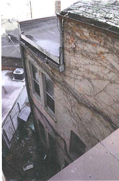
View of the back of facade
