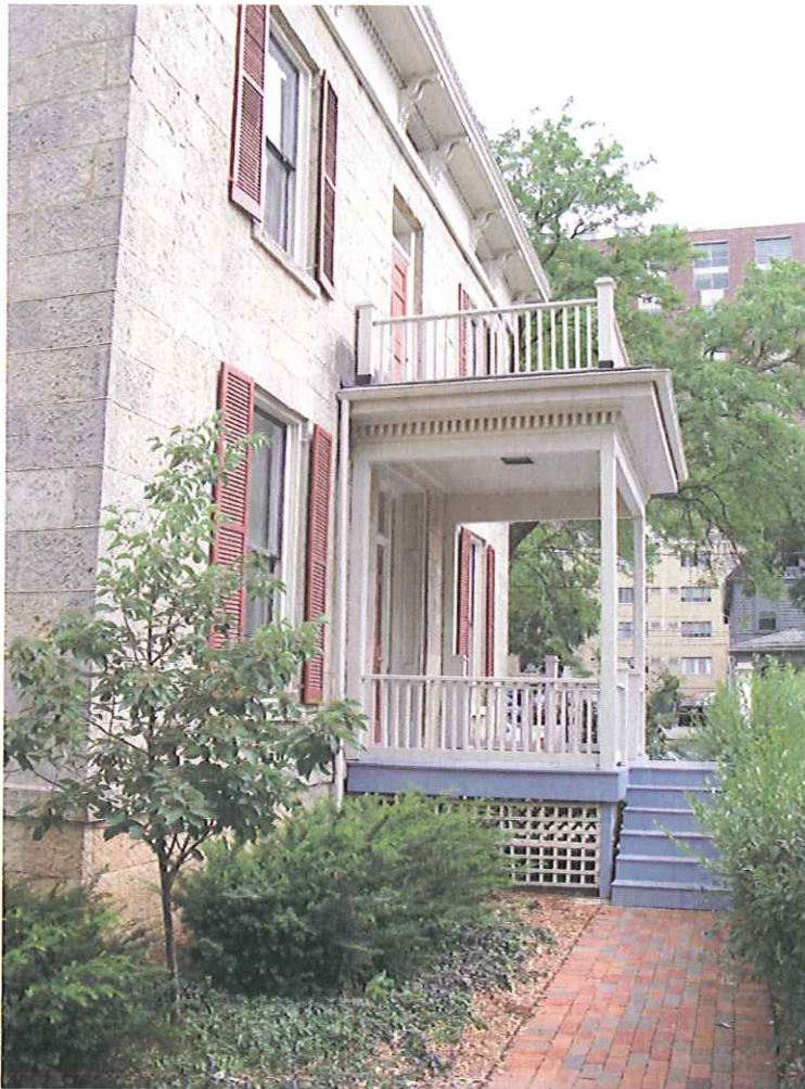
Existing Conditon at Rear Entrance
