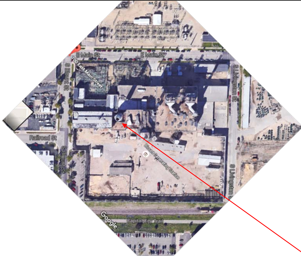
Google aerial view. Exhaust stack proposed for demolition at this time indicated by arrow.
