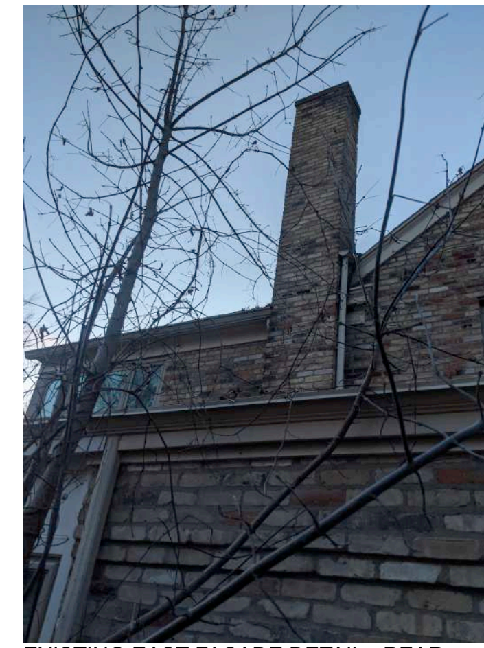
EXISTING EAST FACADE DETAIL - REAR CHIMNEY PROPOSED TO BE DEMOLISHED
