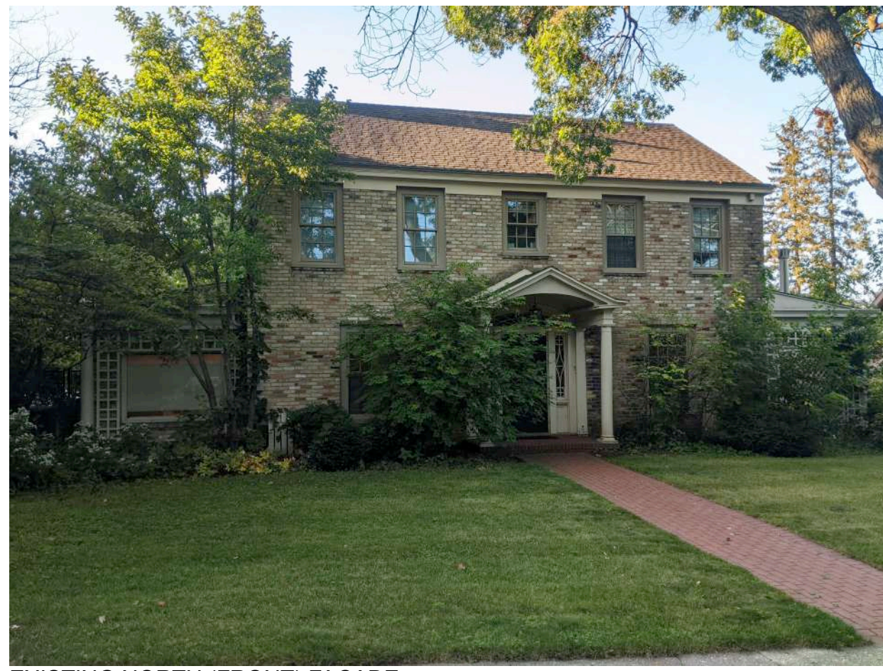
EXISTING NORTH (FRONT) FACADE
