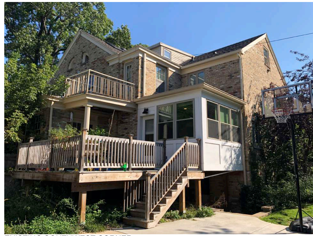
EXISTING SOUTHWEST CORNER -DETERIORATING 2ND FLOOR BALCONY WITH NARROW DOOR VISIBLE -AREA PROPOSED TO BE DEMOLISHED IN FAVOR OF NEW ADDITION -QUARTER ROUND WINDOWS AT UPPER-LEFT AND NARROW DOOR TO BALCONY TO BE REHABILITATED.
