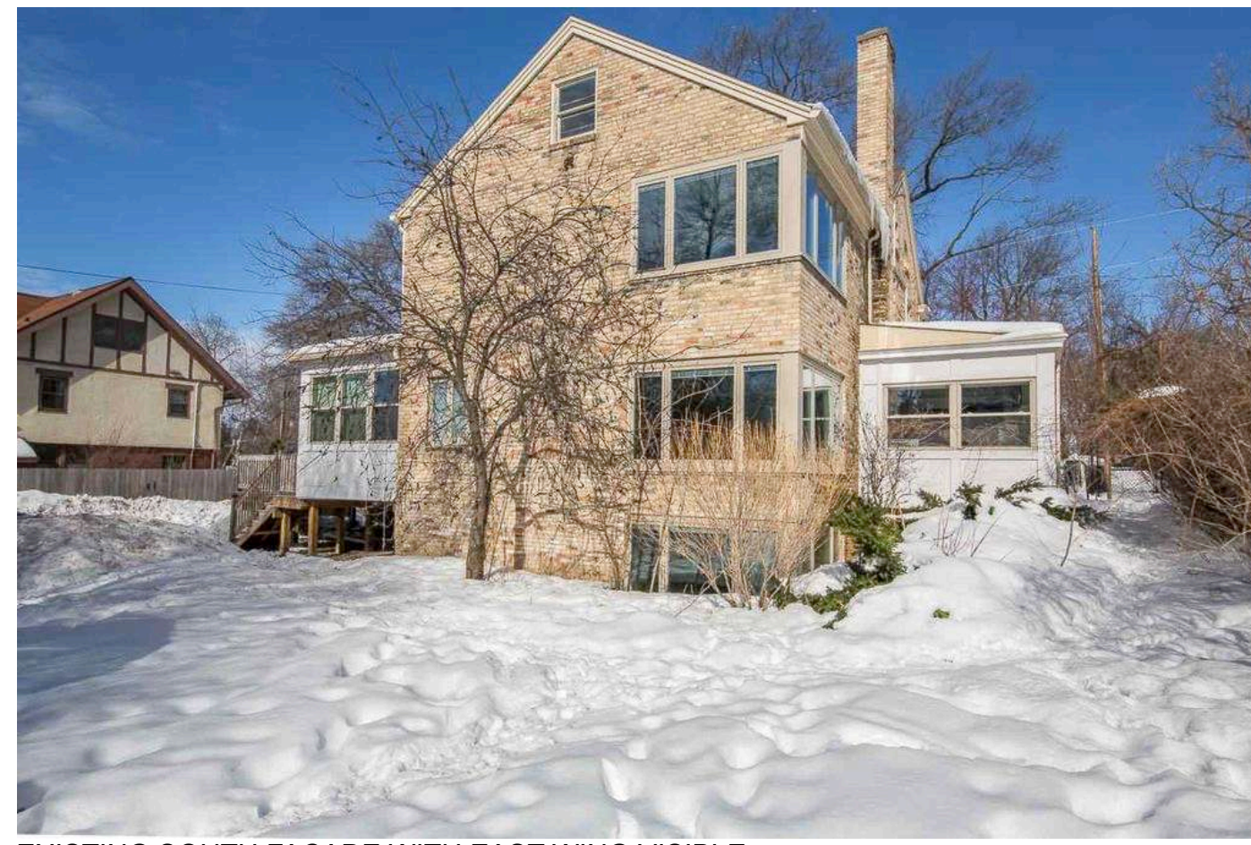
EXISTING SOUTH FACADE WITH EAST WING VISIBLE
