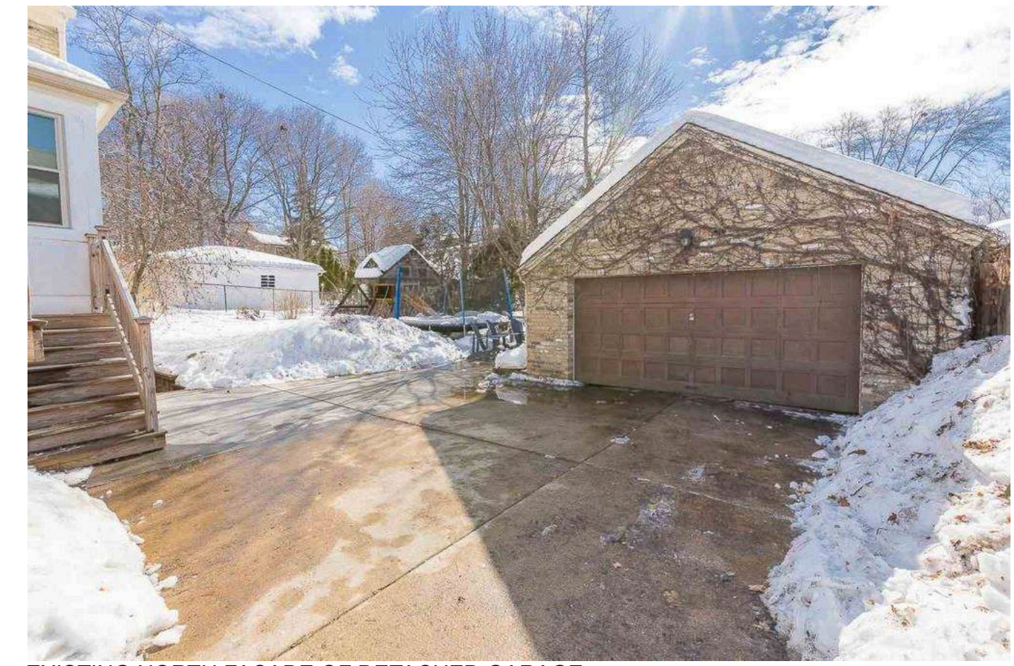
EXISTING NORTH FACADE OF DETACHED GARAGE
