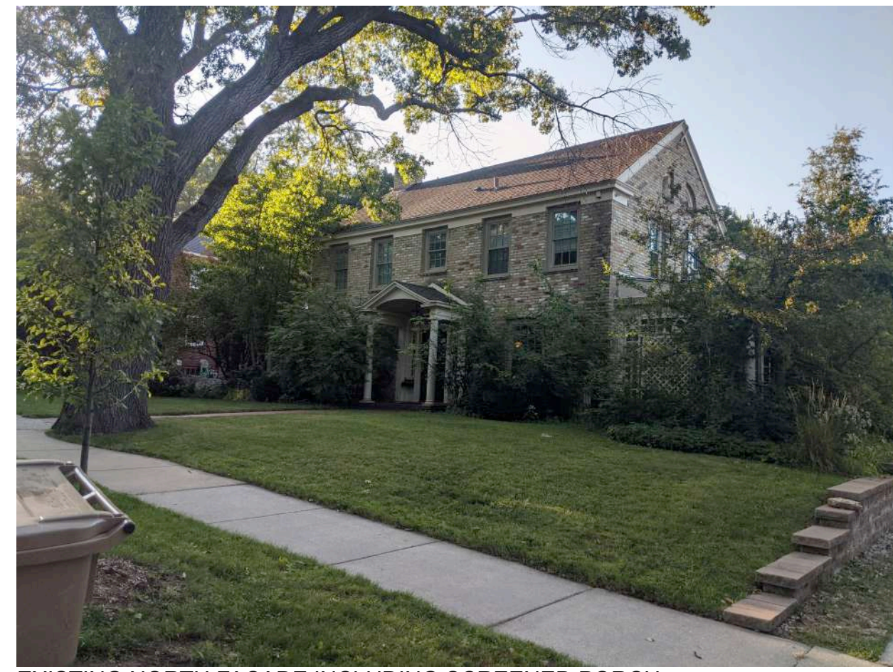
EXISTING NORTH FACADE INCLUDING SCREENED PORCH
