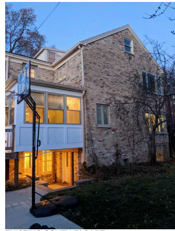
EXISTING SOUTH FACADE
