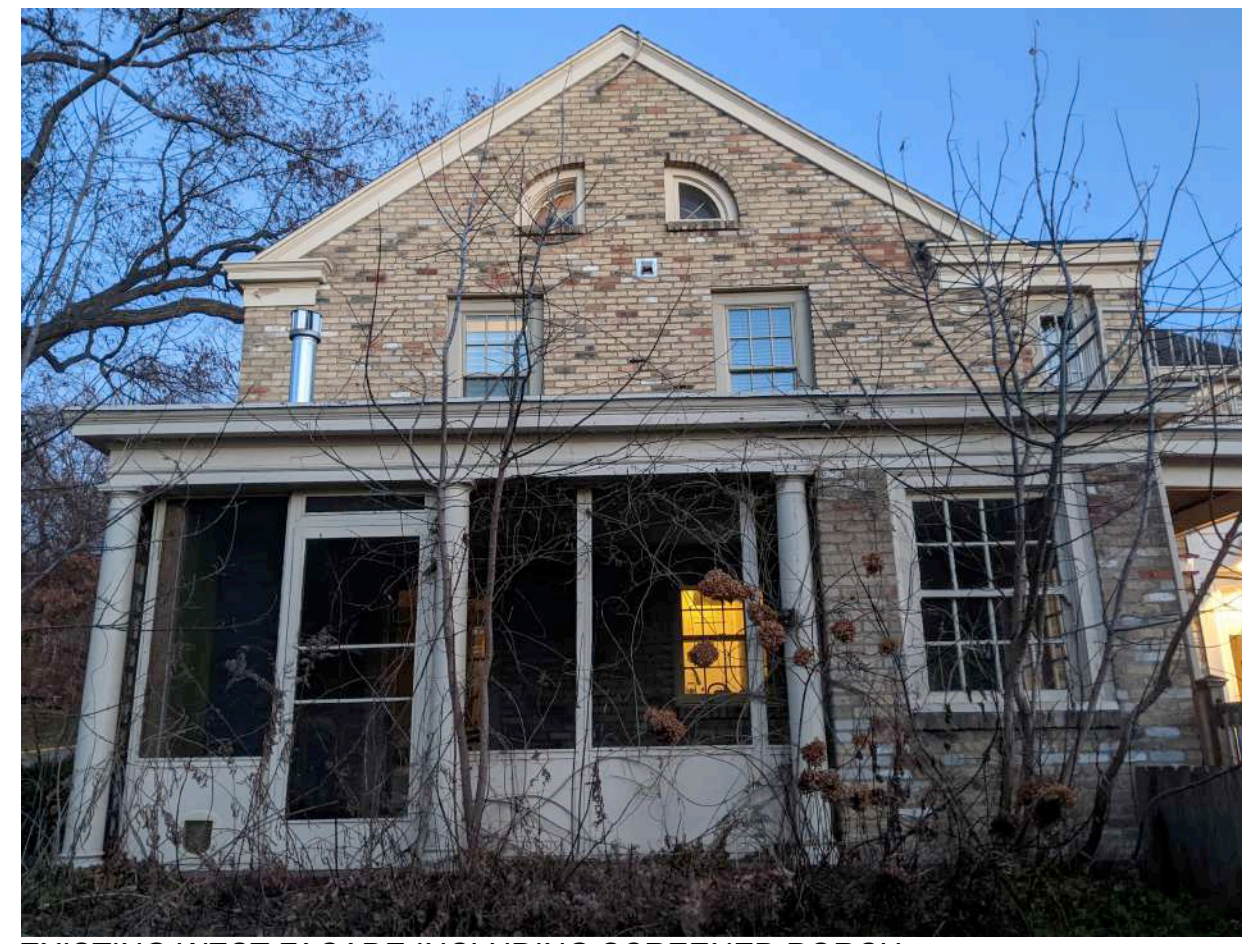
EXISTING WEST FACADE INCLUDING SCREENED PORCH -CONVERT TO WINDOW-FILLED CONDITIONED ROOM -REMOVE GAS STOVE AND ASSOCIATED FLUE -WINDOW ON RIGHT LOCATION OF NEW DOOR
