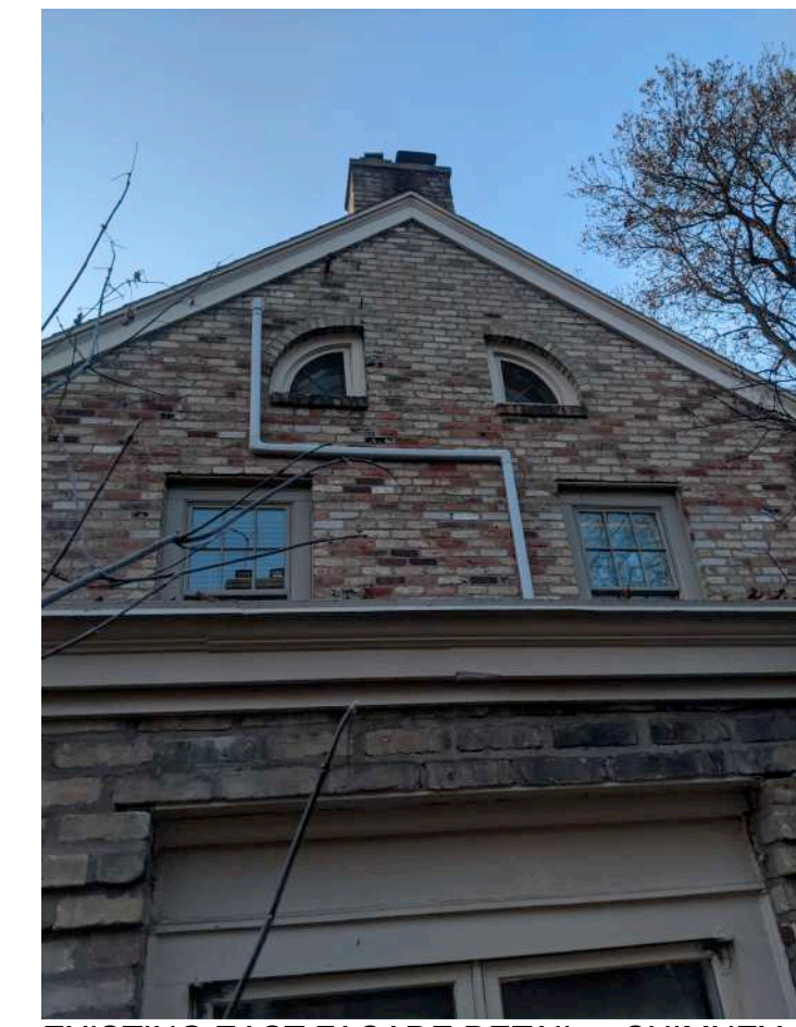
EXISTING EAST FACADE DETAIL - CHIMNEY AND CAP TO BE RESTORED, QUARTER ROUND WINDOWS TO BE REHABILITATED, AND HVAC CONDUIT TO BE ELIMINATED
