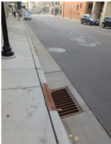
Fairchild at West Washington looking west (overall good condition)
