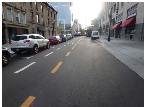
Main looking to Pinckney (overall good condition)
