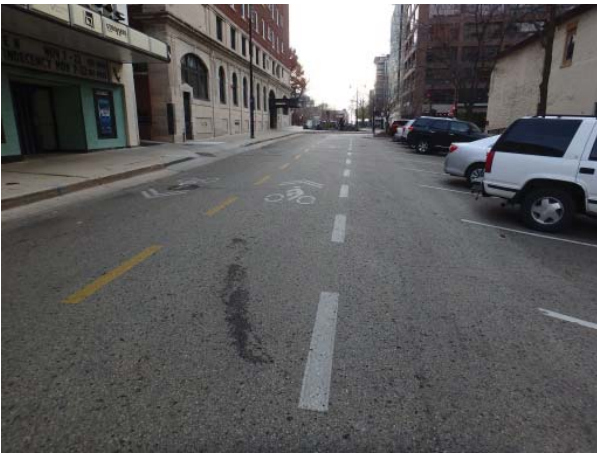
Mifflin looking towards the Capitol (some discoloration on road, overall good condition)
