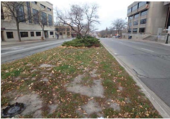
East Washington looking east (patching, cracks, dead patches of grass)
