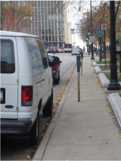
Carroll at State looking southeast (rusted parking meters)
