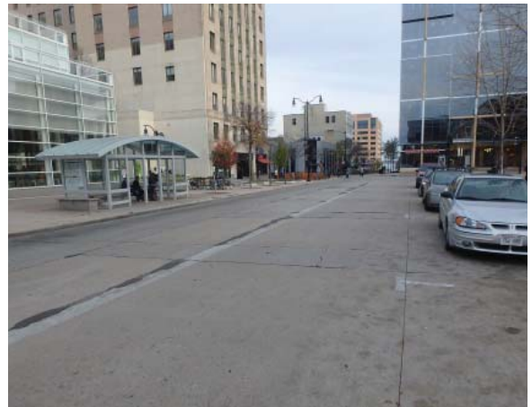
Pinckney looking to Martin Luther King Jr. (cracks, patching, fading)
