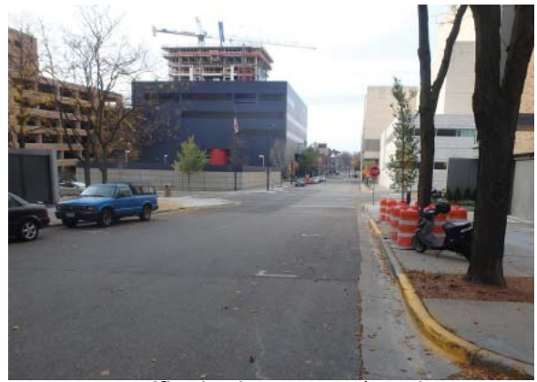
Henry at Mifflin looking West (cracking, patching, curb paint fading)
