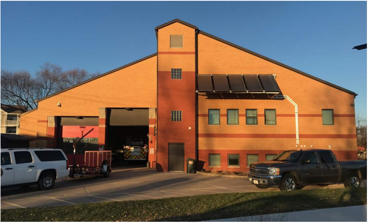
Fire Station 6 south elevation facing adjacent property.
