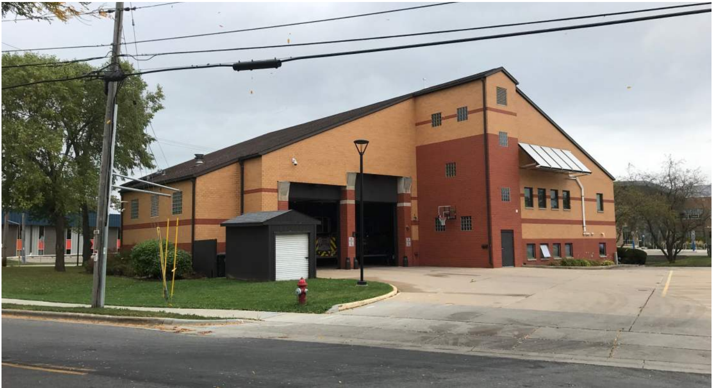
Fire Station 6 west and south elevations facing Perry Street.
