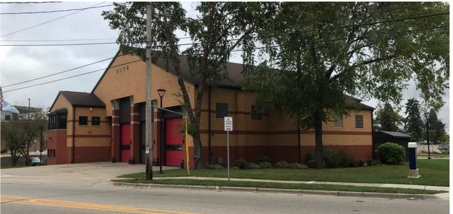
Fire Station 6 front and west side elevations facing West Badger Road and Perry Street.
