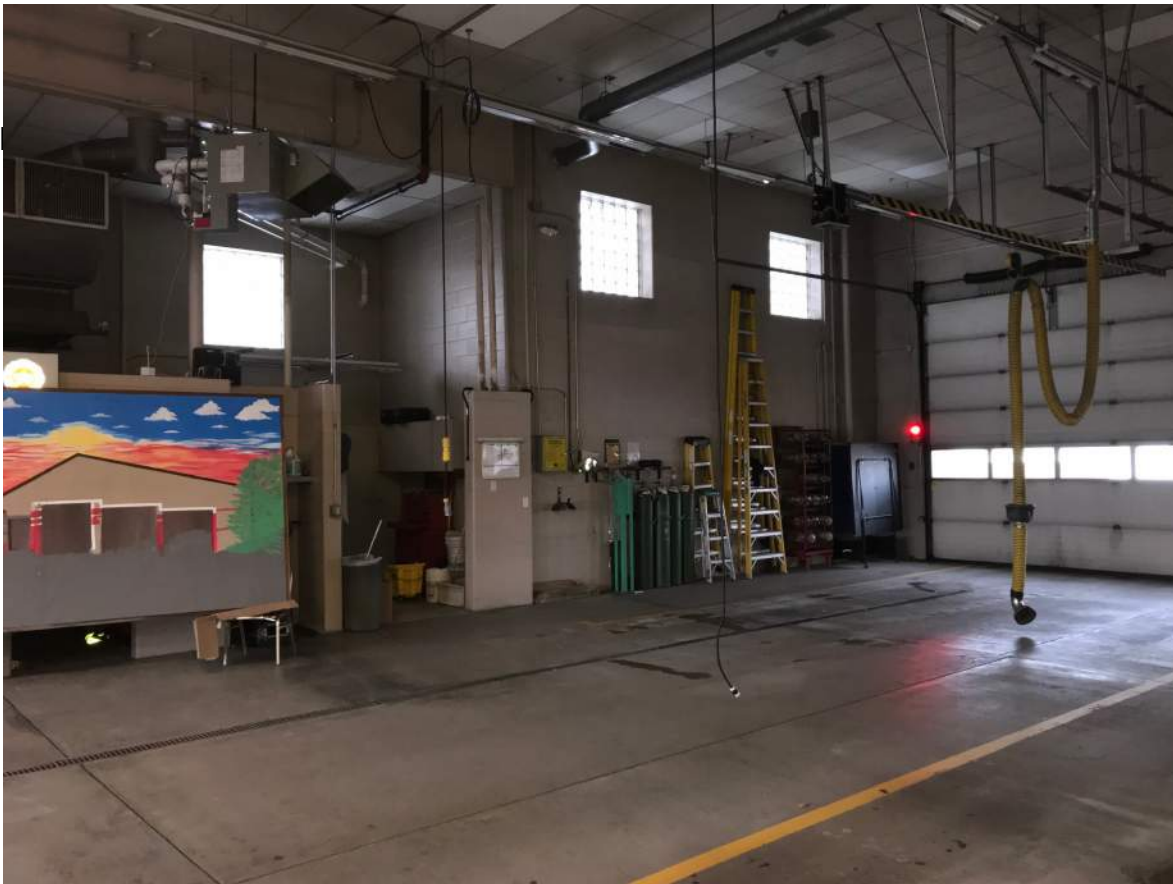
Fire Station 6 interior of apparatus bay facing west. Exterior wall to be removed to accommodate proposed addition.
