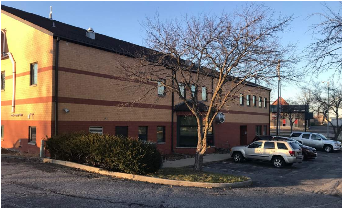
Fire Station 6 south and east elevations facing the adjacent property.
