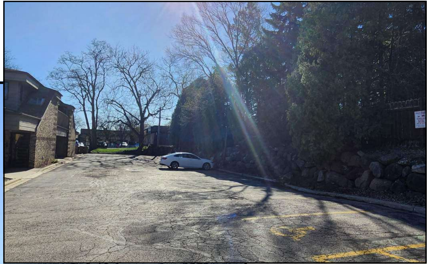
EAST BUILDING PARKING LOT 3535 UNIVERSITY AVENUE
