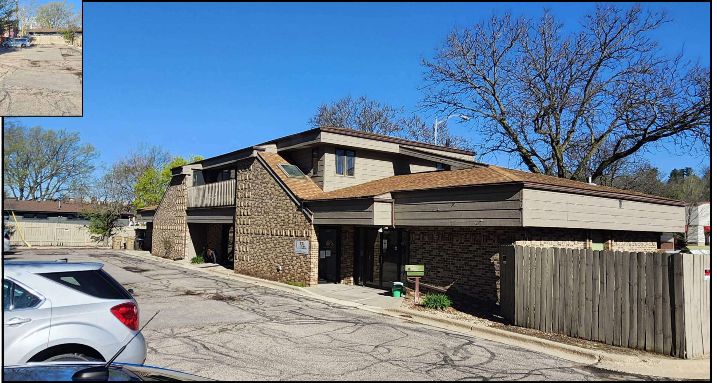
WEST BUILDING - REAR
