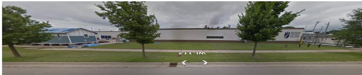
VIEW OF BUILDING B FROM PACKERS AVE
