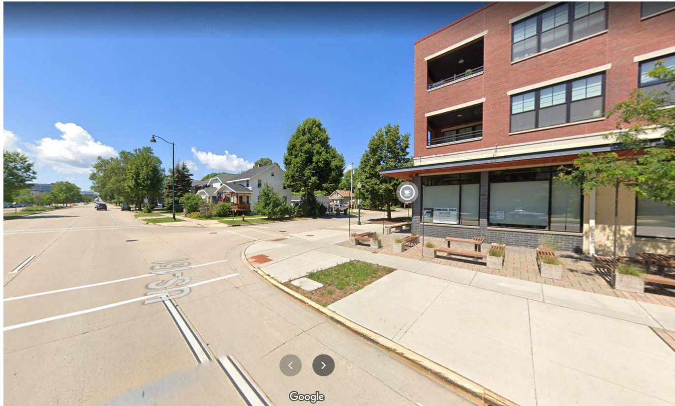
South West view looking at corner of East Washington and North Few Street
