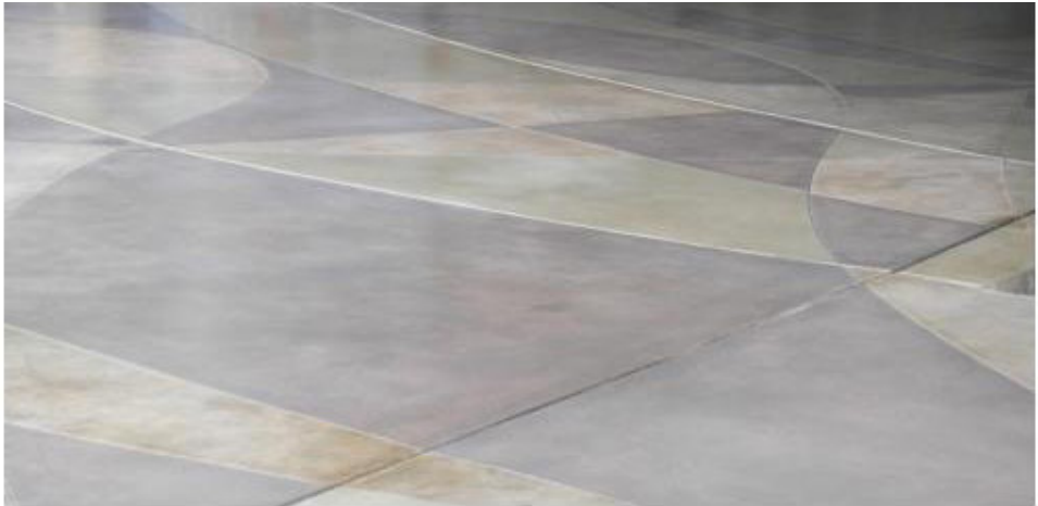
Stained Concrete to create band pattern
