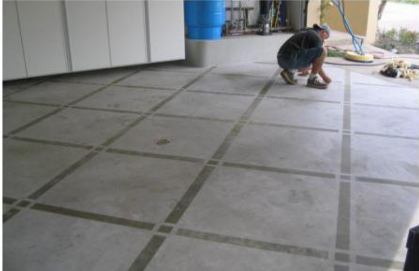
Stained Concrete to create band pattern
