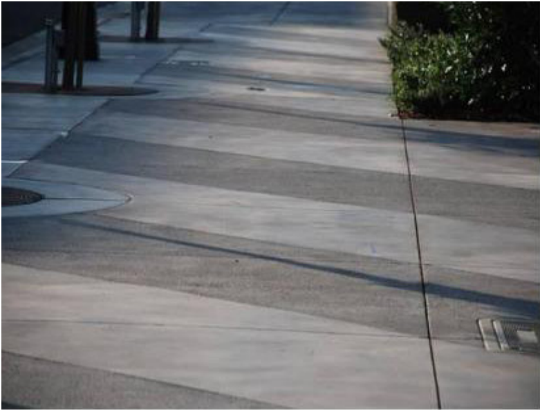
Stained Concrete to create band pattern
