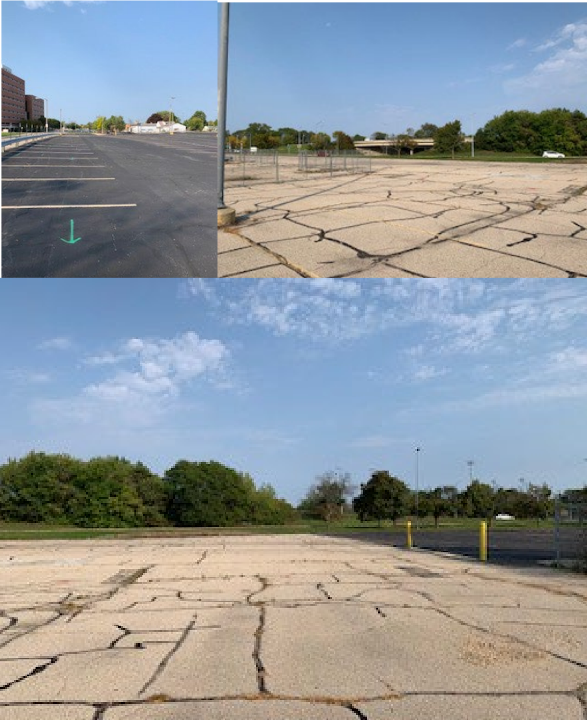
Figure 6. Former Filling Station Site covered by Parking lot
