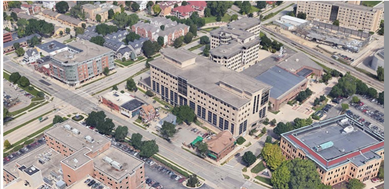
aerial view looking northwest
