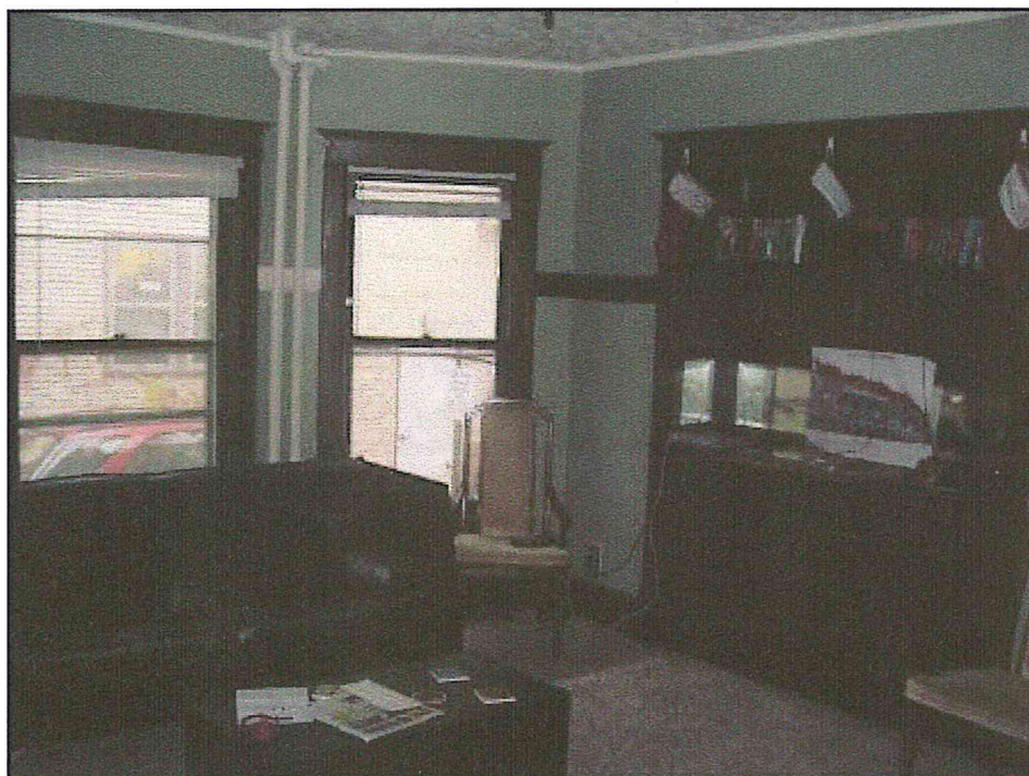
210 Bernard Court. Typical common area. Pipes in background are painted steel with no wrapping material.
