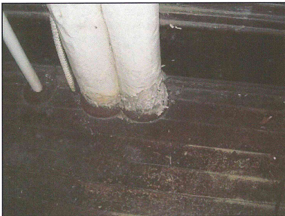
210 Bernard Court. Looking at possible asbestos wrapped pipes in front entry way.
