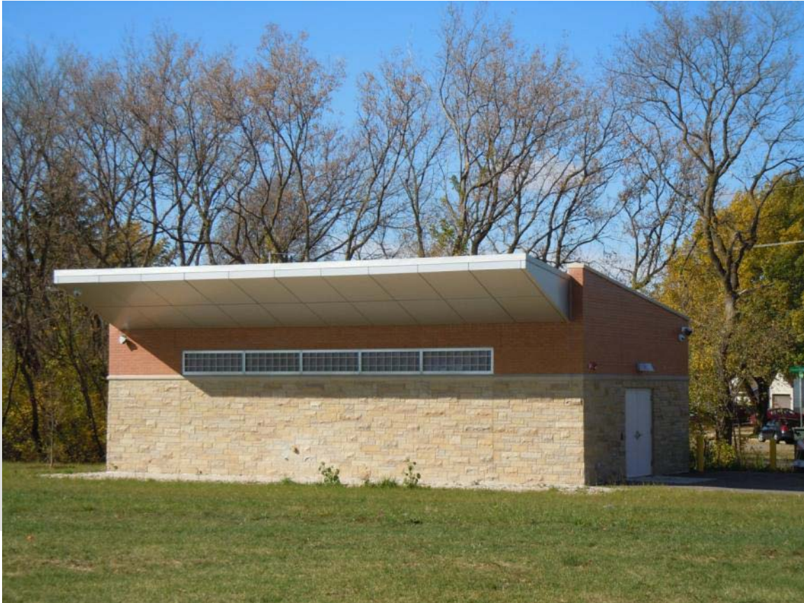
NEW BOOSTER STATION AT LEOPOLD PARK
