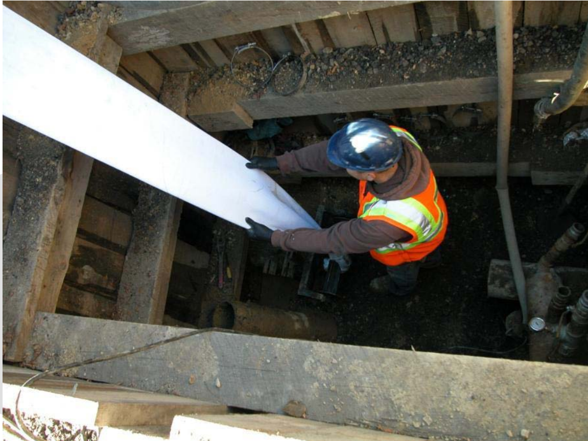
WATER MAIN LINING PROJECT ON DROSTER ROAD
