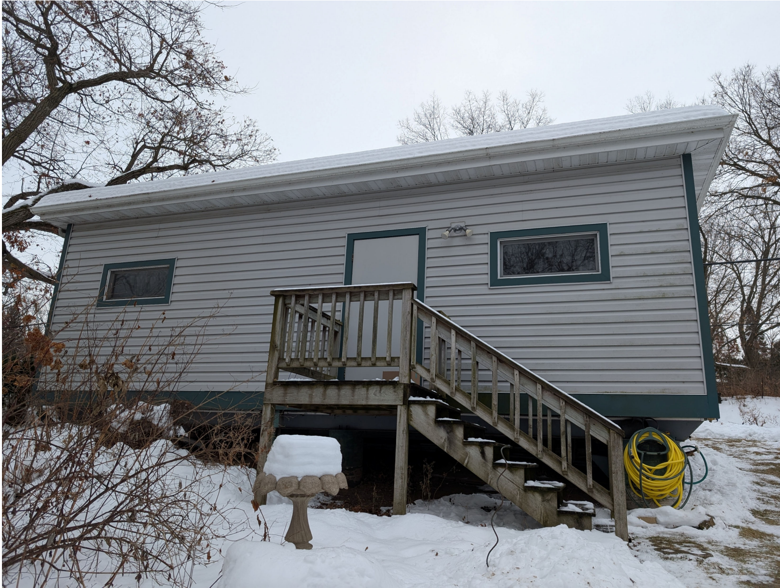
Rear of Garage, Looking Towards Lake Mendota Dr
