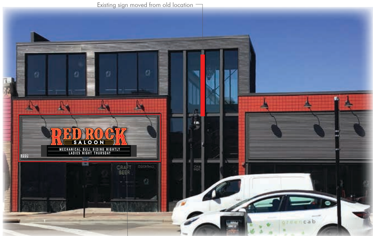
Existing sign moved from old location
