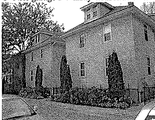
Looking approx. south from O'Niel home
