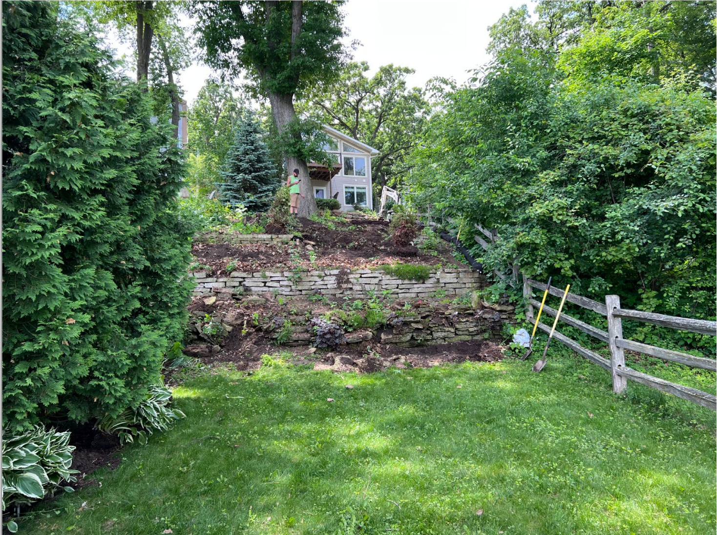
RETAINING WALLS BEFORE REBUILDING
