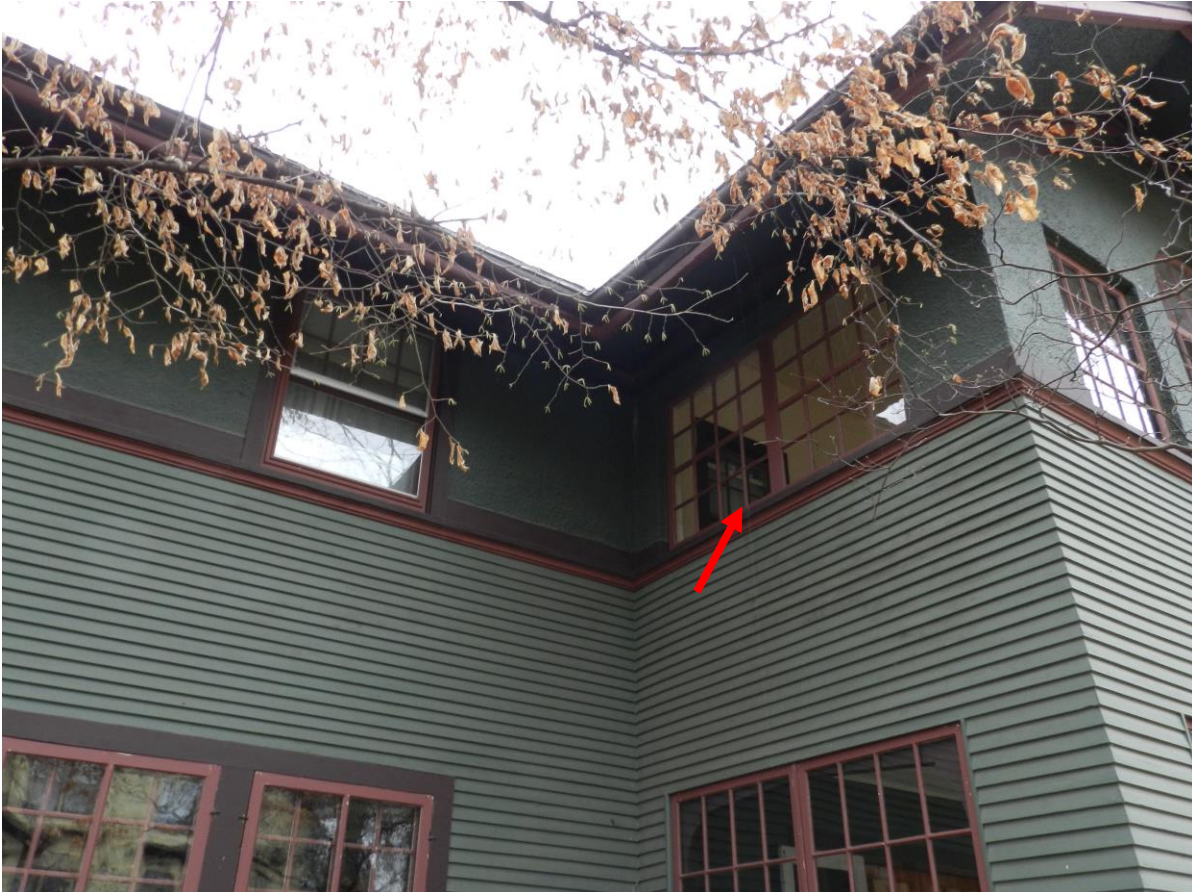
East side upper porch windows to be replaced
