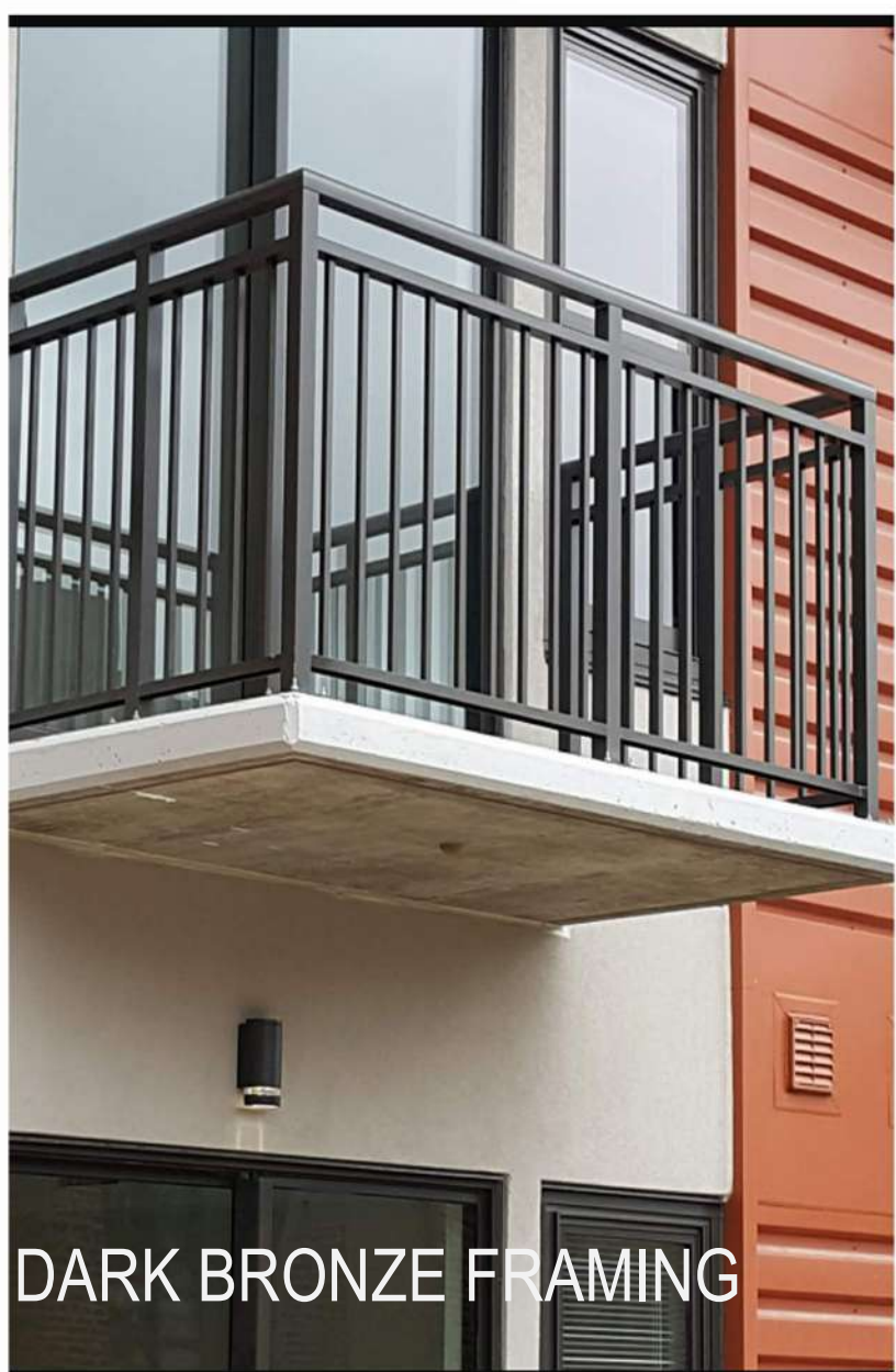
GUARDRAIL ASSEMBLY - ALUM PICKETS
