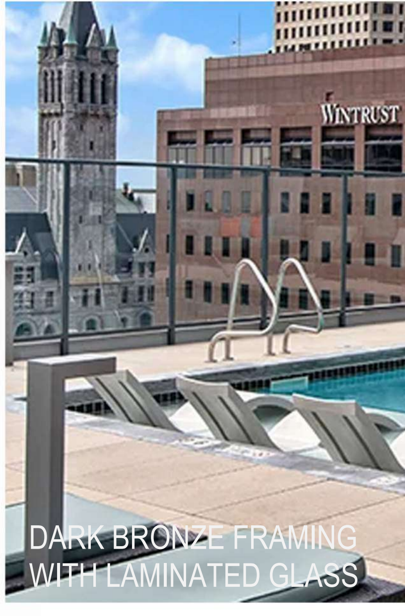
GLASS GUARDRAIL ASSEMBLY
