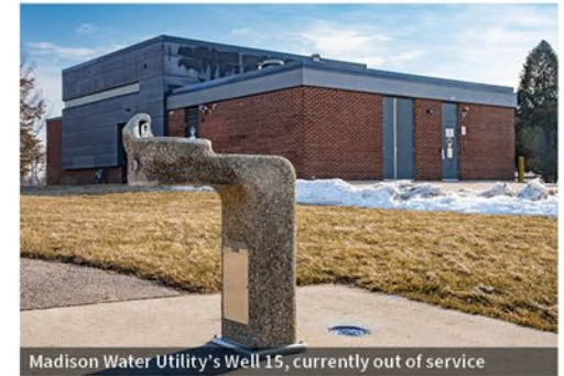
Madison Water Utility's Well 15, currently out of service
