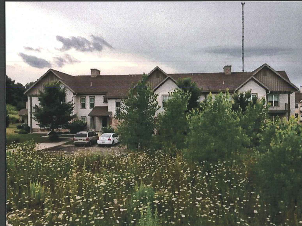
12 UNIT CONDEO, HILLSIDE ESTATES
