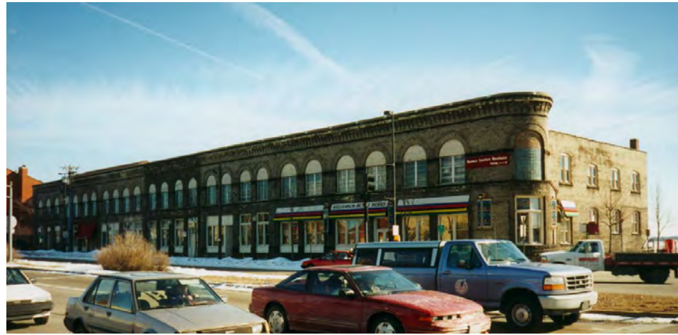
View Prior to Renovation
