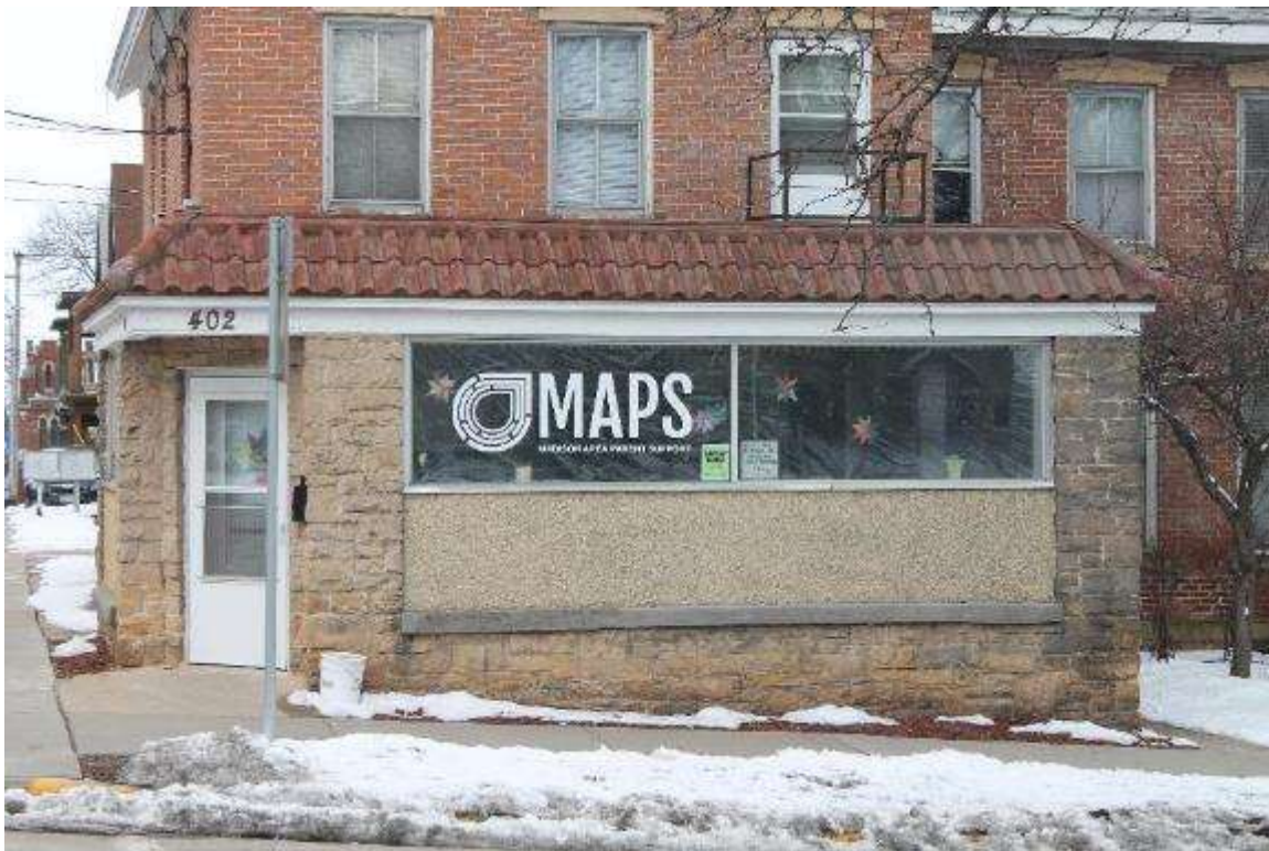
Photo 134: 402-408 East Washington Avenue, Exterior, facing northwest
