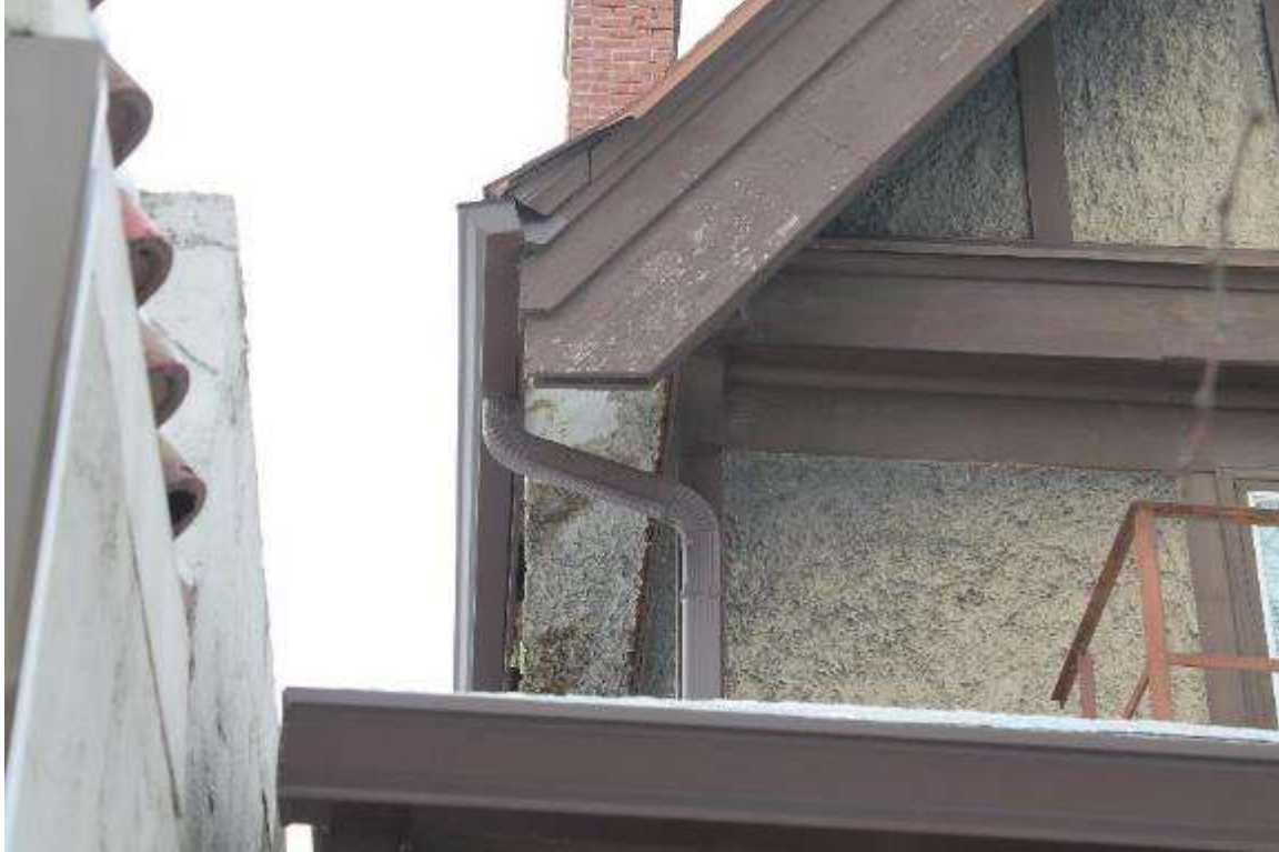
Photo 235: 410 East Washington Avenue, Exterior, facing northwest
