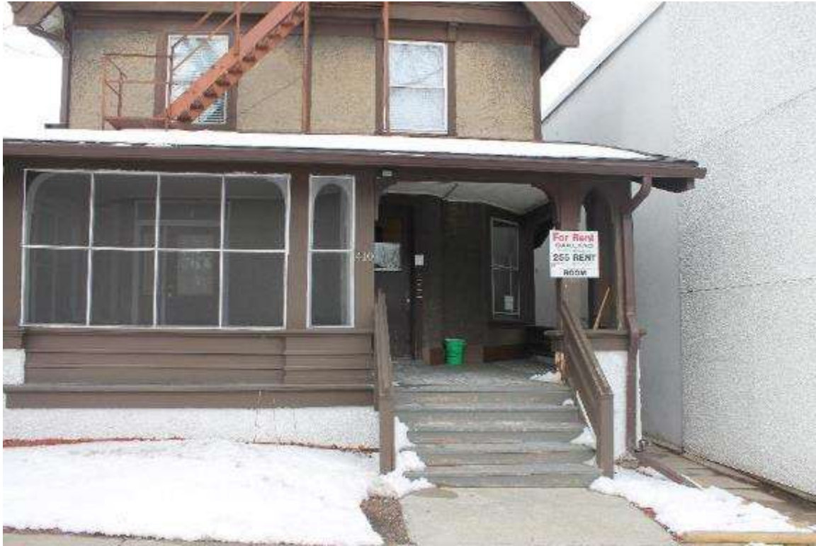
Photo 228: 410 East Washington Avenue, Exterior, facing northwest
