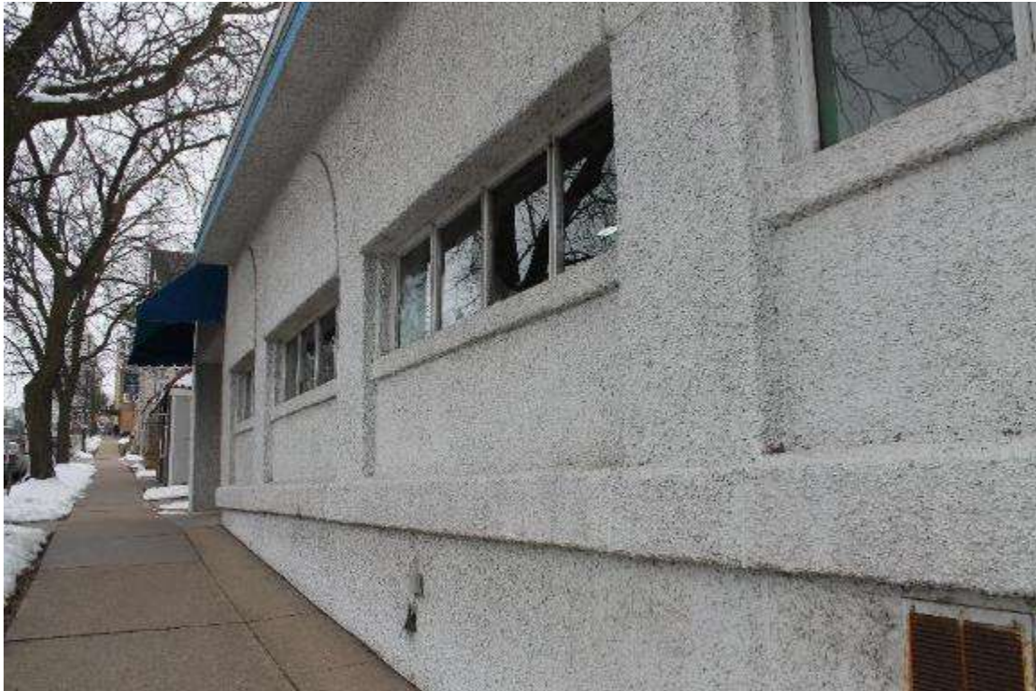
Photo 338: 412-414 East Washington Avenue, Exterior, facing southwest
