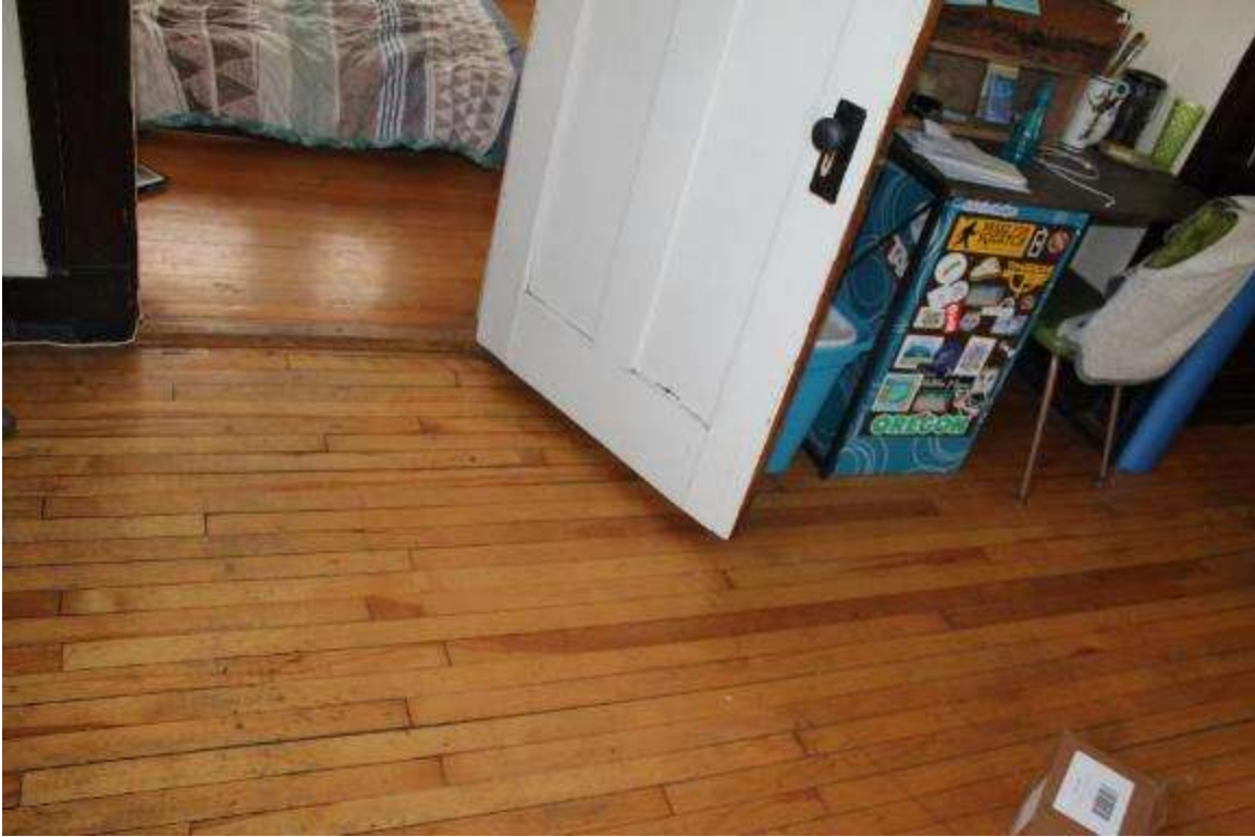
Photo 287: 410 East Washington Avenue, Interior, first floor unit 2
