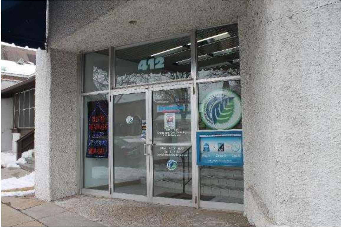
Photo 340: 412-414 East Washington Avenue, Exterior, facing northwest
