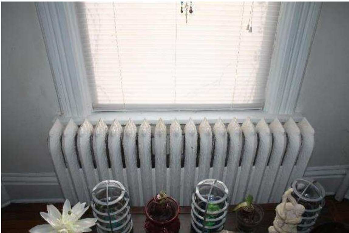
Photo 22: 9 North Hancock Street, Interior, first floor unit 1
