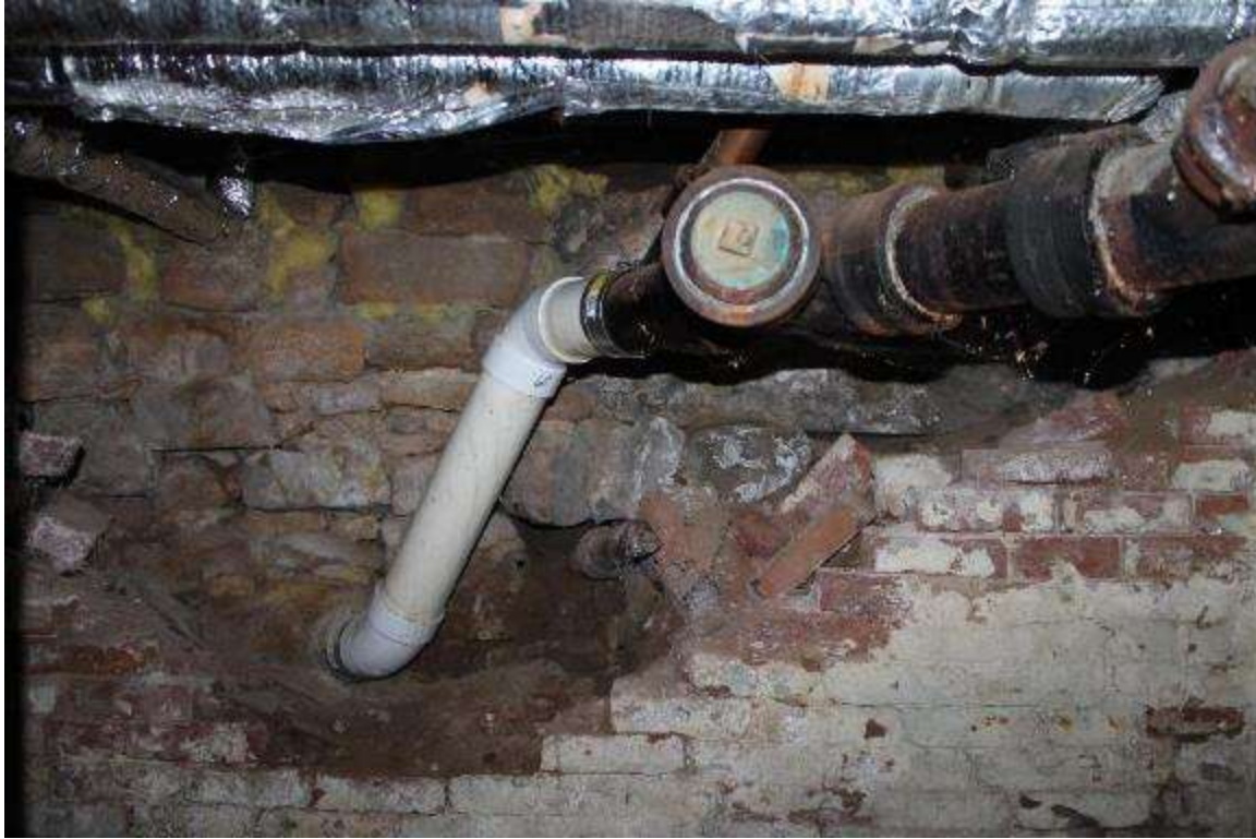
Photo 129: 12 North Franklin Street, Interior, basement
