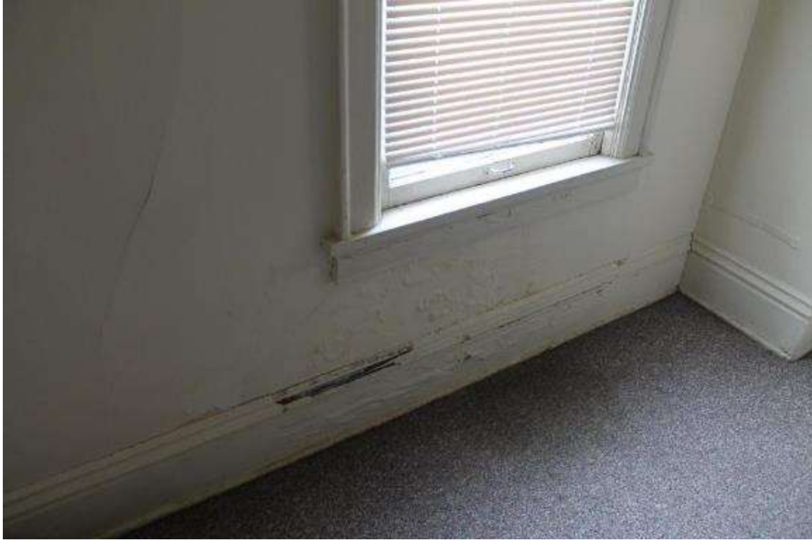
Photo 73: 8-10 North Franklin Street, Interior, first floor unit 1
