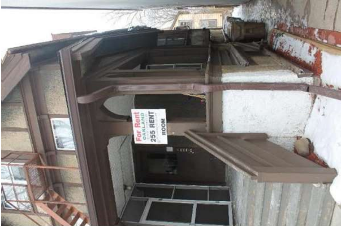
Photo 230: 410 East Washington Avenue, Exterior, facing west
