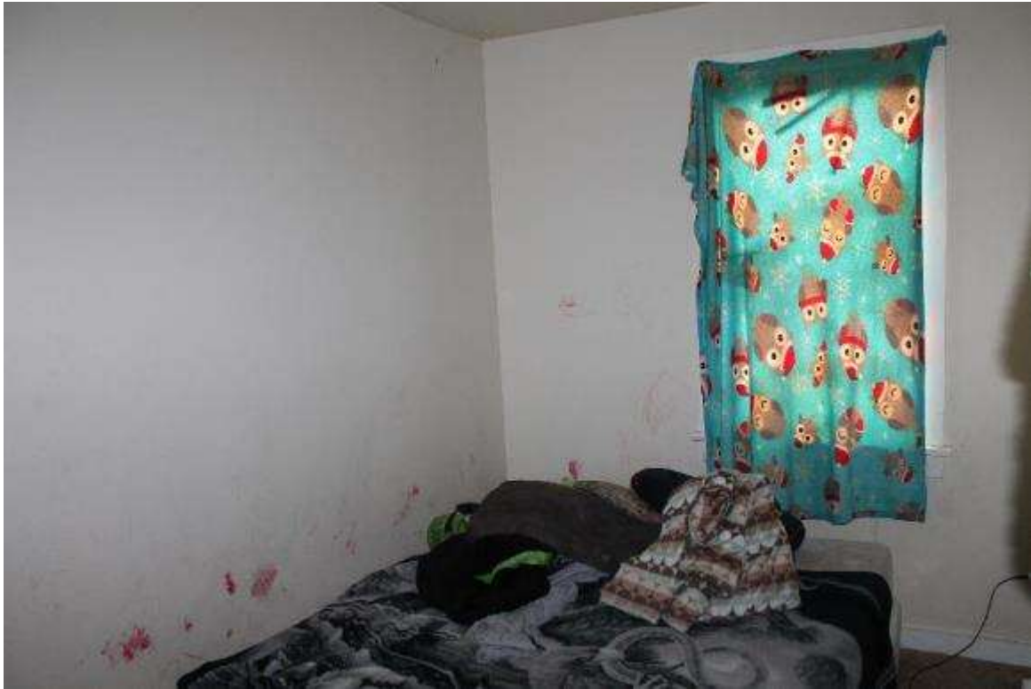
Photo 116: 12 North Franklin Street, Interior, first floor unit 1
