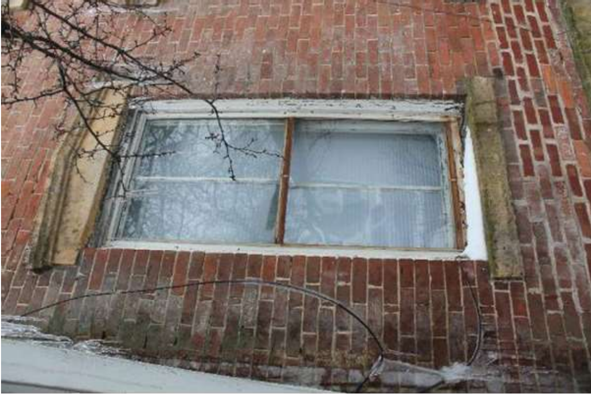
Photo 155: 402-408 East Washington Avenue, Exterior, facing northwest
