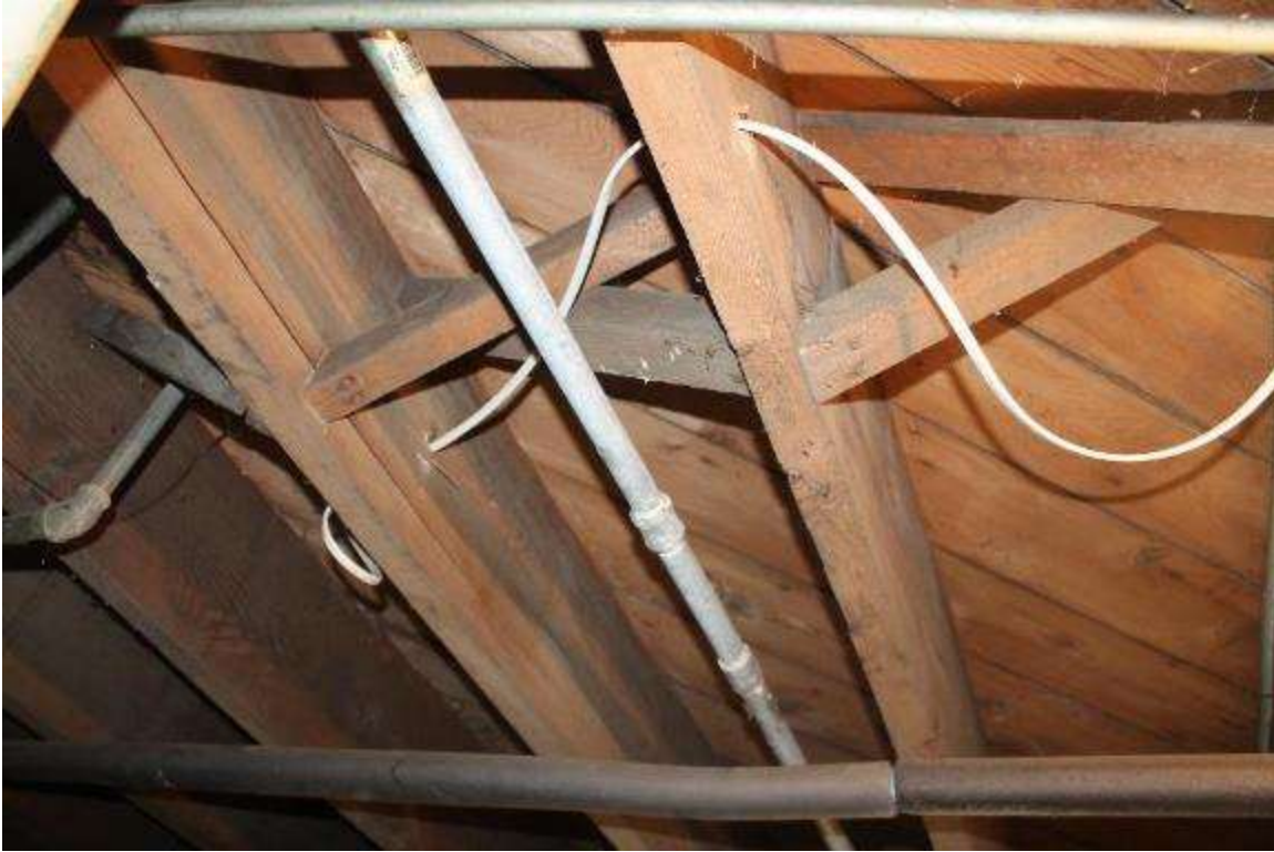
Photo 293: 410 East Washington Avenue, Interior, basement
