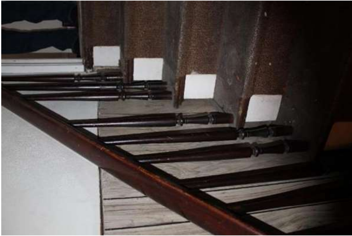
Photo 208: 402-408 East Washington Avenue, Interior, second floor stairs
