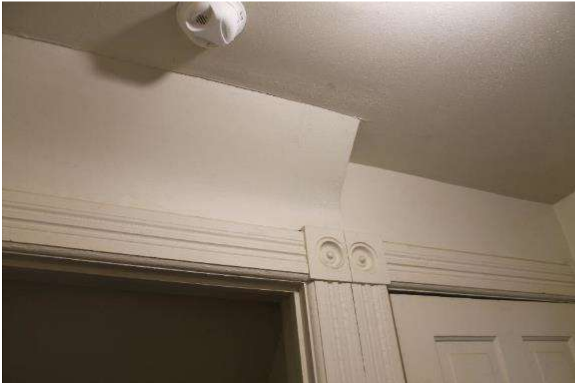
Photo 28: 9 North Hancock Street, Interior, first floor unit 1
