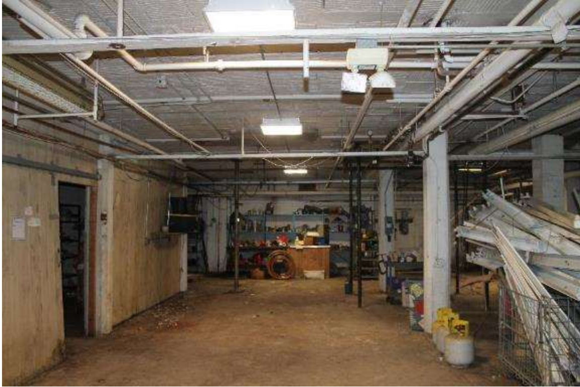
Photo 361: 412-414 East Washington Avenue, Interior, lower level storage space
