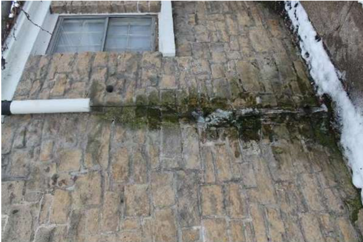
Photo 152: 402-408 East Washington Avenue, Exterior, facing west
