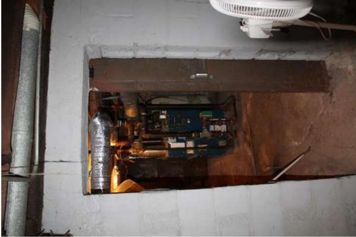
Photo 219: 402-408 East Washington Avenue, Interior, basement
