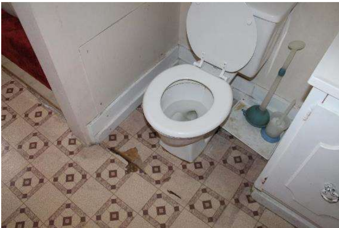
Photo 282: 410 East Washington Avenue, Interior, third floor unit 7
