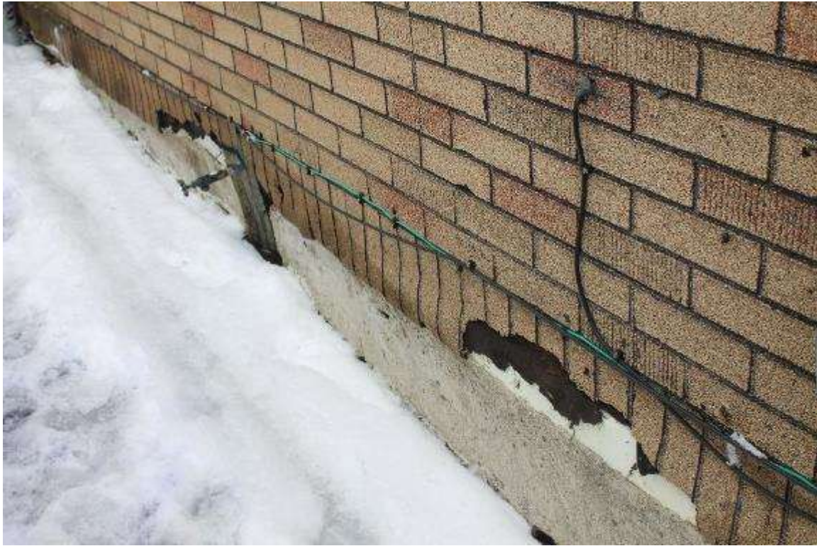
Photo 106: 12 North Franklin Street, Exterior, facing west
