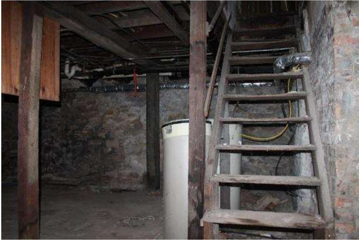
Photo 220: 402-408 East Washington Avenue, Interior, basement
