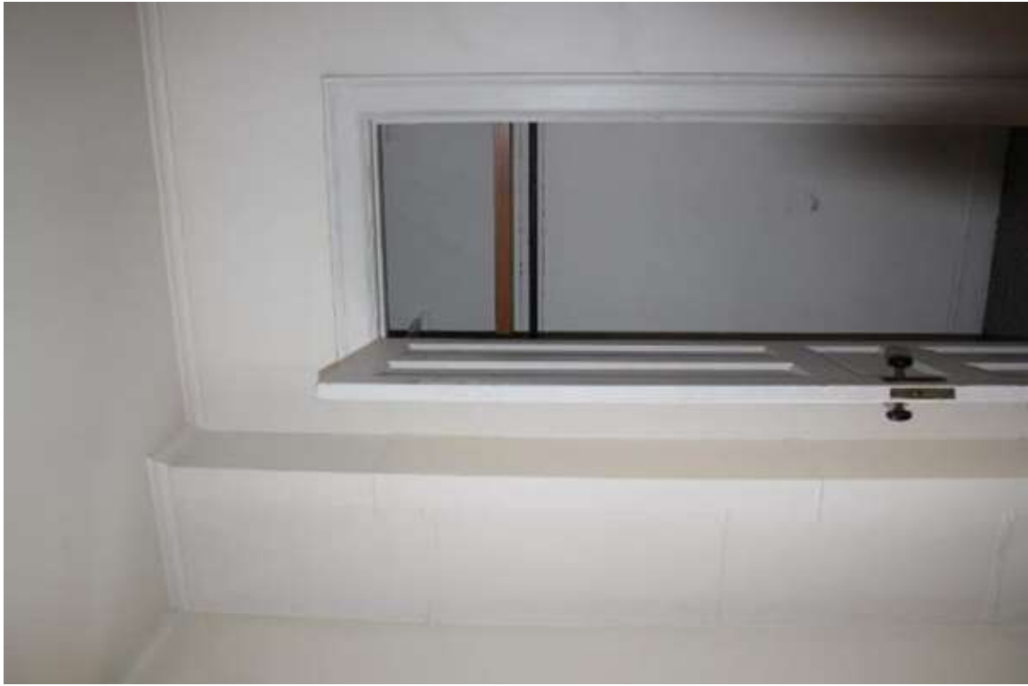
Photo 74: 8-10 North Franklin Street, Interior, first floor unit 1
