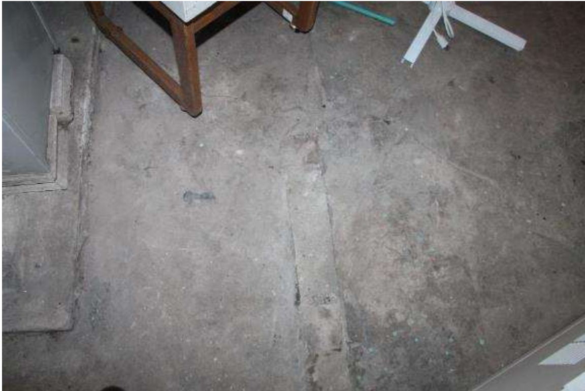
Photo 100: 8-10 North Franklin Street, Interior, basement
