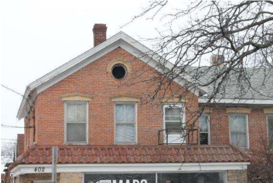
Photo 133: 402-408 East Washington Avenue, Exterior, facing northwest
