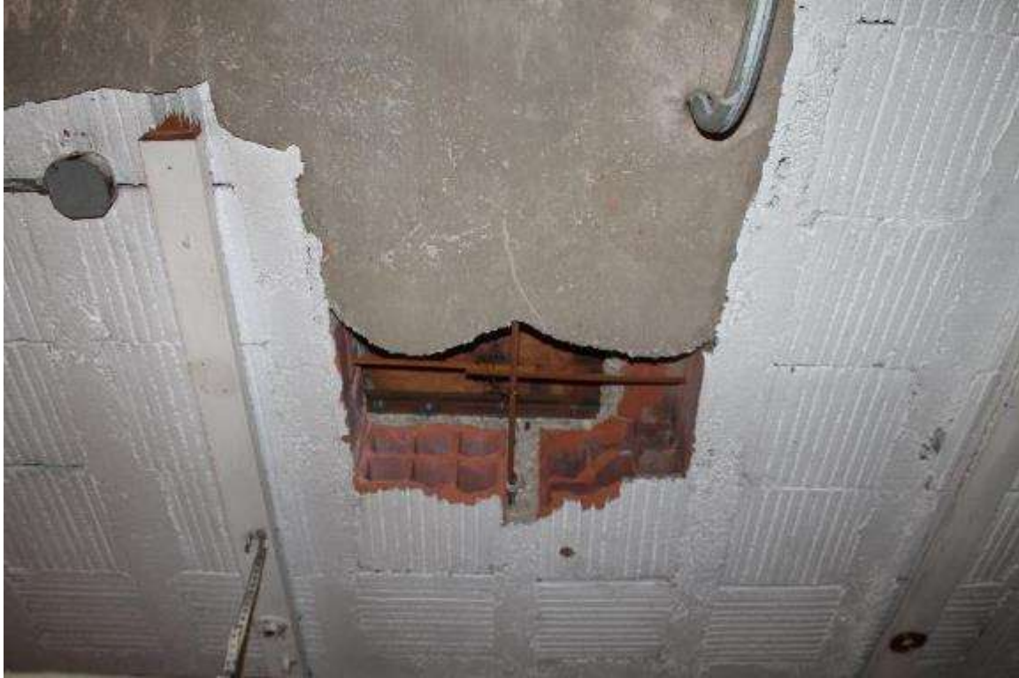
Photo 365: 412-414 East Washington Avenue, Interior, lower level storage space
