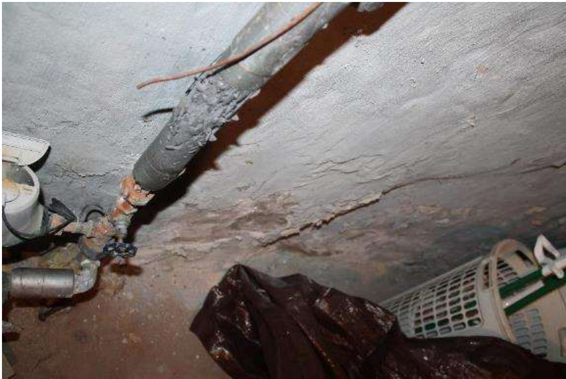
Photo 292: 410 East Washington Avenue, Interior, basement
