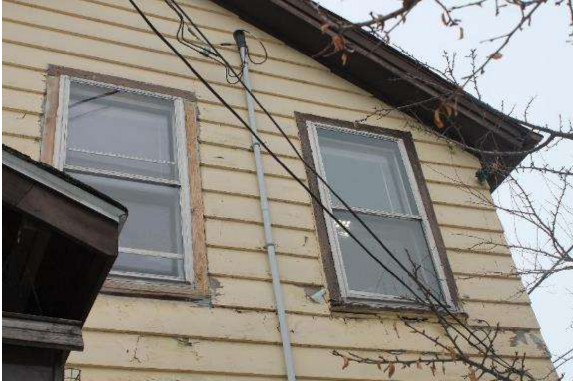
Photo 299: 410 1/2 East Washington Avenue, Exterior, facing northwest
