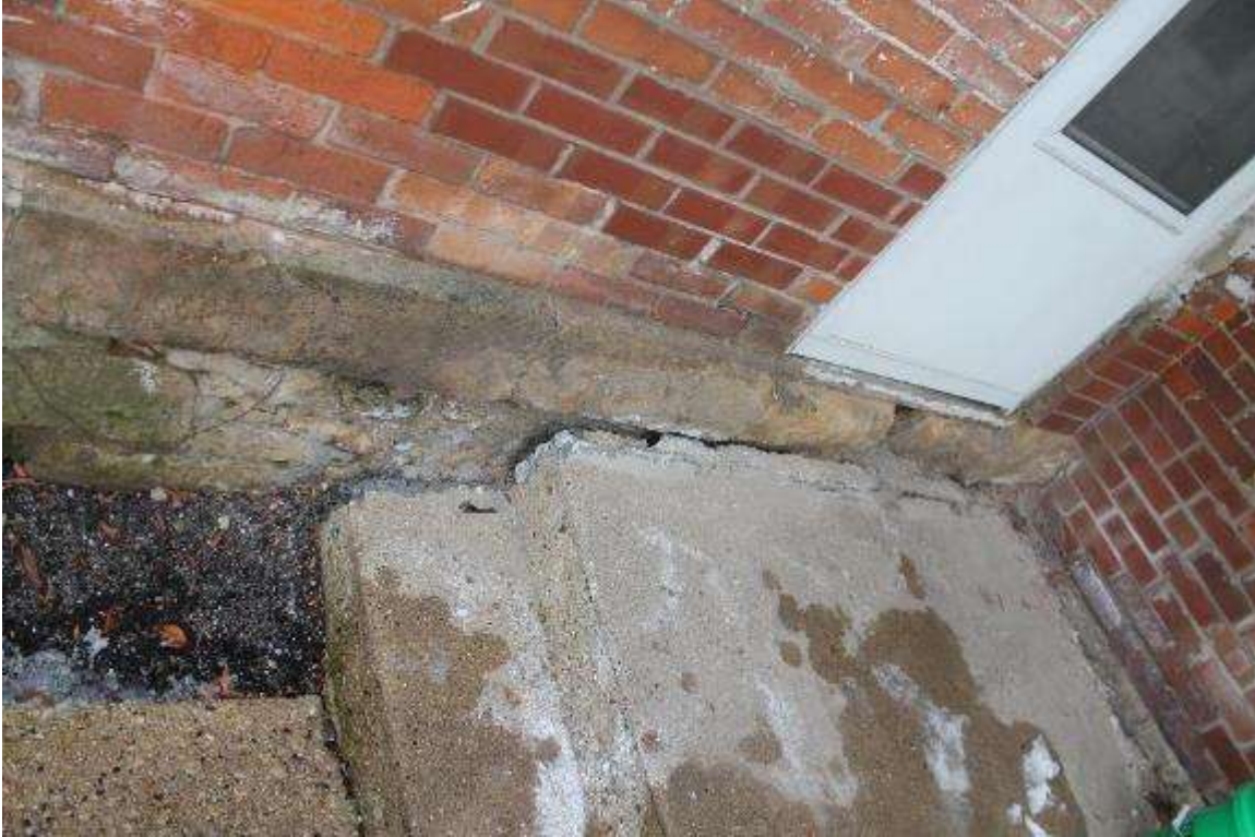
Photo 153: 402-408 East Washington Avenue, Exterior, facing west
