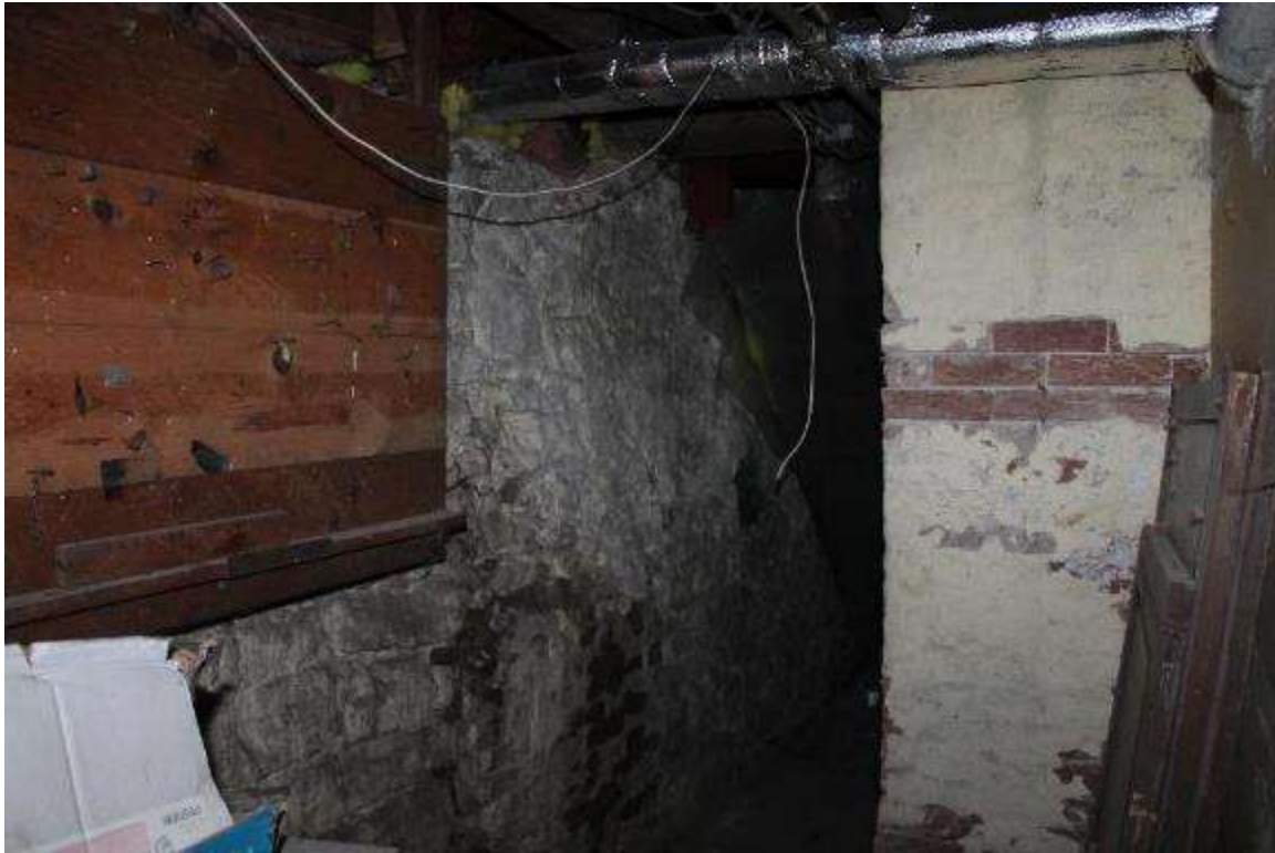
Photo 130: 12 North Franklin Street, Interior, basement
