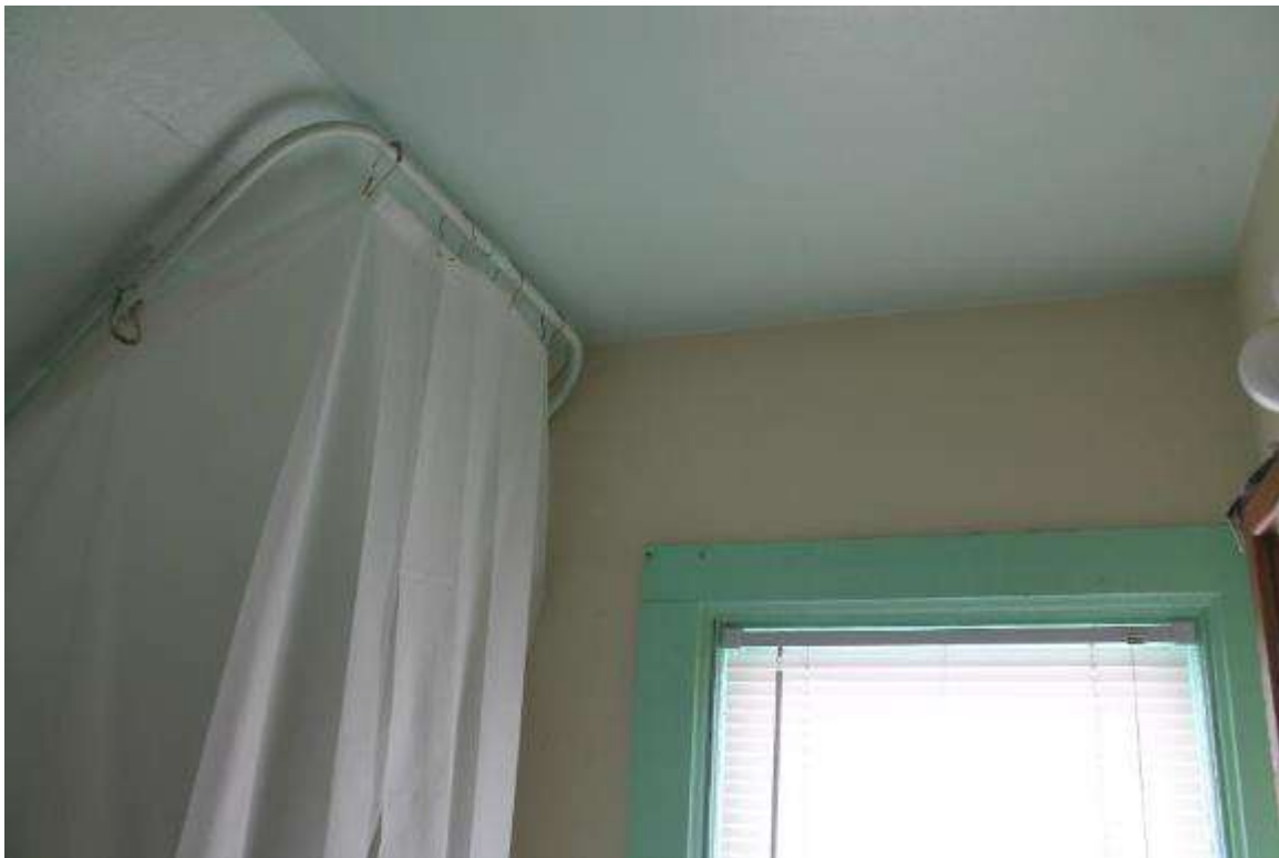
Photo 94: 8-10 North Franklin Street, Interior, third floor unit 3
