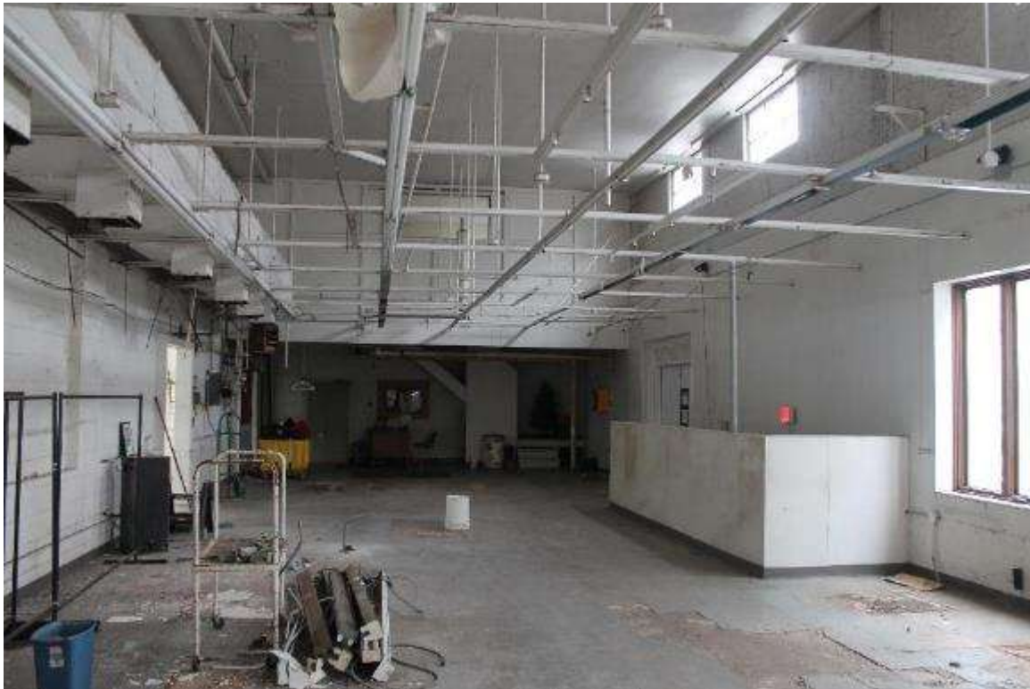
Photo 350: 412-414 East Washington Avenue, Interior, first floor processing space
