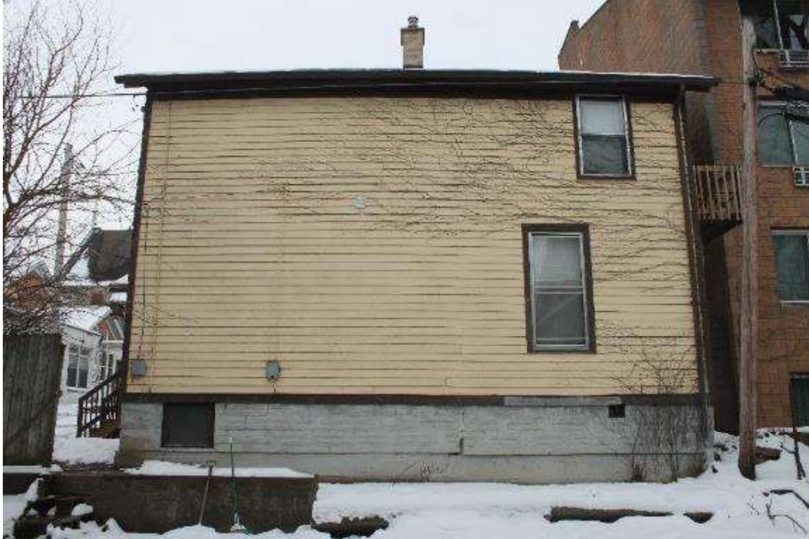
Photo 301: 410 1/2 East Washington Avenue, Exterior, facing southwest
