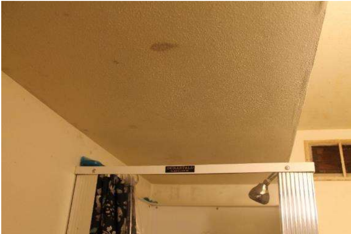
Photo 186: 402-408 East Washington Avenue, Interior, first floor unit 2
