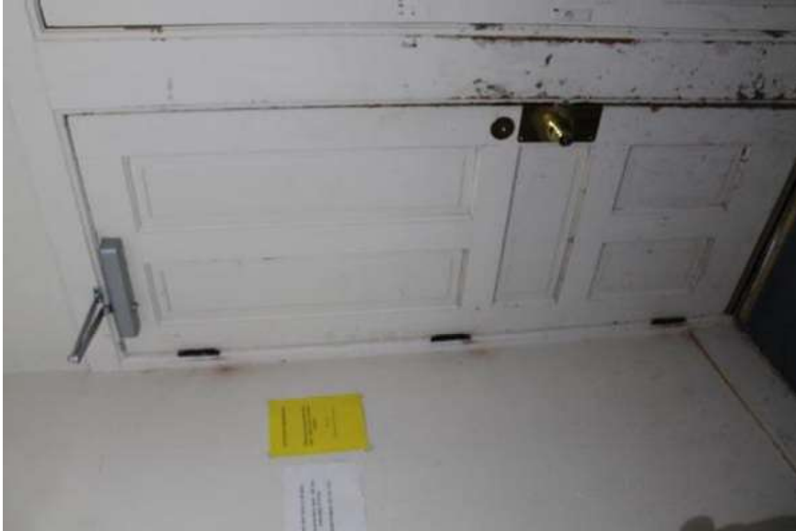
Photo 95: 8-10 North Franklin Street, Interior, third floor unit 3
