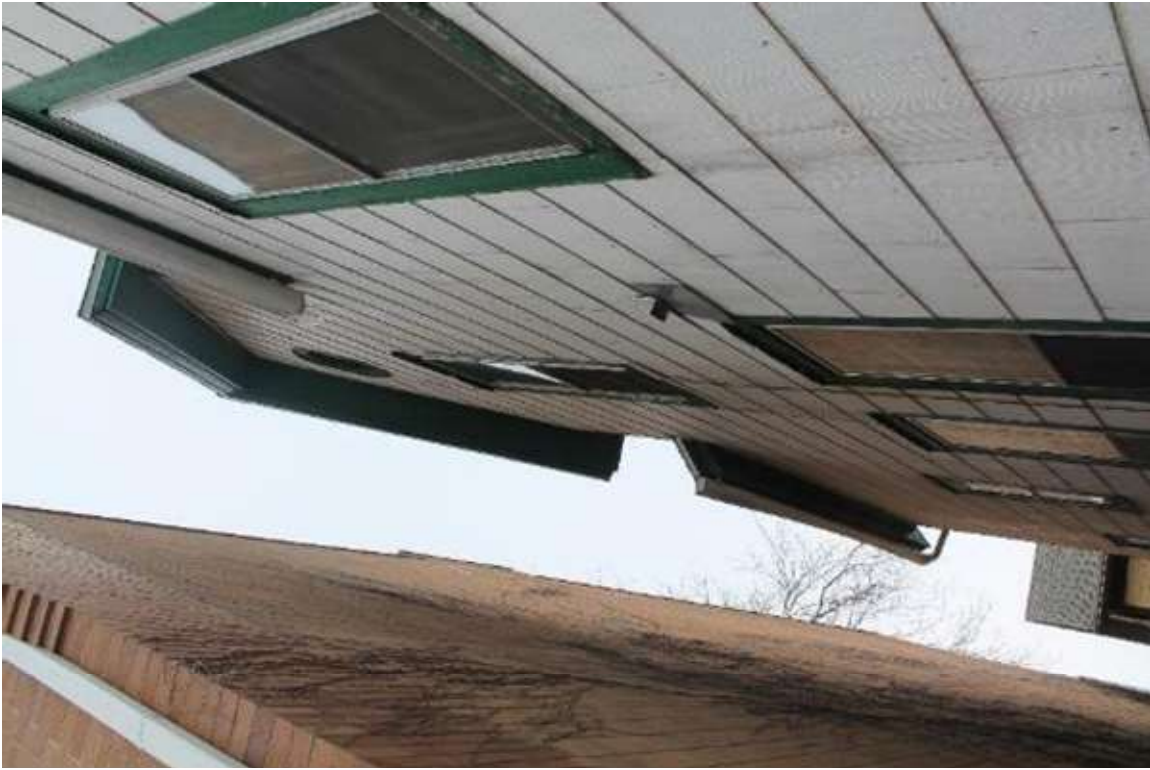
Photo 12: 9 North Hancock Street, Exterior, facing east
