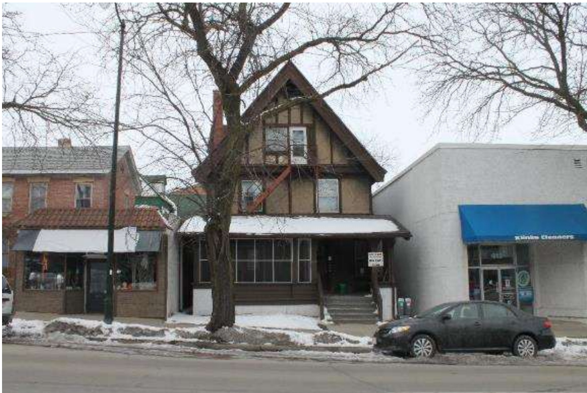
Photo 226: 410 East Washington Avenue, Exterior, facing northwest
