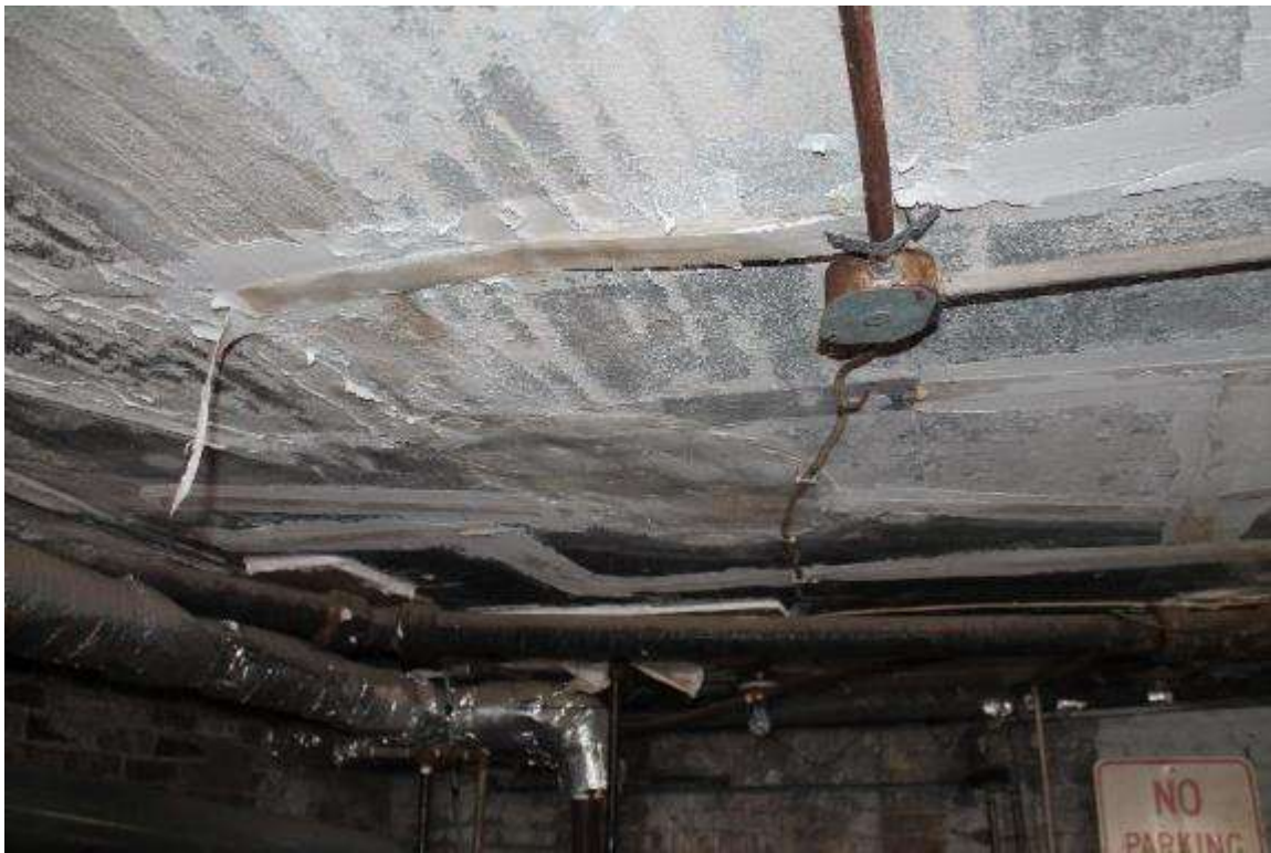
Photo 50: 9 North Hancock Street, Interior, basement
