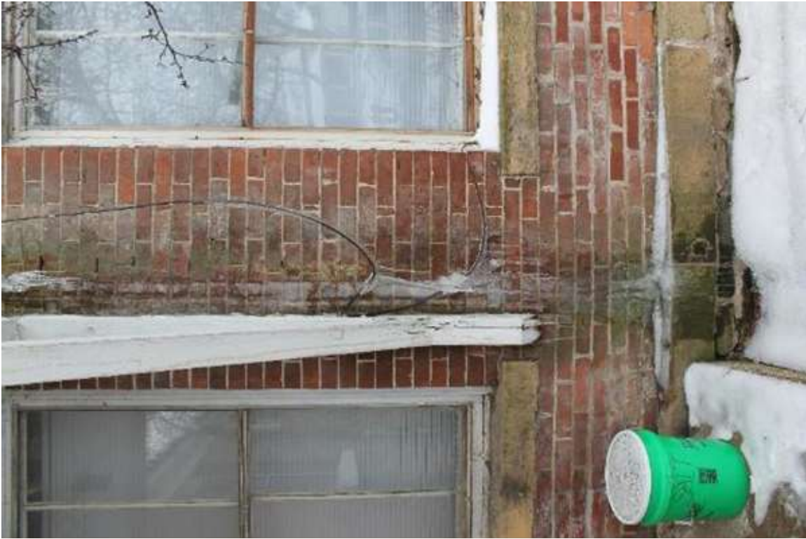
Photo 154: 402-408 East Washington Avenue, Exterior, facing northwest
