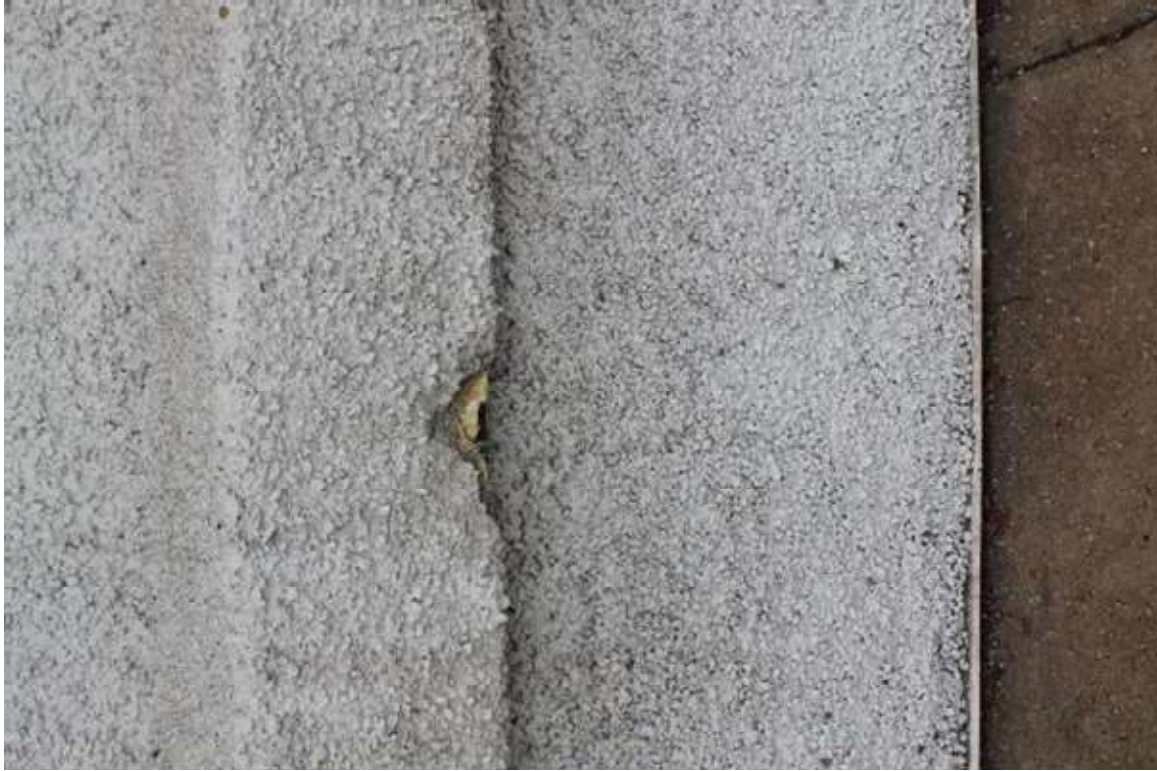
Photo 339: 412-414 East Washington Avenue, Exterior, facing northwest
