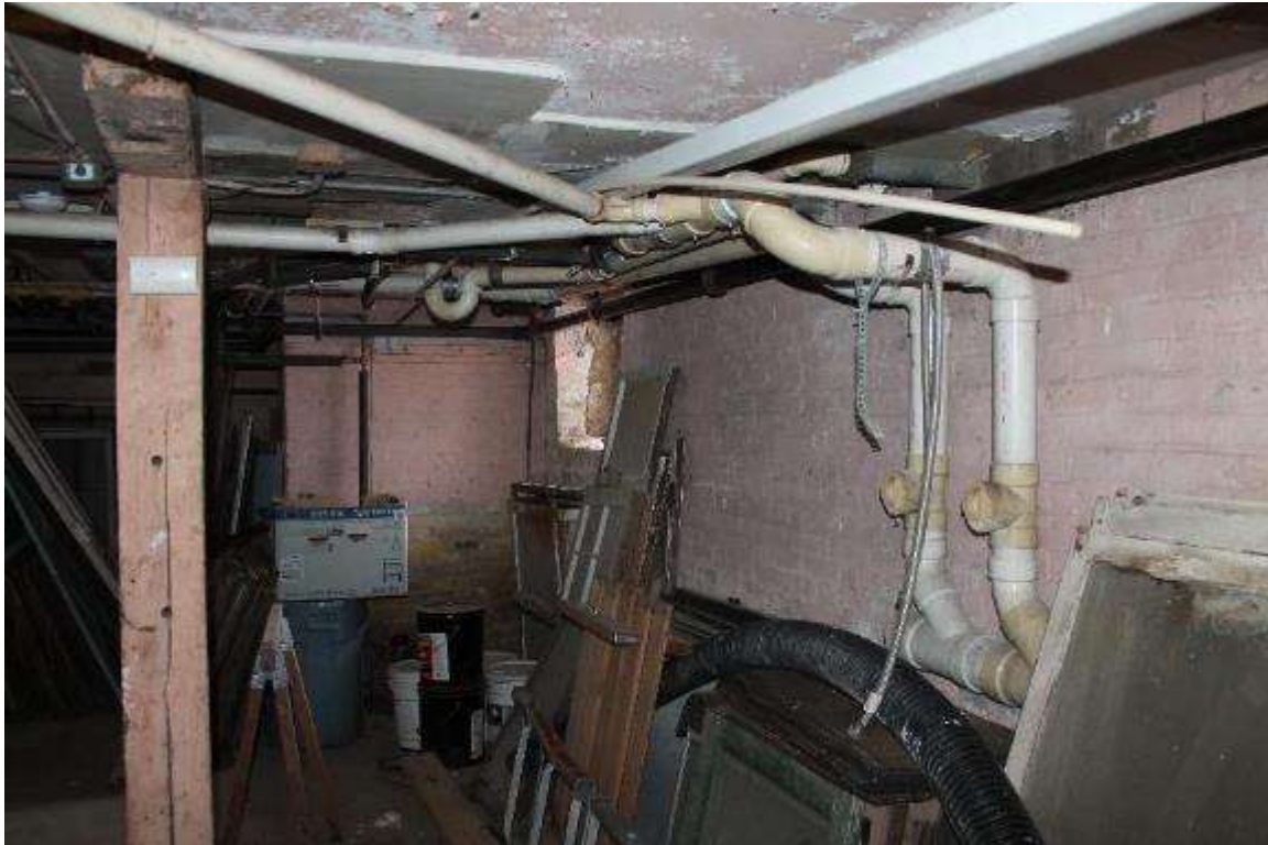
Photo 48: 9 North Hancock Street, Interior, basement
