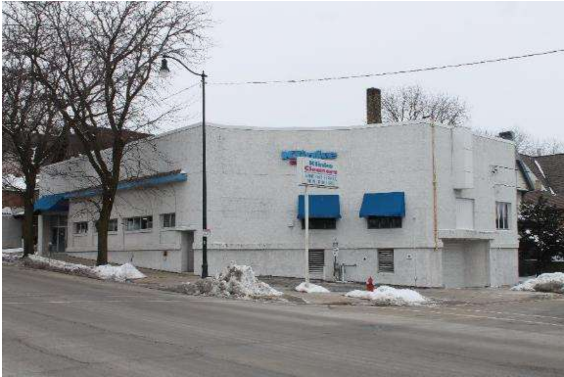
Photo 326: 412-414 East Washington Avenue, Exterior, facing west
