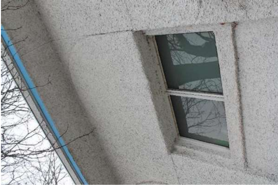
Photo 337: 412-414 East Washington Avenue, Exterior, facing northwest
