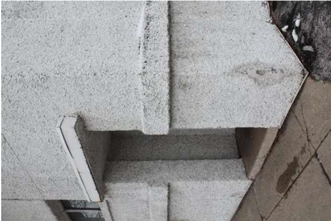
Photo 336: 412-414 East Washington Avenue, Exterior, facing west
