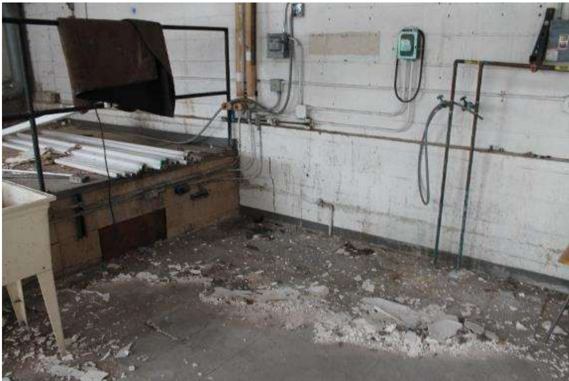
Photo 352: 412-414 East Washington Avenue, Interior, first floor processing space
