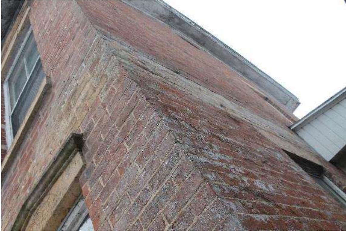
Photo 157: 402-408 East Washington Avenue, Exterior, facing west
