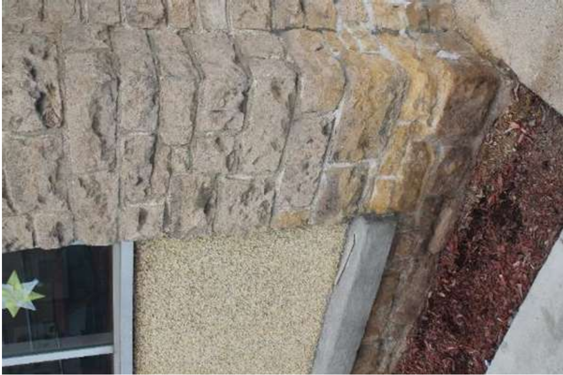
Photo 137: 402-408 East Washington Avenue, Exterior, facing northwest
