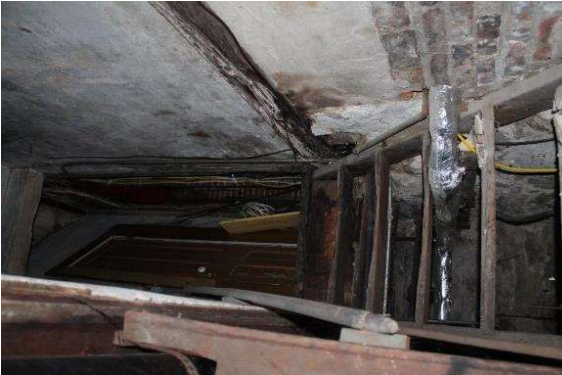
Photo 224: 402-408 East Washington Avenue, Interior, basement
