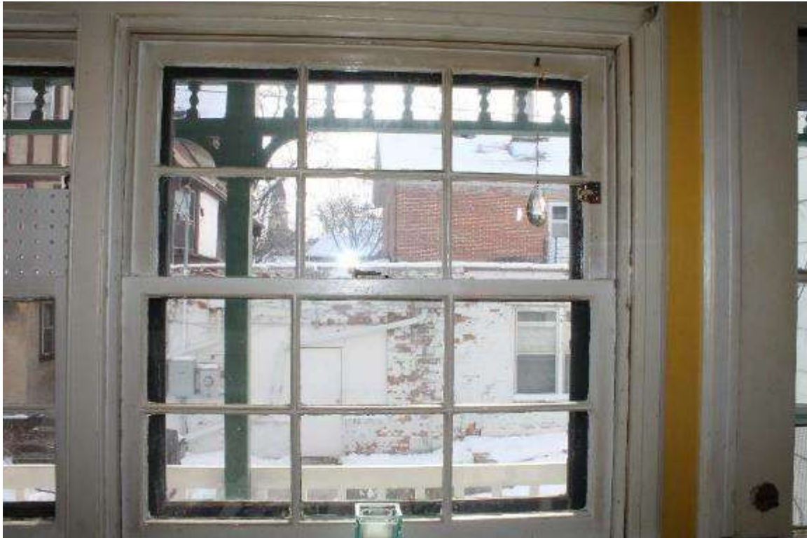
Photo 24: 9 North Hancock Street, Interior, first floor unit 1
