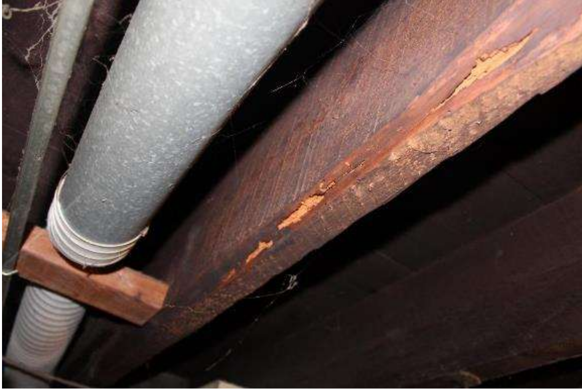
Photo 225: 402-408 East Washington Avenue, Interior, basement
