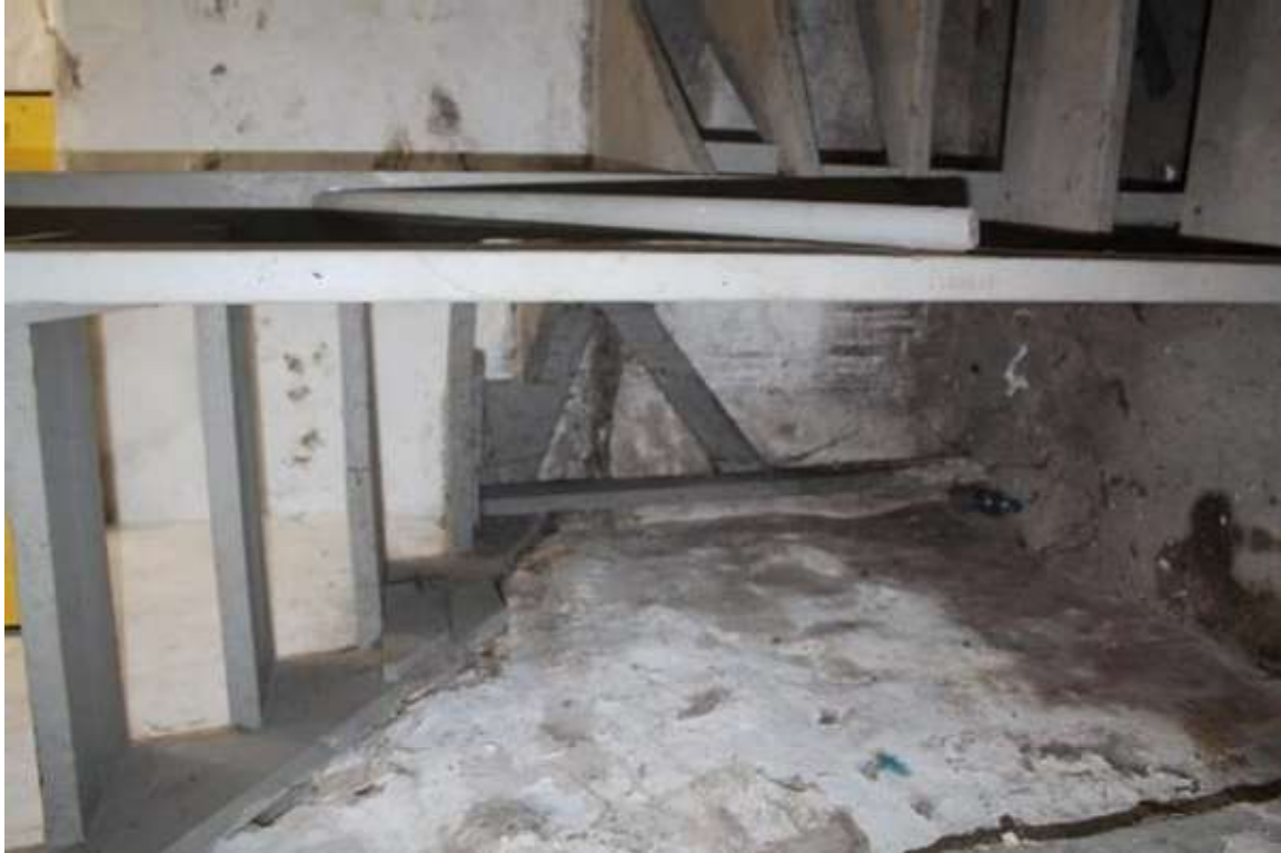
Photo 97: 8-10 North Franklin Street, Interior, basement
