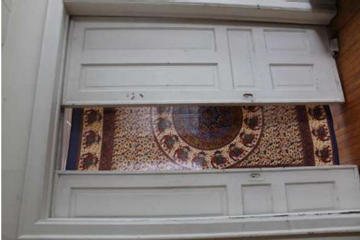
Photo 69: 8-10 North Franklin Street, Interior, first floor unit 1
