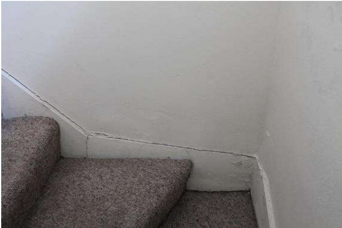
Photo 274: 410 East Washington Avenue, Interior, third floor stairwell
