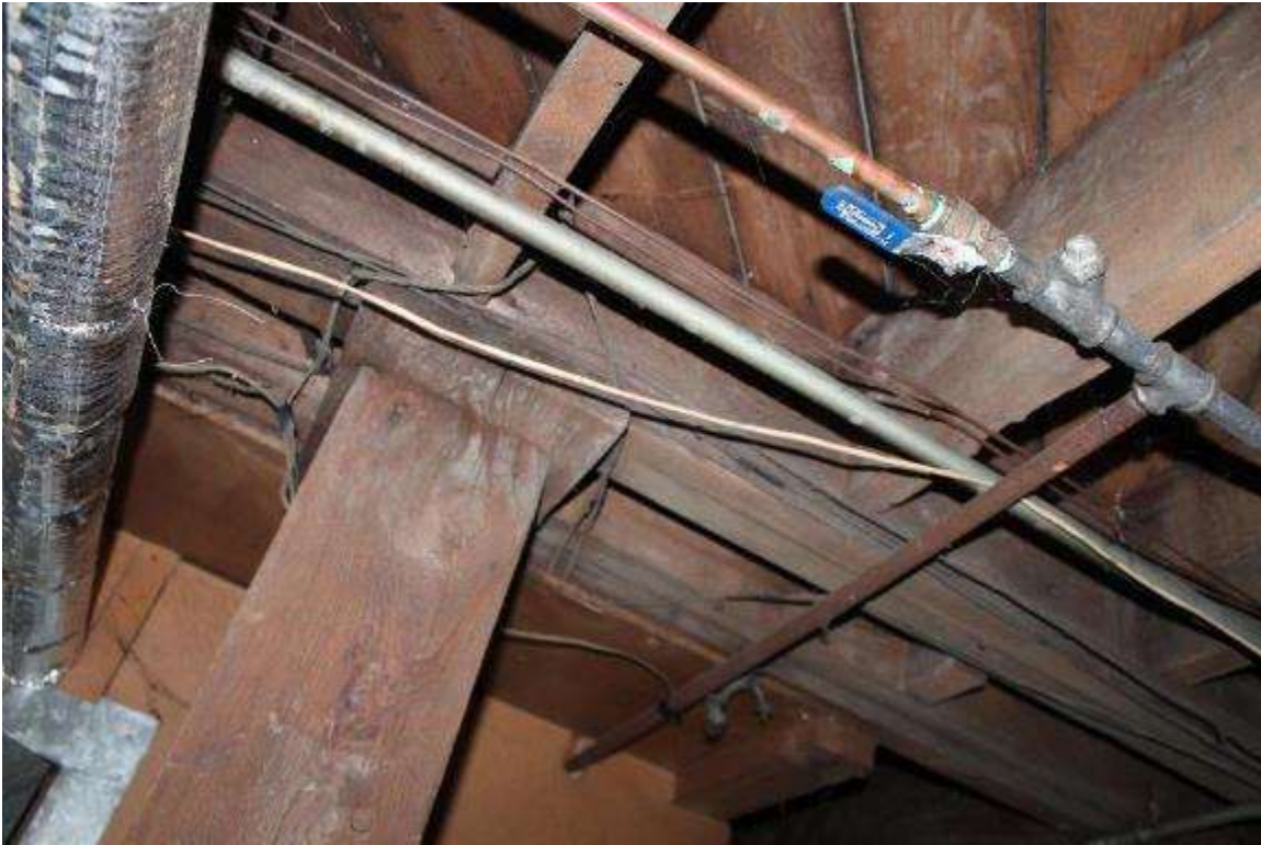
Photo 294: 410 East Washington Avenue, Interior, basement
