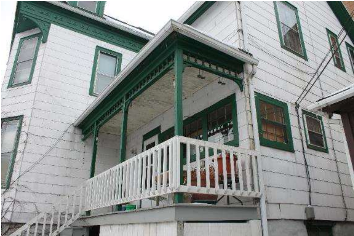
Photo 6: 9 North Hancock Street, Exterior, facing west
