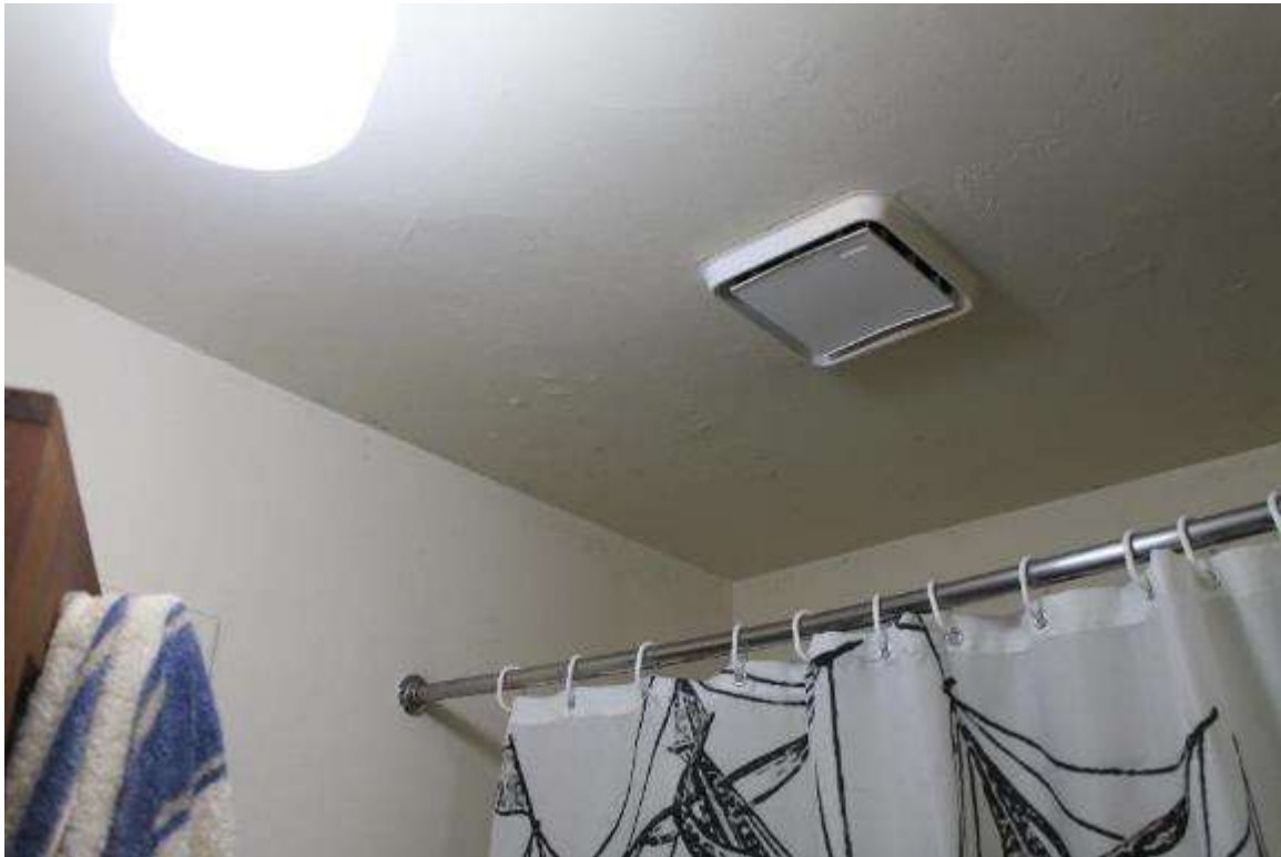
Photo 194: 402-408 East Washington Avenue, Interior, first floor unit 1
