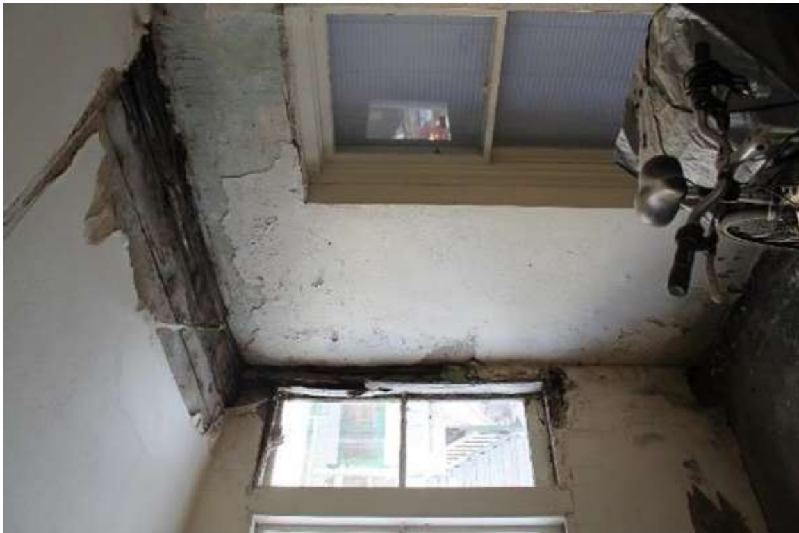
Photo 178: 402-408 East Washington Avenue, Interior, first floor unit 2
