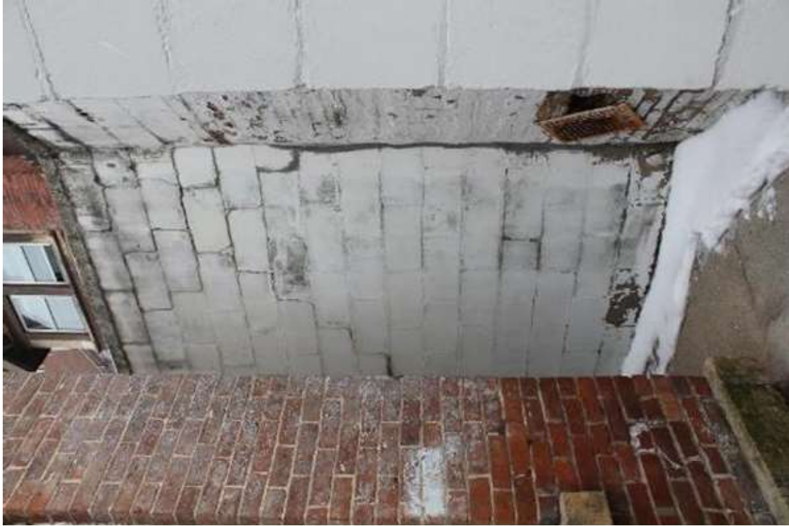
Photo 159: 402-408 East Washington Avenue, Exterior, facing northeast
