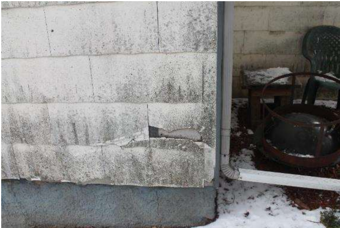
Photo 62: 8-10 North Franklin Street, Exterior, facing southeast
