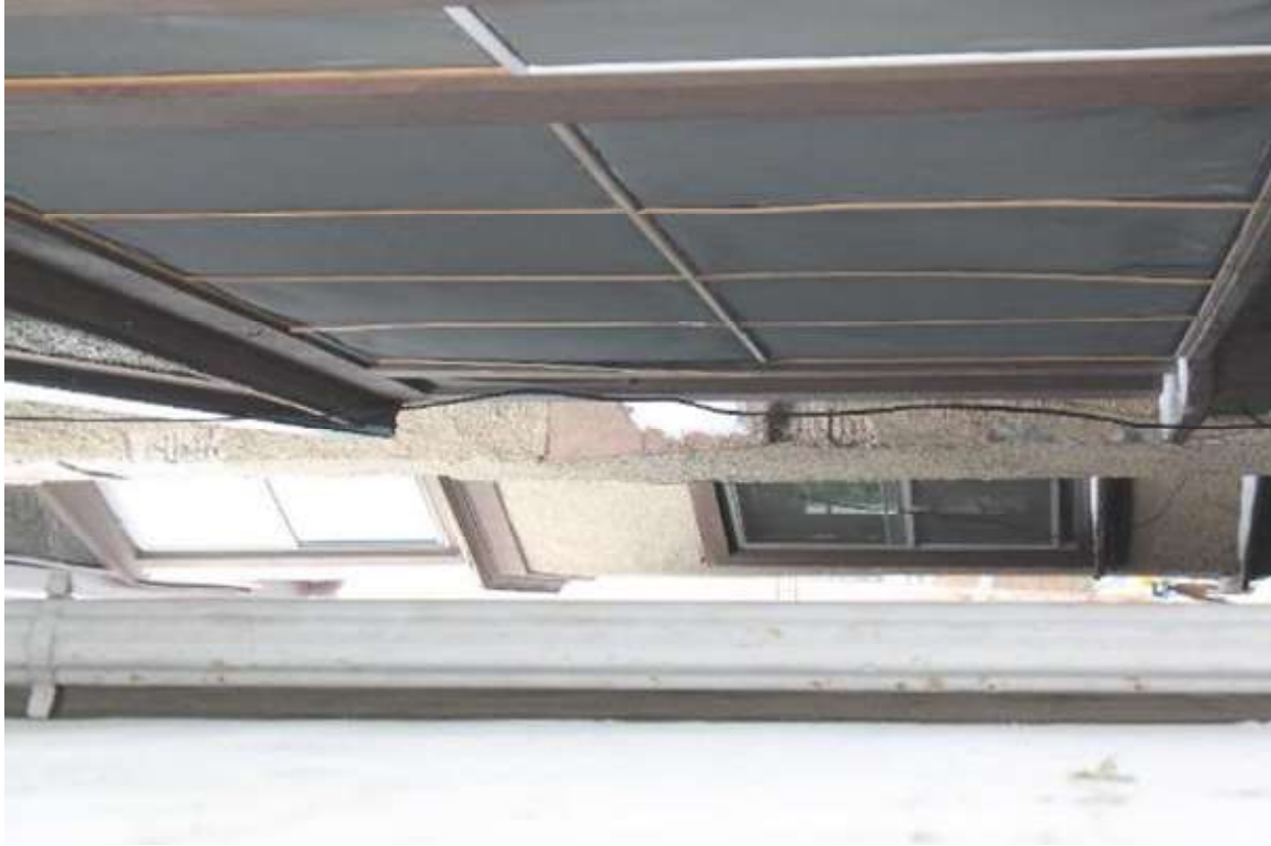
Photo 237: 410 East Washington Avenue, Exterior, facing northwest
