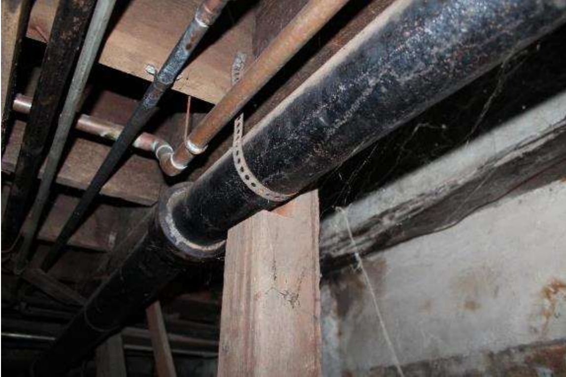
Photo 223: 402-408 East Washington Avenue, Interior, basement
