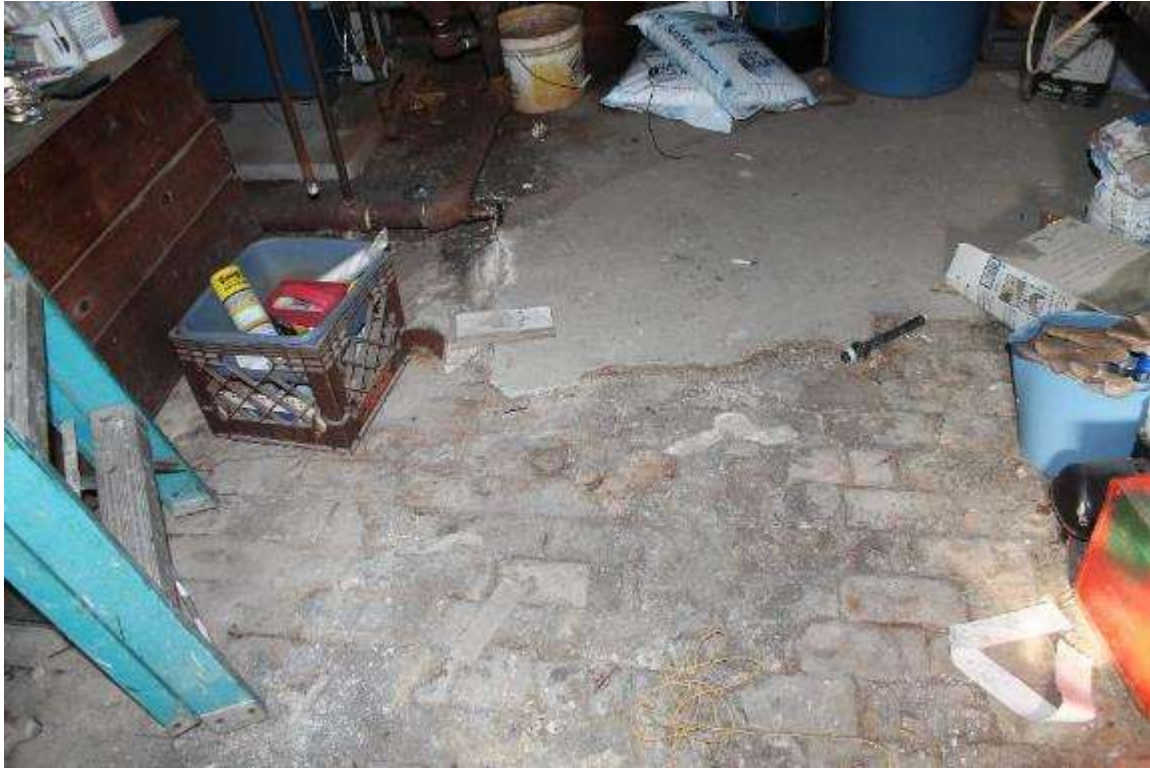
Photo 49: 9 North Hancock Street, Interior, basement
