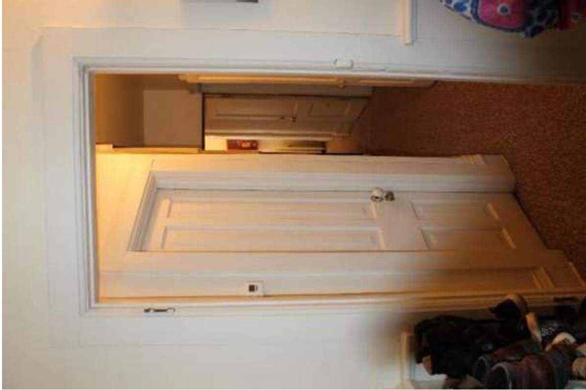
Photo 187: 402-408 East Washington Avenue, Interior, first floor unit 2
