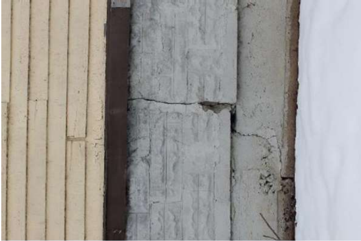
Photo 303: 410 1/2 East Washington Avenue, Exterior, facing southwest
