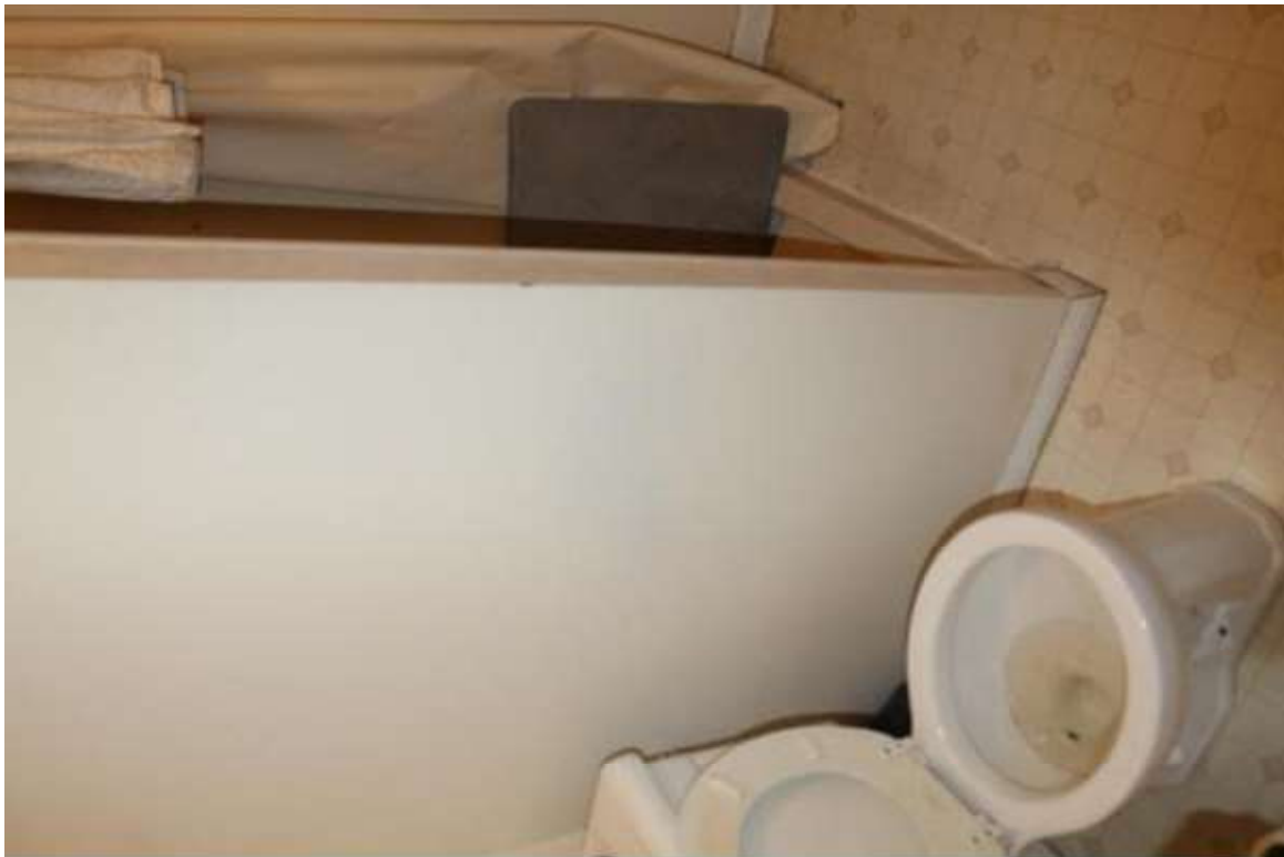
Photo 308: 410 1/2 East Washington Avenue, Interior, first floor unit 1
