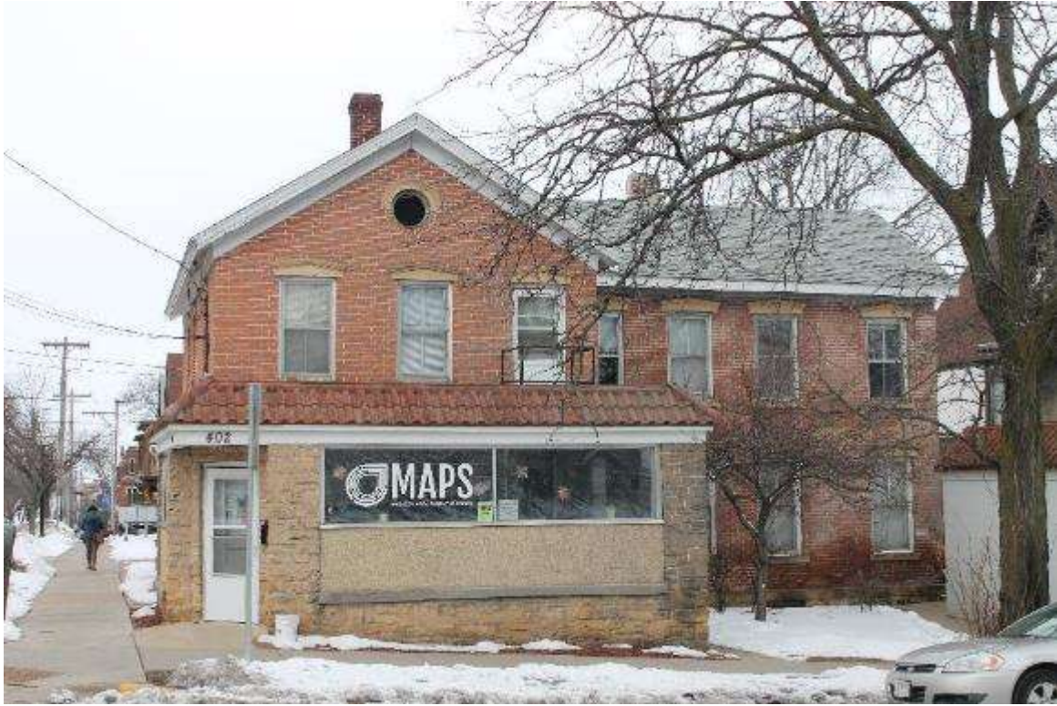
Photo 131: 402-408 East Washington Avenue, Exterior, facing northwest
