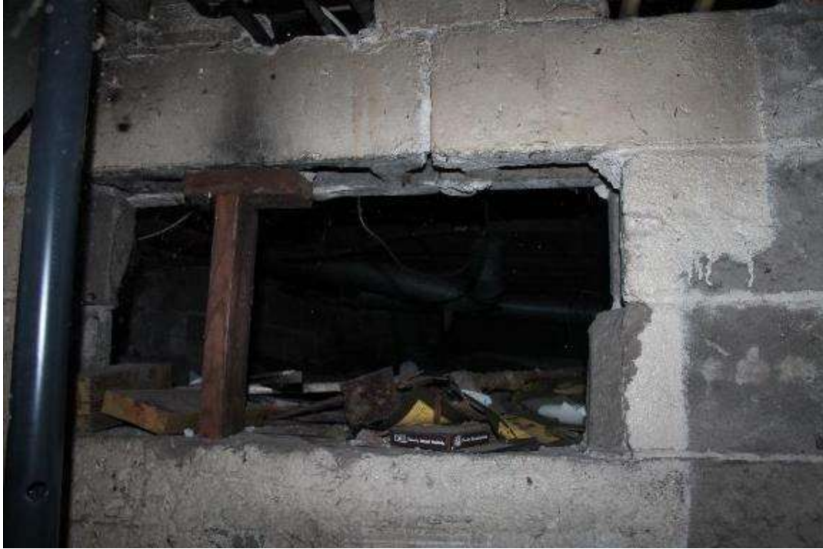
Photo 325: 410 1/2 East Washington Avenue, Interior, basement
