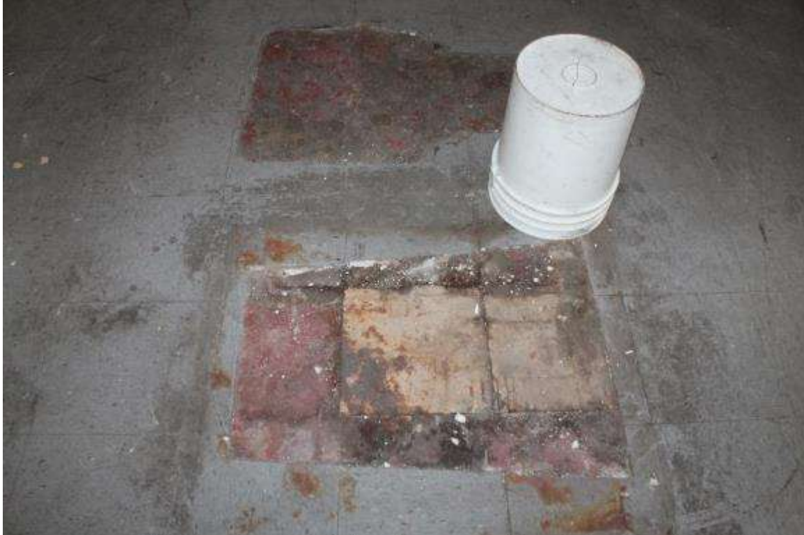
Photo 353: 412-414 East Washington Avenue, Interior, first floor processing space
