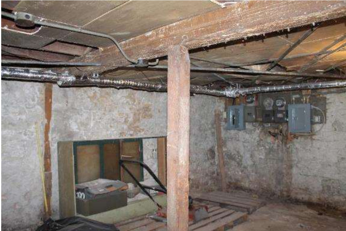
Photo 221: 402-408 East Washington Avenue, Interior, basement
