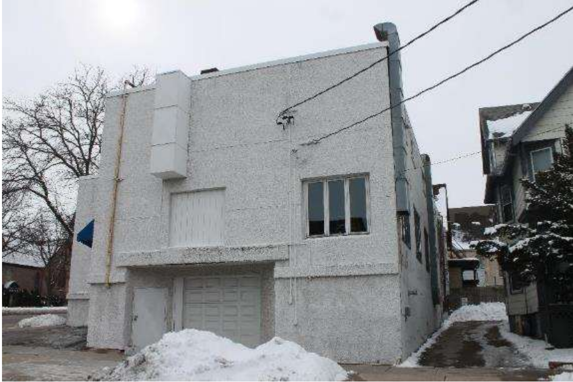
Photo 329: 412-414 East Washington Avenue, Exterior, facing southwest
