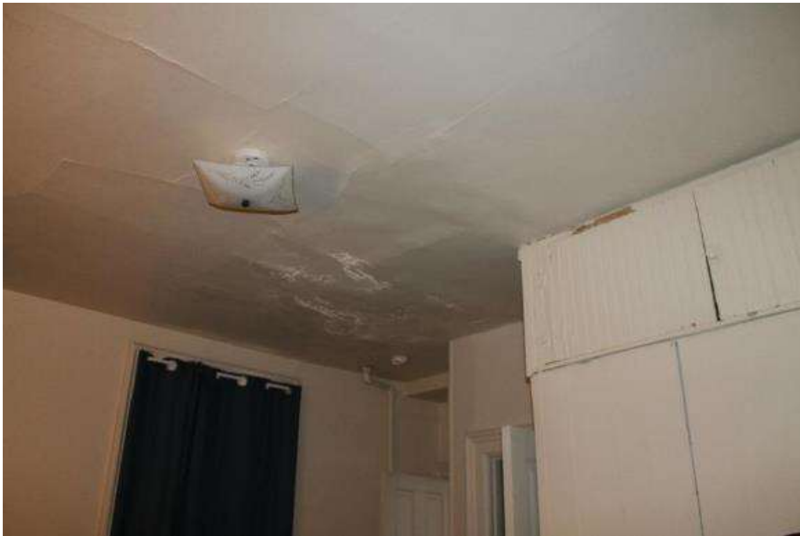
Photo 184: 402-408 East Washington Avenue, Interior, first floor unit 2
