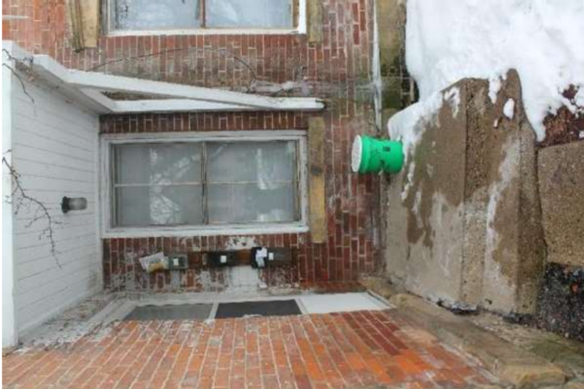
Photo 151: 402-408 East Washington Avenue, Exterior, facing northwest
