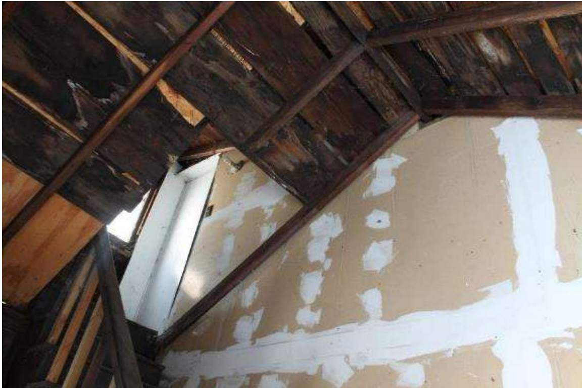
Photo 128: 12 North Franklin Street, Interior, rear stairs
