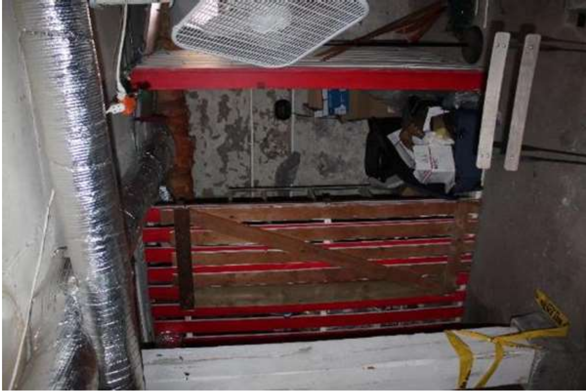
Photo 99: 8-10 North Franklin Street, Interior, basement
