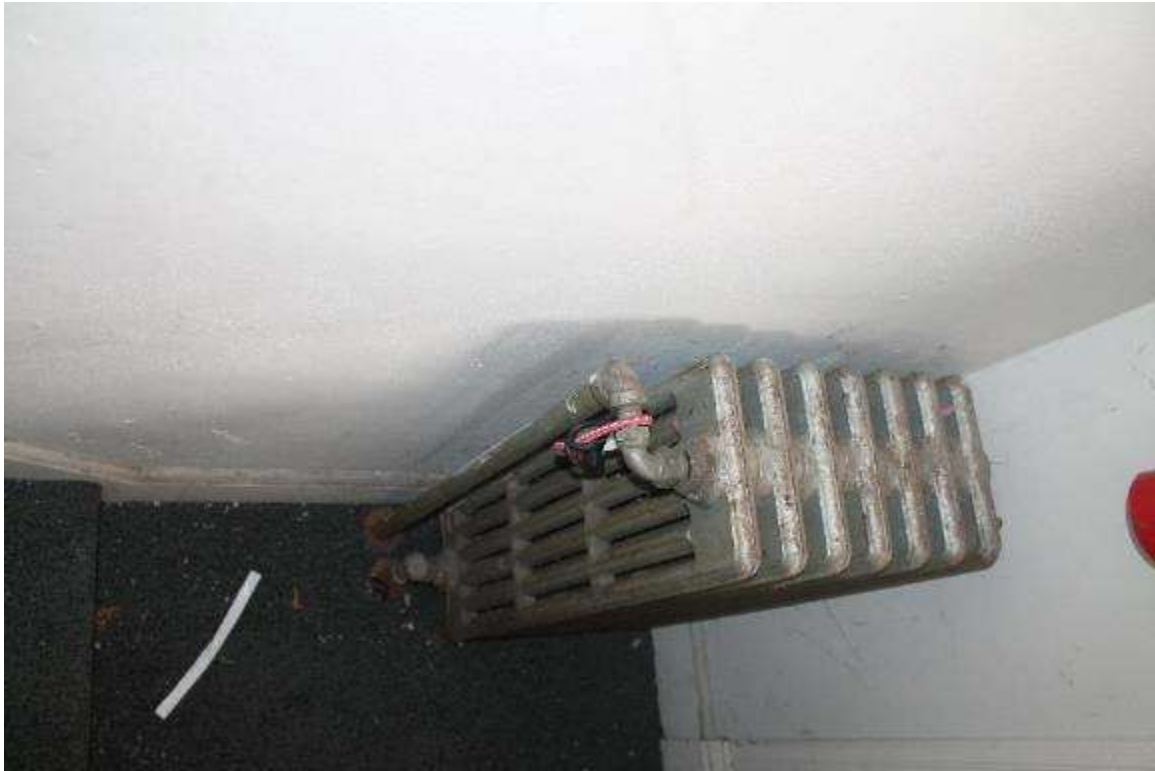
Photo 112: 12 North Franklin Street, Interior, first floor entryway
