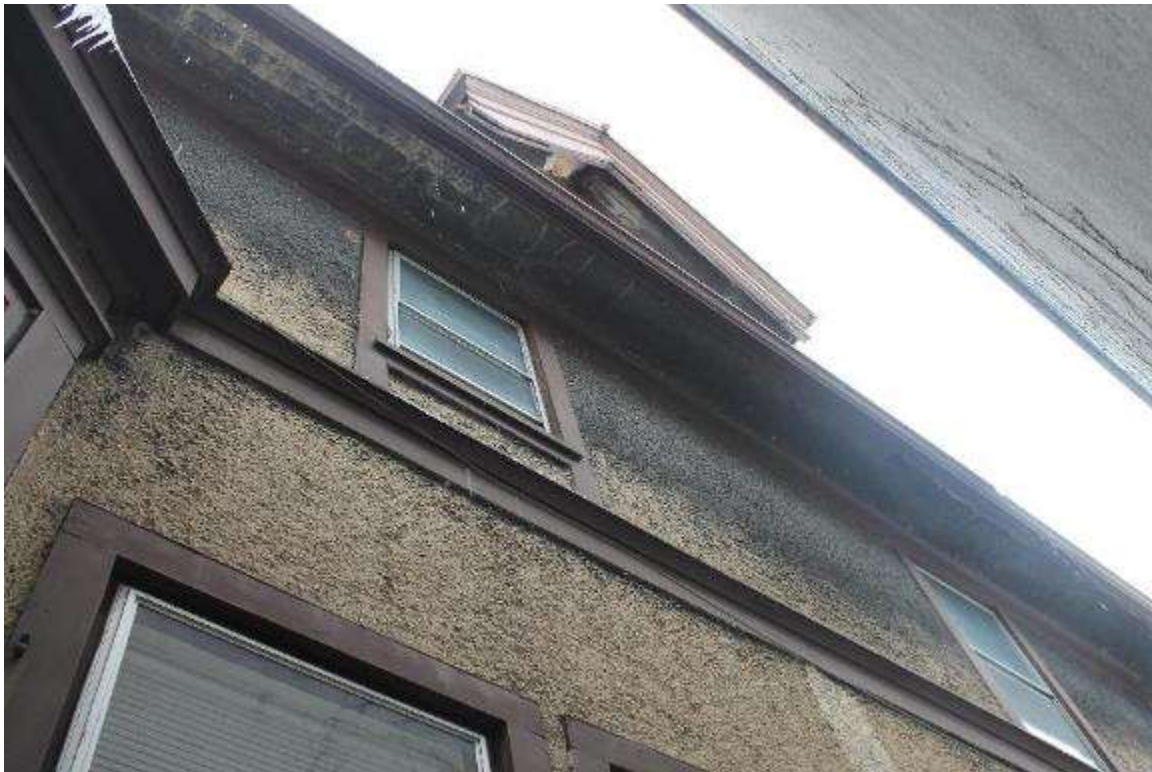
Photo 240: 410 East Washington Avenue, Exterior, facing west
