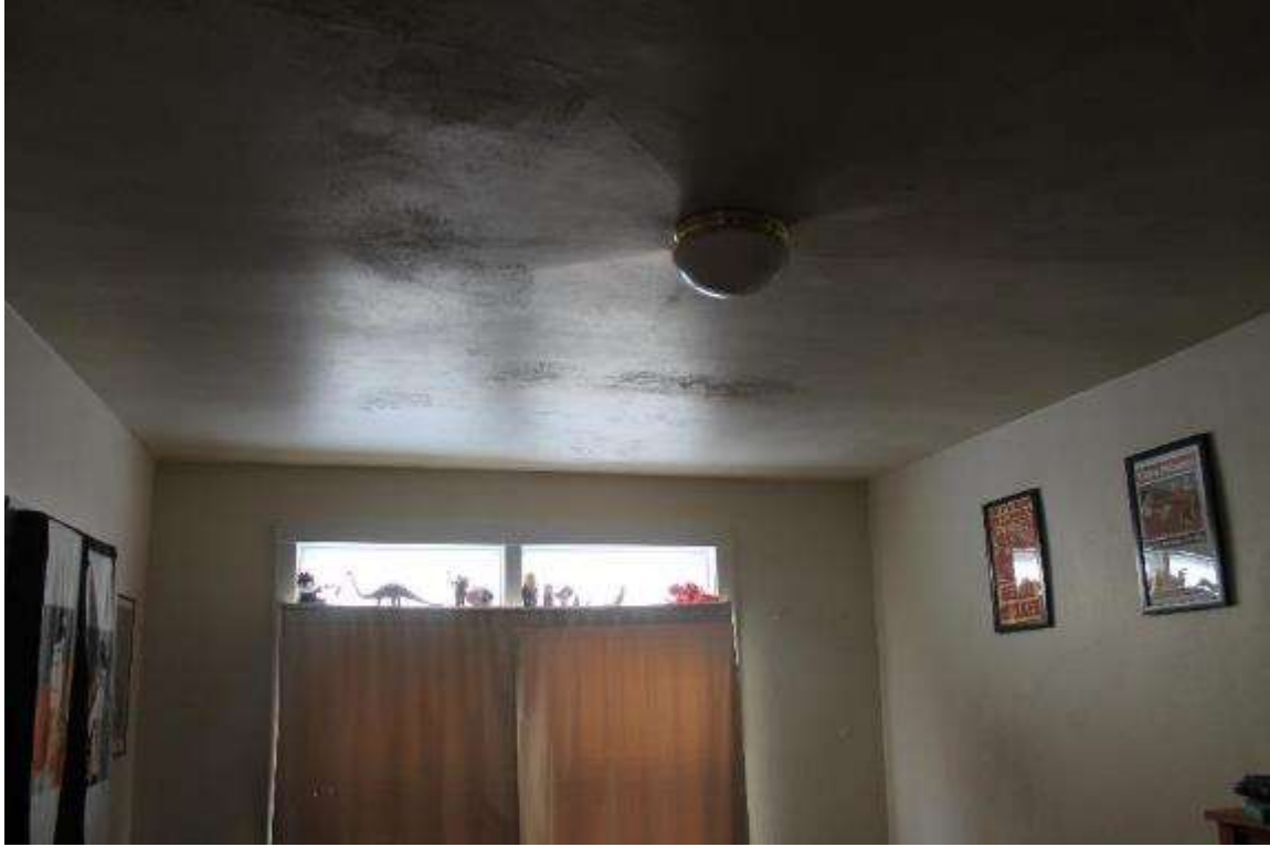
Photo 191: 402-408 East Washington Avenue, Interior, first floor unit 1
