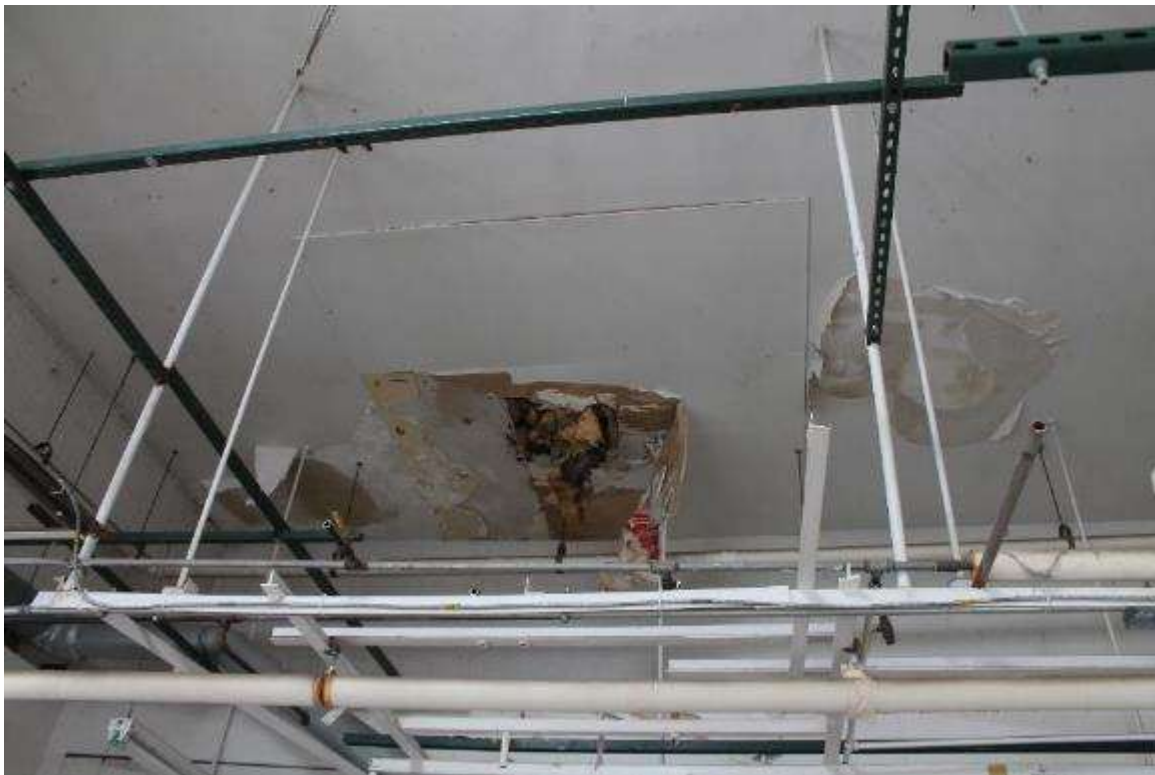
Photo 354: 412-414 East Washington Avenue, Interior, first floor processing space
