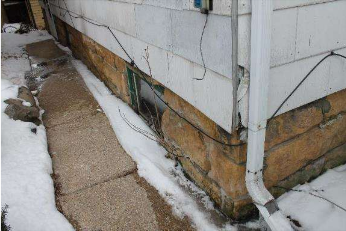
Photo 11: 9 North Hancock Street, Exterior, facing east
