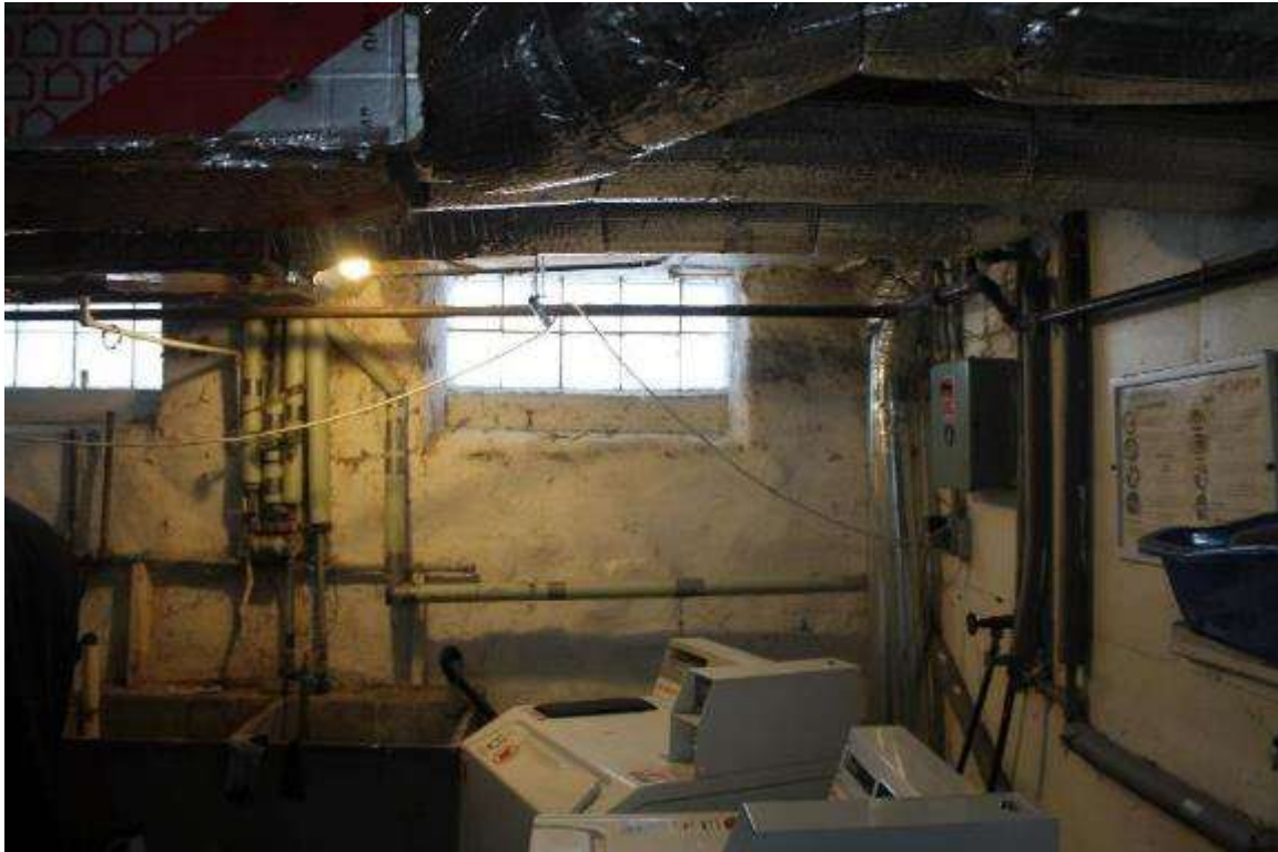
Photo 98: 8-10 North Franklin Street, Interior, basement
