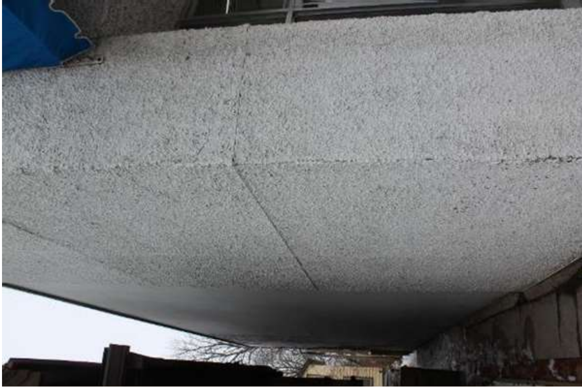
Photo 341: 412-414 East Washington Avenue, Exterior, facing northwest
