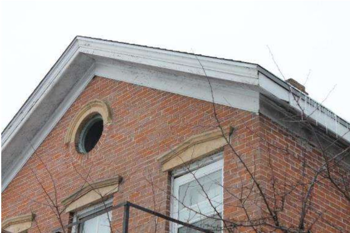
Photo 140: 402-408 East Washington Avenue, Exterior, facing northwest
