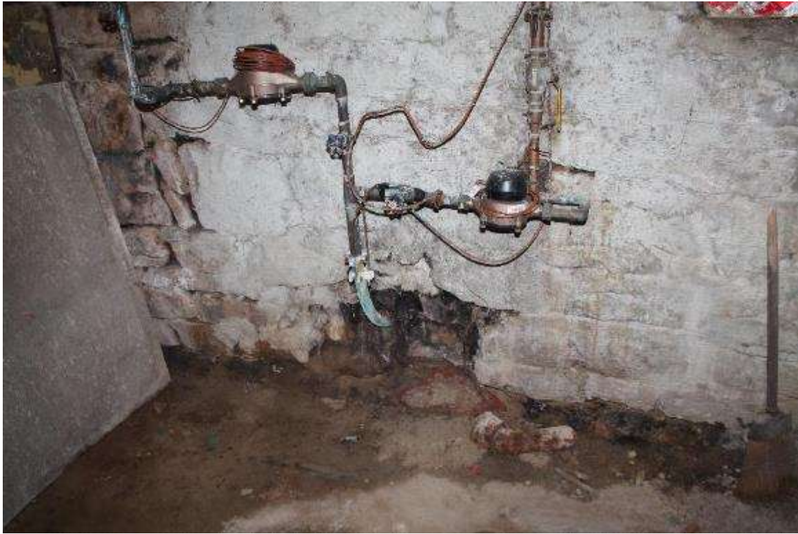
Photo 222: 402-408 East Washington Avenue, Interior, basement
