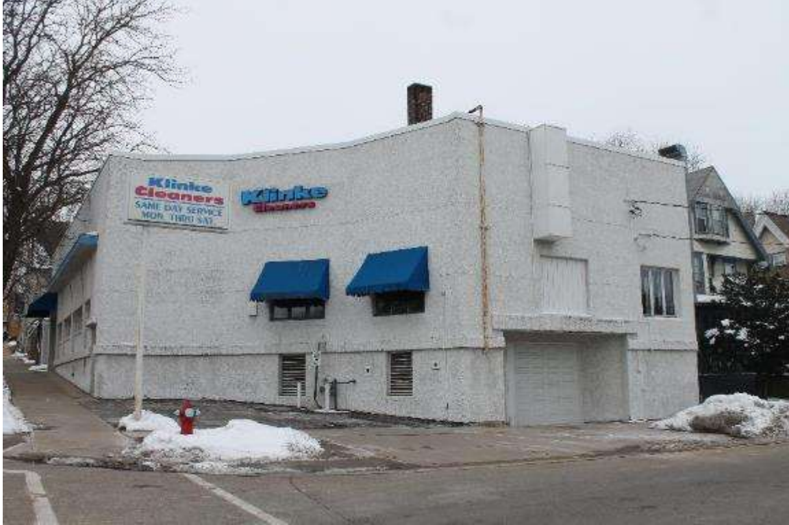
Photo 327: 412-414 East Washington Avenue, Exterior, facing west
