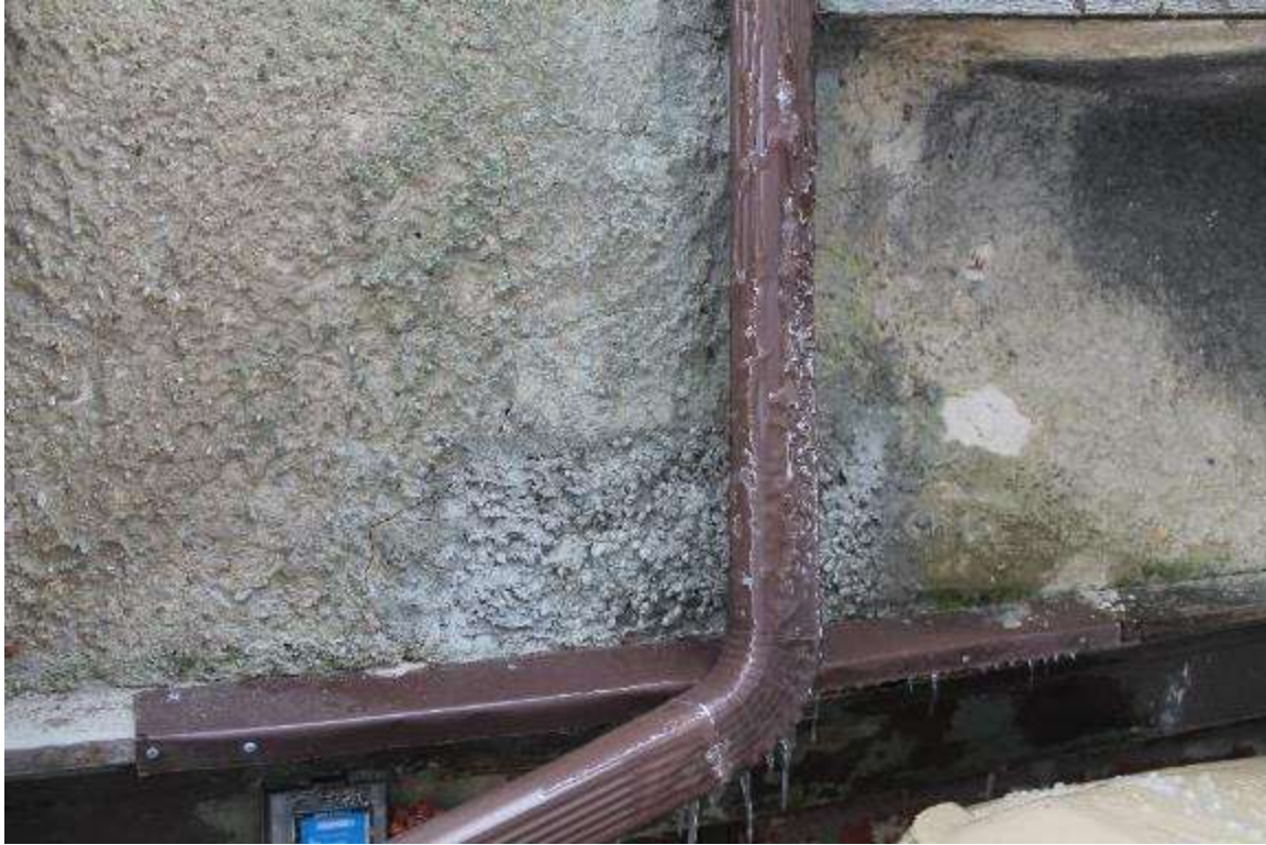
Photo 239: 410 East Washington Avenue, Exterior, facing west
