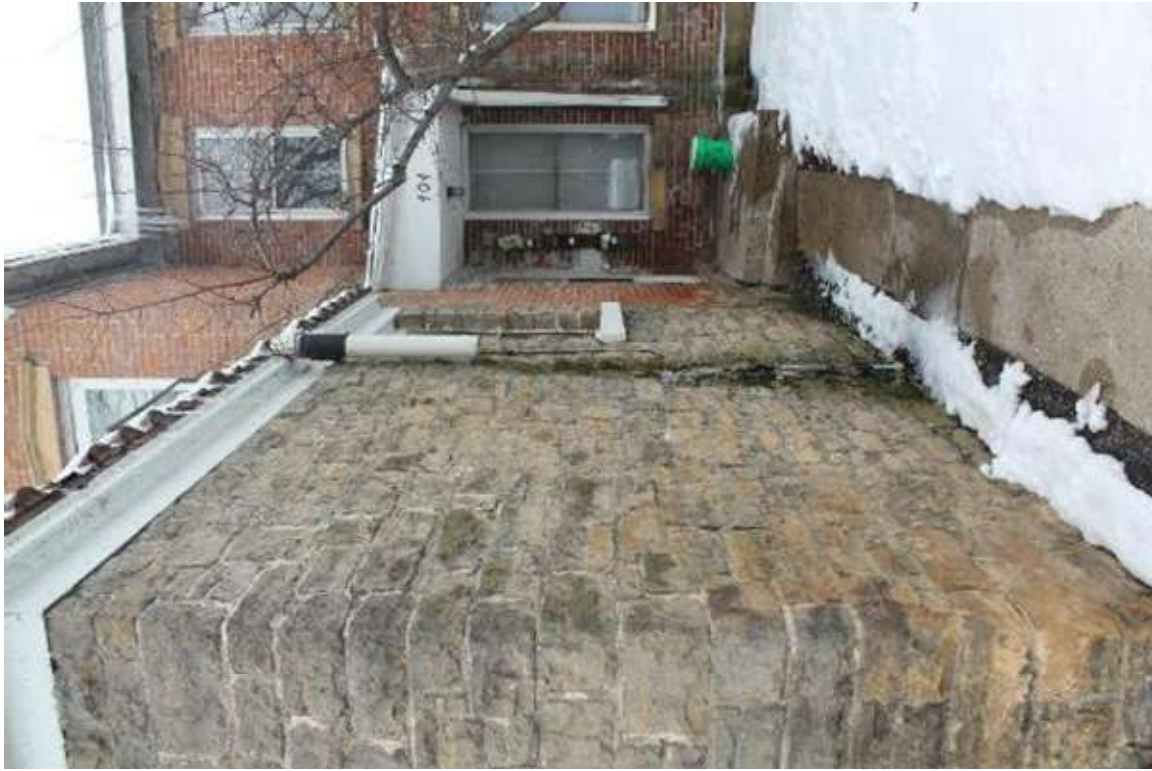
Photo 150: 402-408 East Washington Avenue, Exterior, facing northwest
