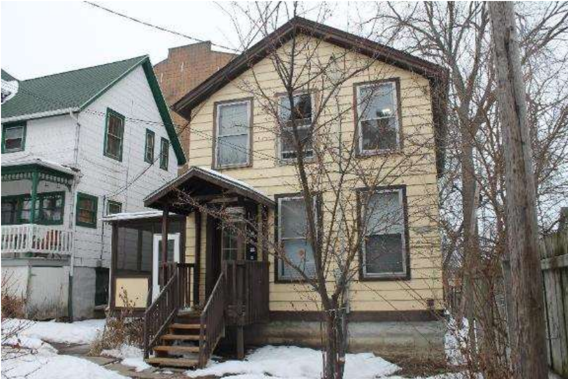
Photo 296: 410 1/2 East Washington Avenue, Exterior, facing northwest
