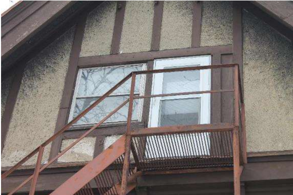
Photo 236: 410 East Washington Avenue, Exterior, facing northwest
