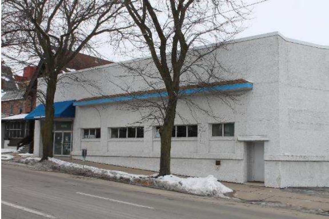
Photo 335: 412-414 East Washington Avenue, Exterior, facing west
