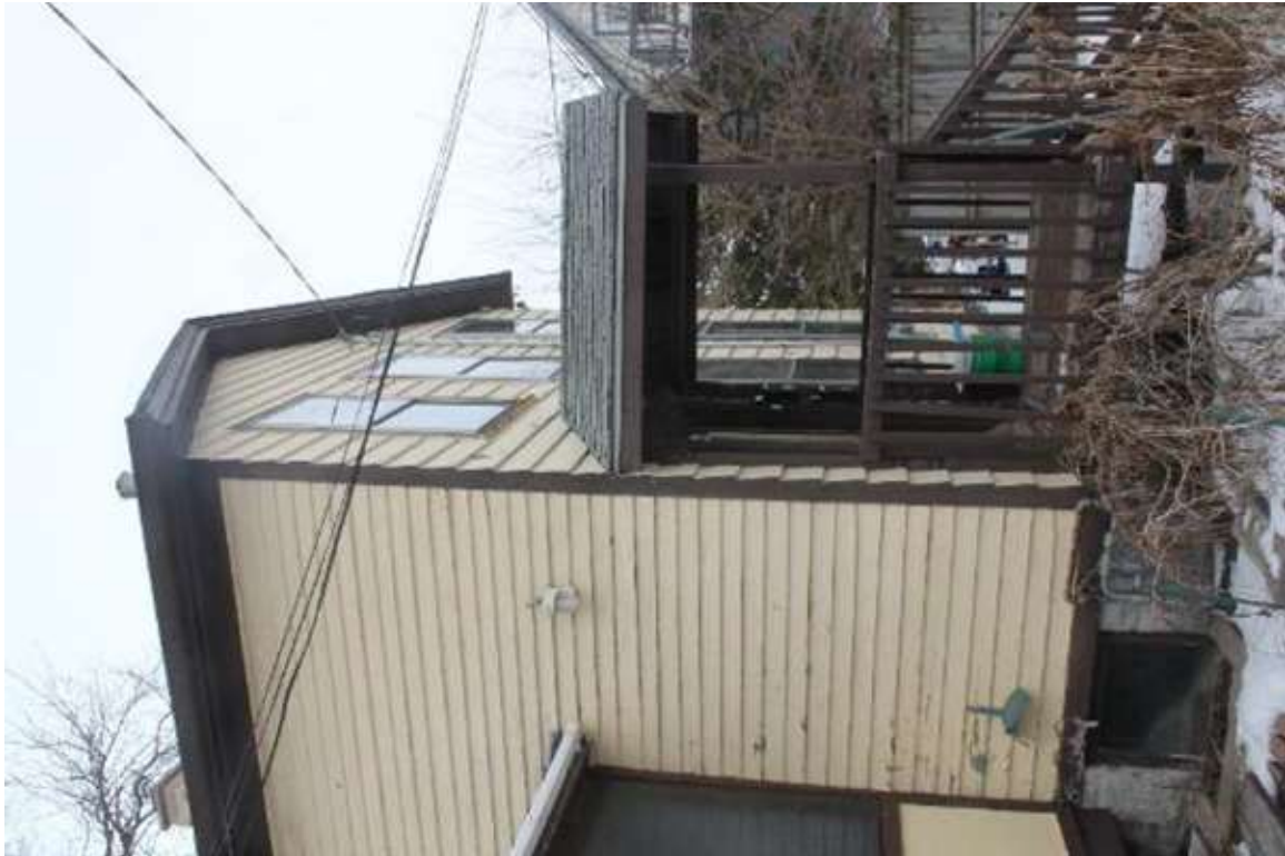
Photo 300: 410 1/2 East Washington Avenue, Exterior, facing northeast
