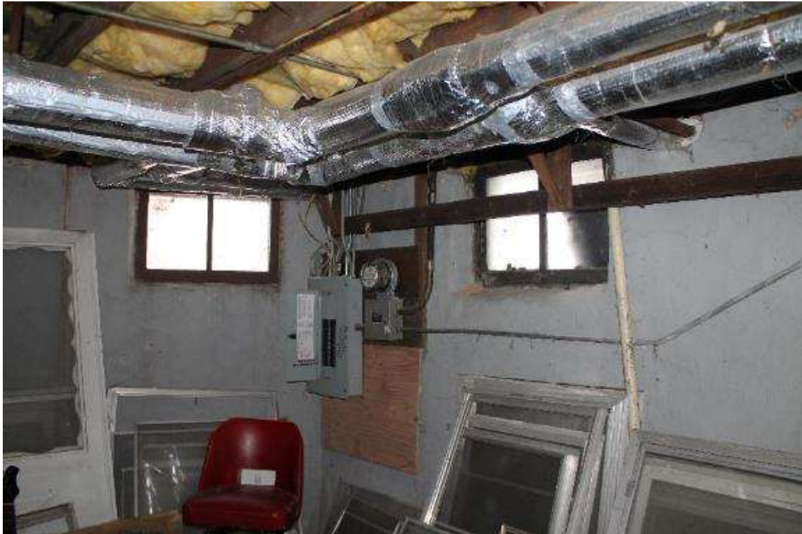
Photo 290: 410 East Washington Avenue, Interior, basement
