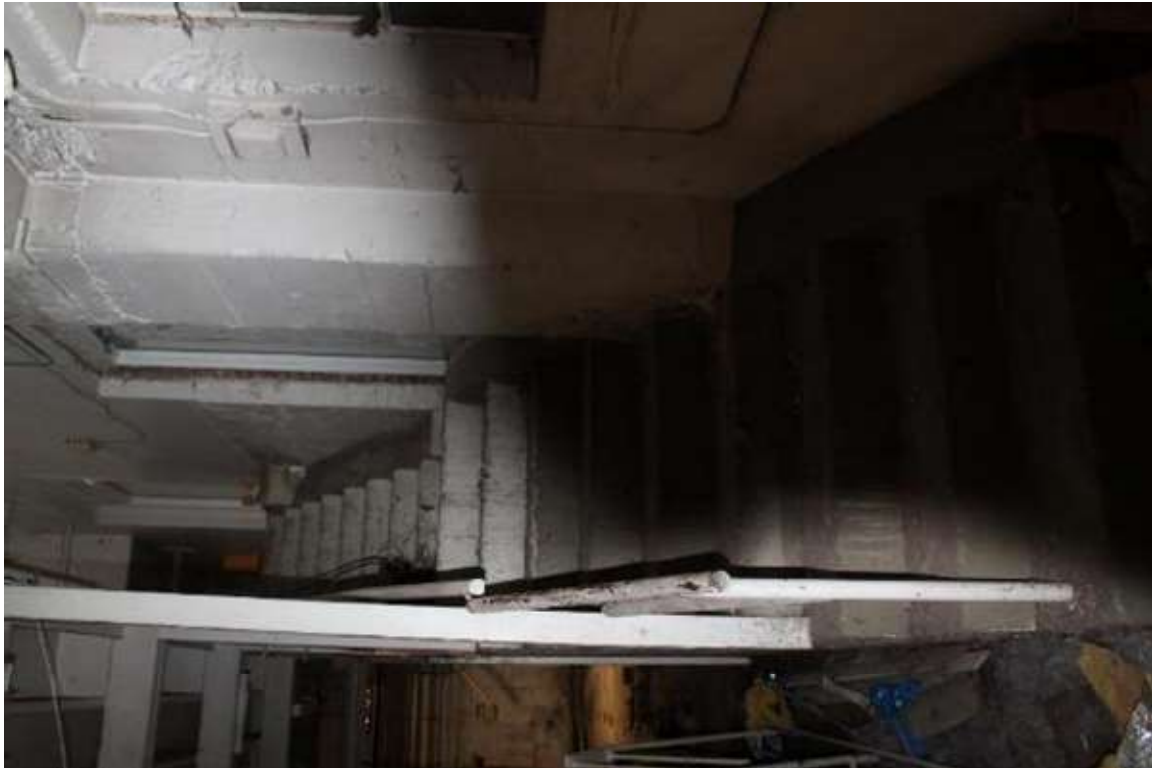
Photo 364: 412-414 East Washington Avenue, Interior, lower level storage space
