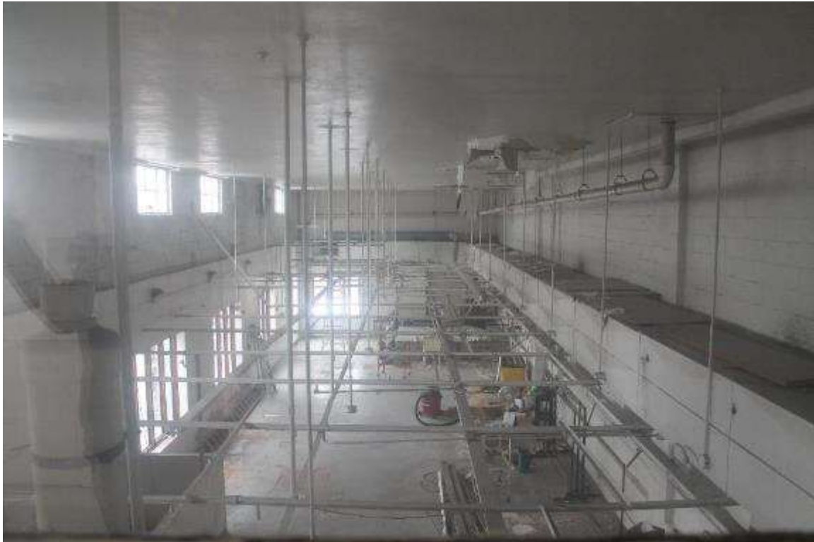
Photo 356: 412-414 East Washington Avenue, Interior, first floor mezzanine space
