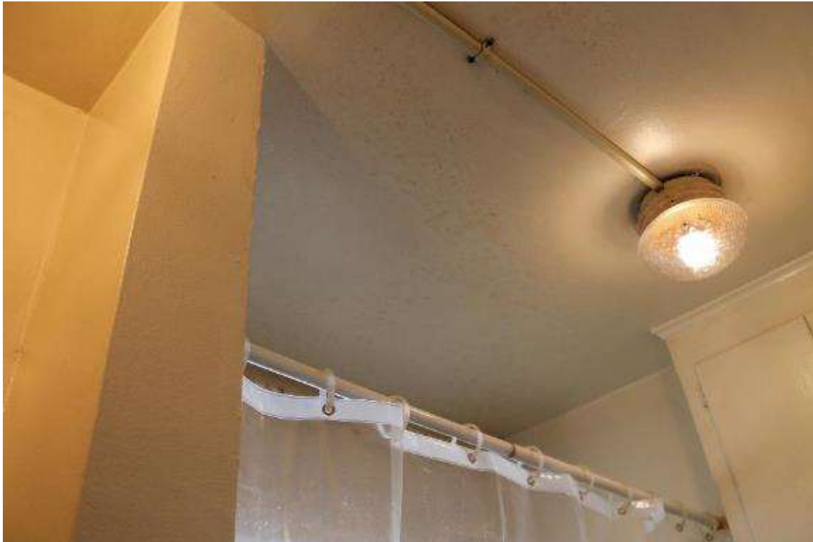
Photo 26: 9 North Hancock Street, Interior, first floor unit 1
