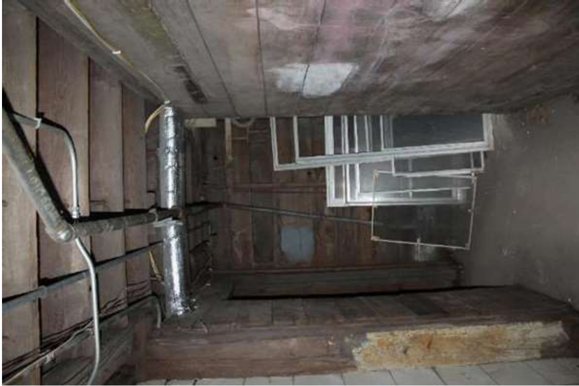
Photo 291: 410 East Washington Avenue, Interior, basement
