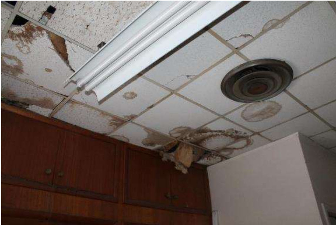
Photo 360: 412-414 East Washington Avenue, Interior, first floor mezzanine space
