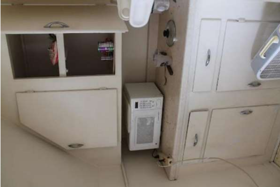
Photo 278: 410 East Washington Avenue, Interior, third floor unit 7
