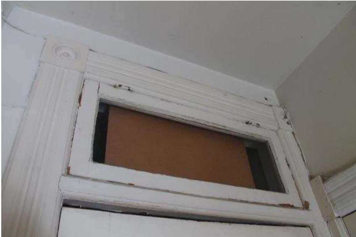
Photo 34: 9 North Hancock Street, Interior, second floor hallway
