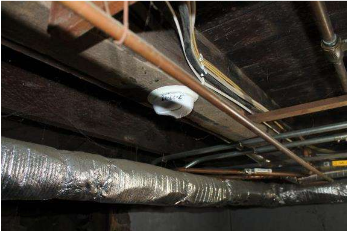
Photo 218: 402-408 East Washington Avenue, Interior, basement
