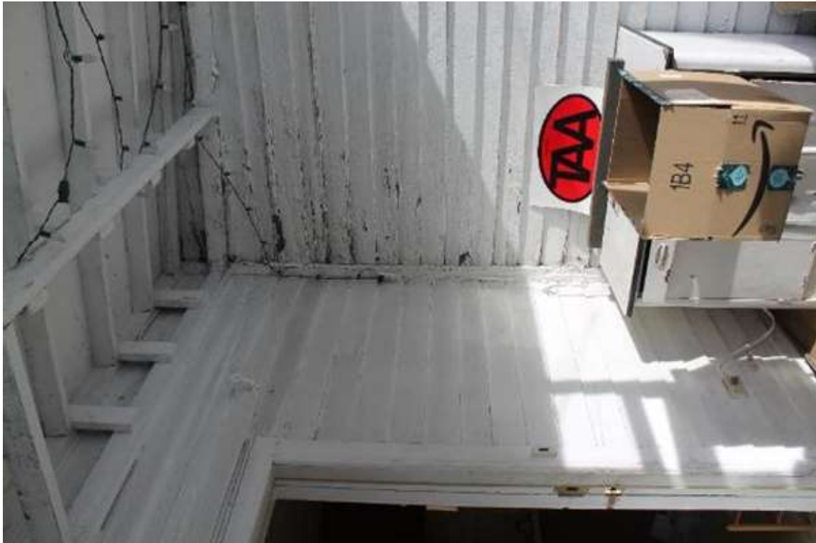
Photo 306: 410 1/2 East Washington Avenue, Exterior, facing northeast
