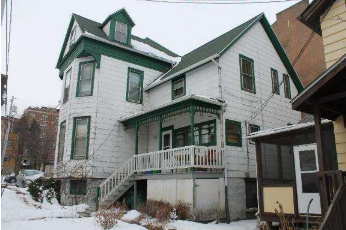
Photo 5: 9 North Hancock Street, Exterior, facing west
