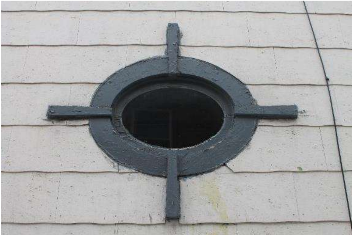
Photo 64: 8-10 North Franklin Street, Exterior, facing southeast
