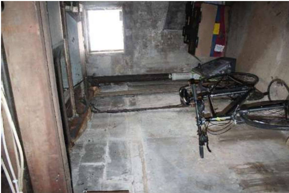
Photo 324: 410 1/2 East Washington Avenue, Interior, basement
