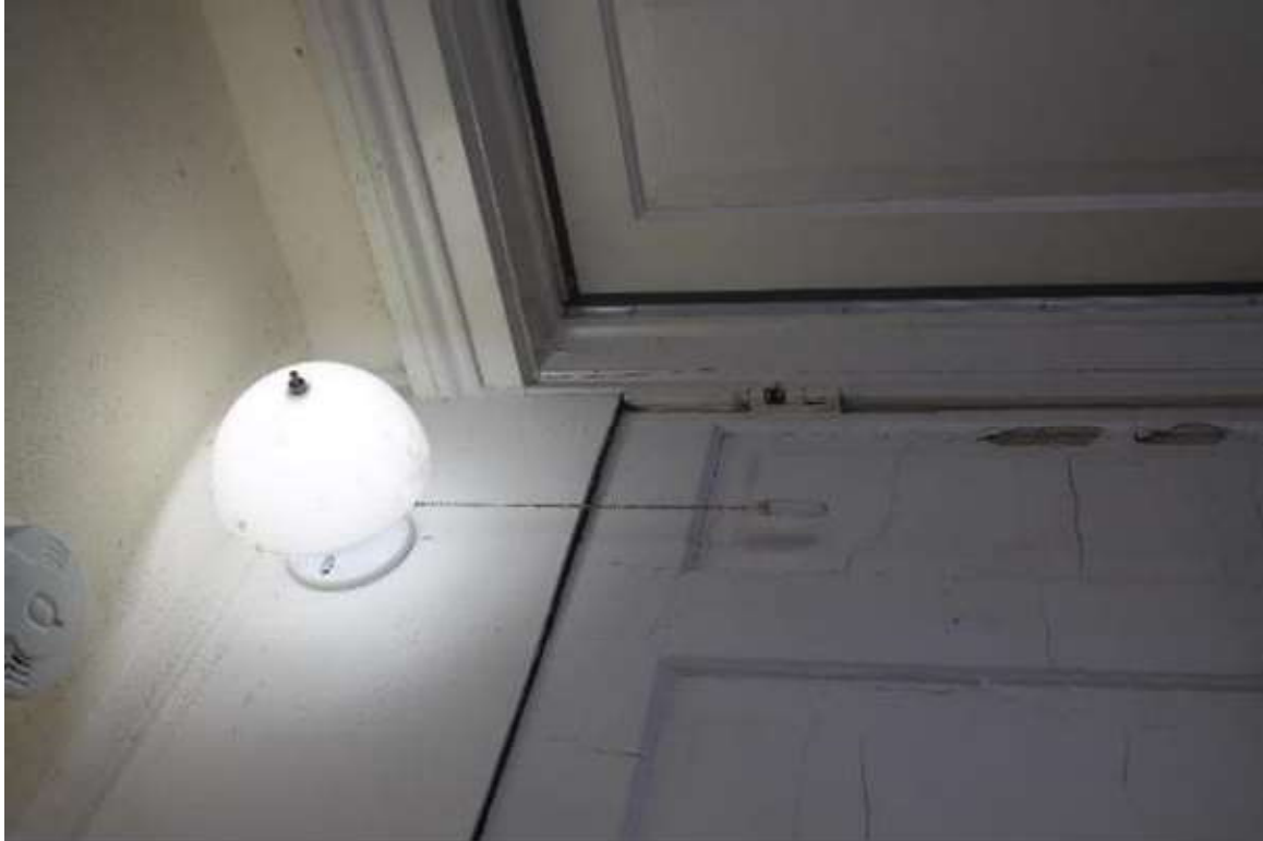
Photo 313: 410 1/2 East Washington Avenue, Interior, first floor entryway
