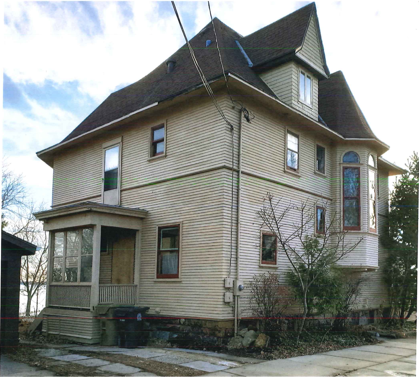
Rear of house from Jenifer Street looking south
