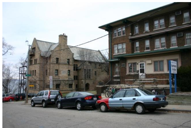
625-31 N. Henry (building on right) – proposed for demolition & 150 Iota Court
