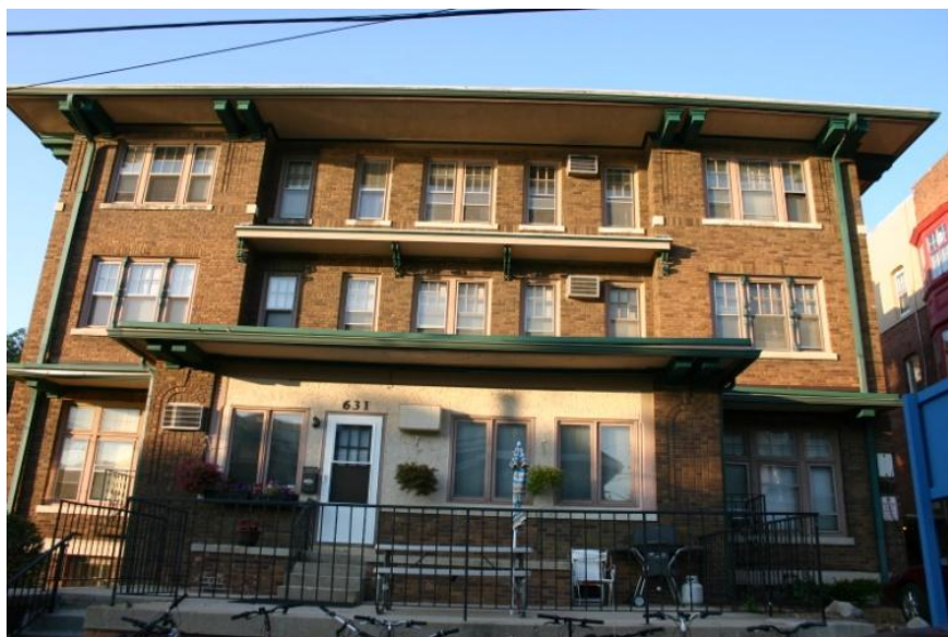
Another photograph of 625-31 N. Henry – proposed for demolition
