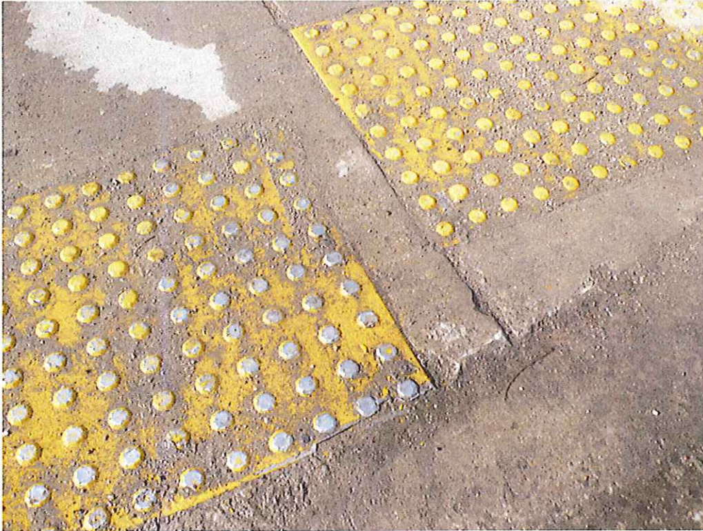
Stainless steel panel with surface wear. Beginning to tear on bottom corner creating sharp edges. Located on bike path.
