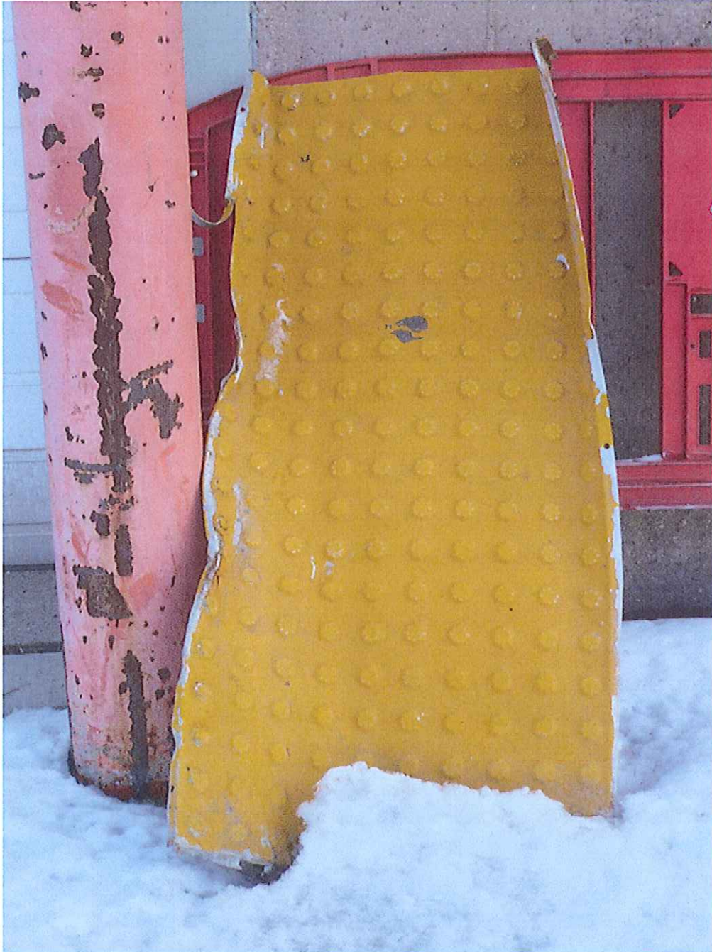
Stainless steel panel removed after citizen report of sharp and peeling edges
