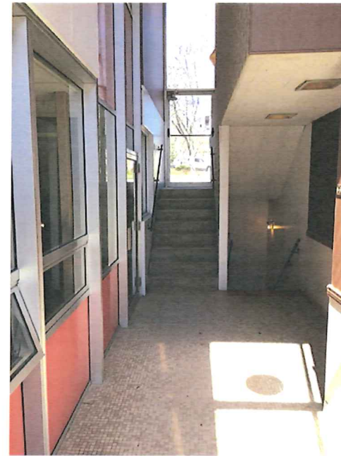
Office - Back Entry & Stairs
