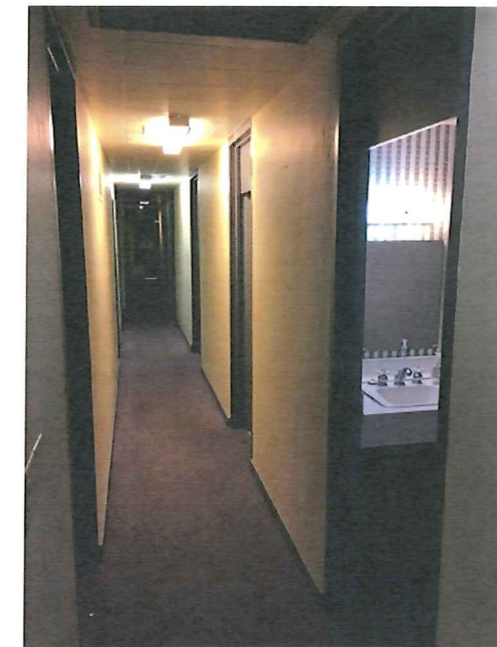
Office - Typical Corridor
