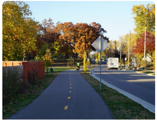
Prior to 2023, Dempsey Rd. and Davies St. lacked sidewalks or dedicated bikeways. Now, the corridor connects the neighborhood to the rest of Madison's active transportation network.
