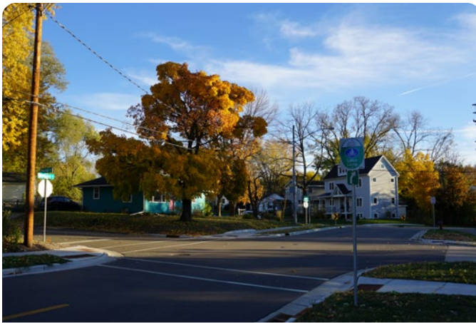
Five streets previously intersected at a single point. The reconstructed corridor now includes clear pavement markings, accessible curb ramps, and improved sightlines.
