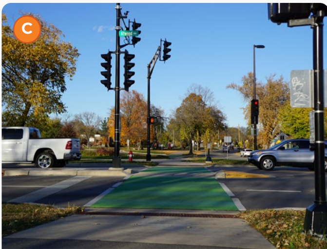
Figure C: Wide pedestrian-bike crossings at Atwood Ave. and Walter St.
