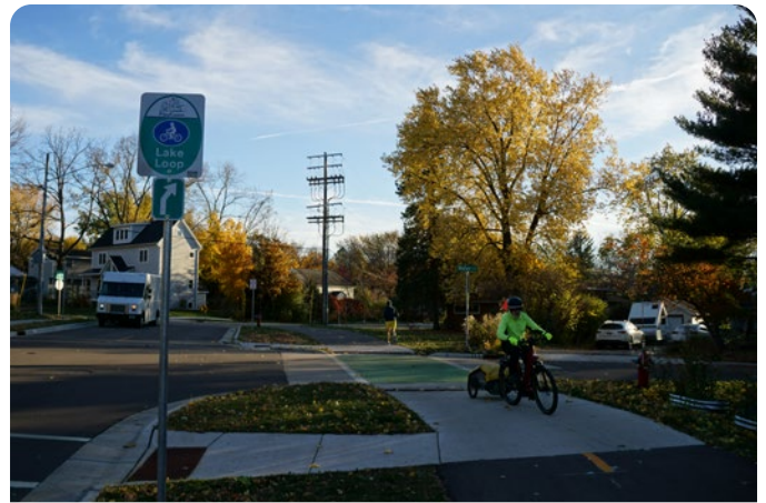
Raised crossings along the new shared-use path improve bike and pedestrian safety and comfort while making path users more visible to cars.
