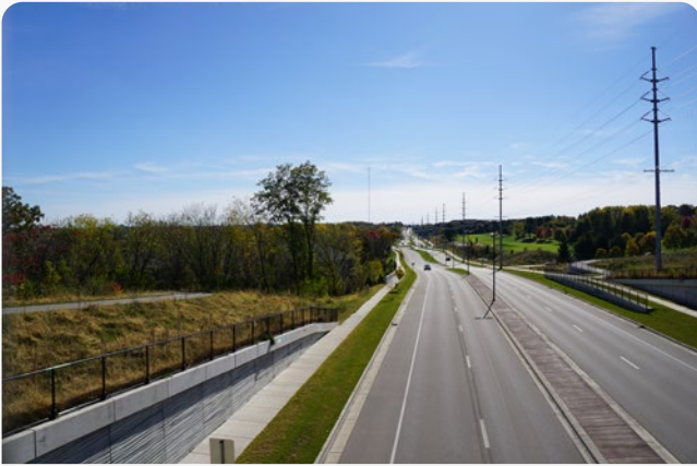
After: Pleasant View Road following its reconstruction. Photo taken from shared-use path bridge, which connects to Greenway Station.
