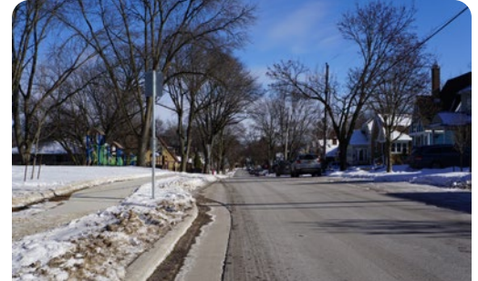
The narrowed street makes way for a new sidewalk and slows car traffic down.
