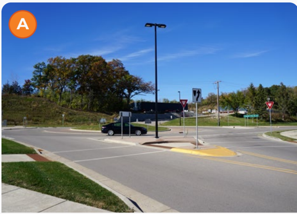
Figure A: Refuge Islands at roundabouts and lighting improvements keep path and sidewalk users visible and comfortable.
