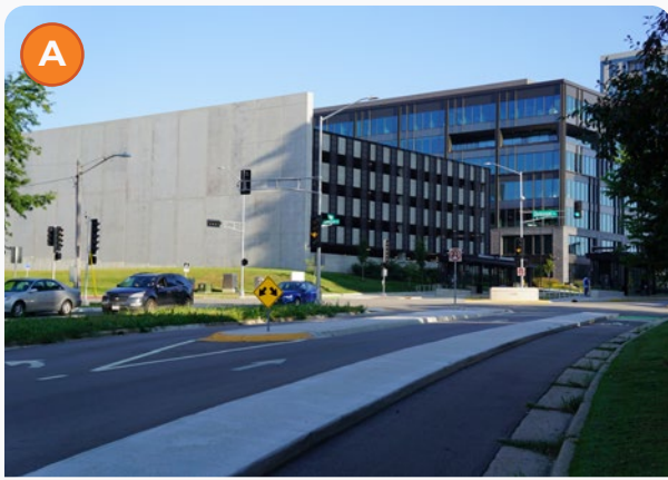
Figure A: Separated turn lane and protected bike lanes calm traffic at the intersection of Segoe Road and Sheboygan Avenue.
