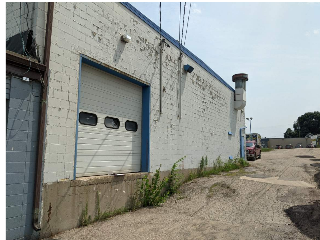
REAR FAÇADE (WEST)
