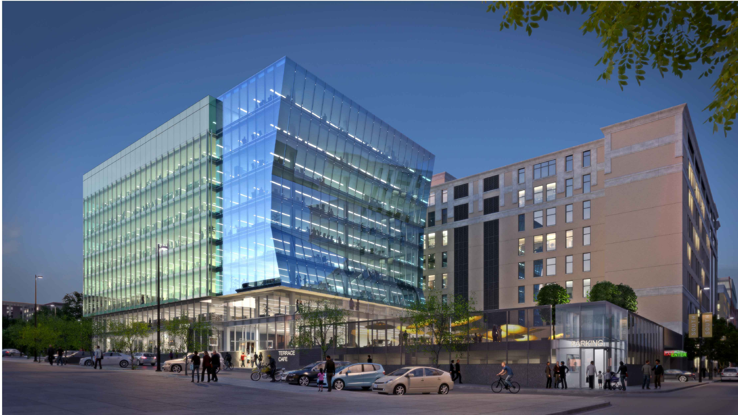
ANCHOR BANK building DECEMBER 12, 2012
