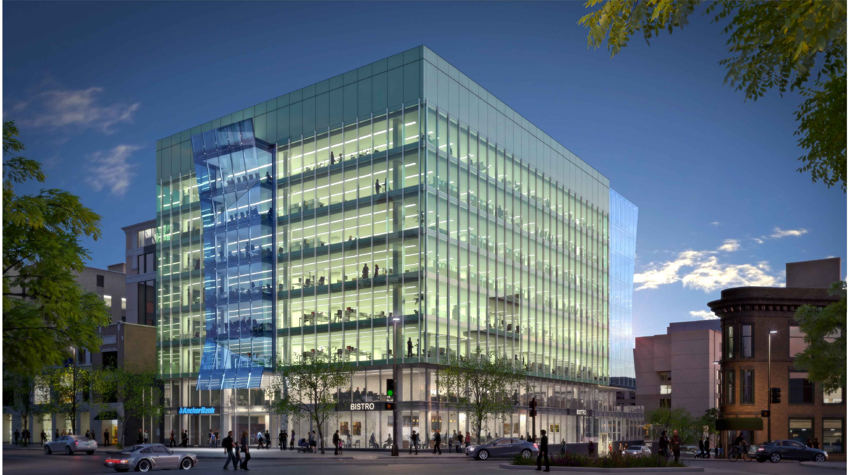
ANCHOR BANK building DECEMBER 12, 2012
