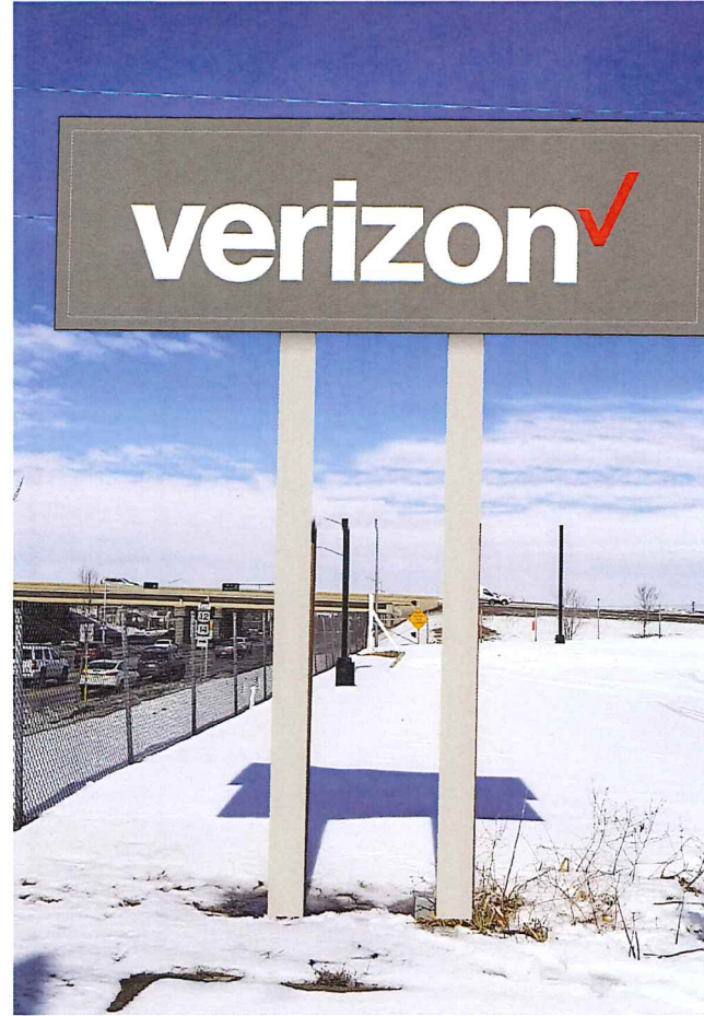
READERBOARD CABINET TO BE REMOVED. EXISTING STEEL POSTS TO BE UPDATED TO SW 7075 WEB GRAY.
