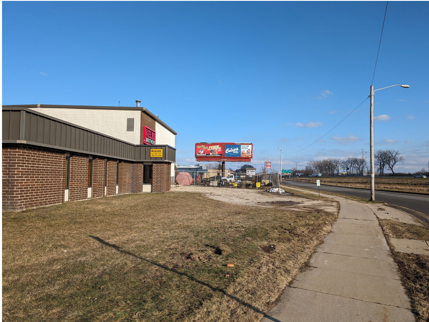
South Elevation – View from E Broadway St
