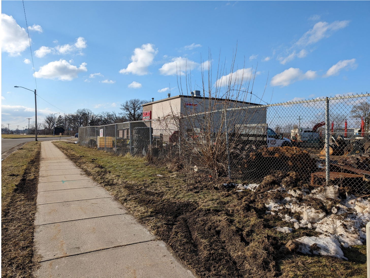
South Elevation – View from E Broadway St
