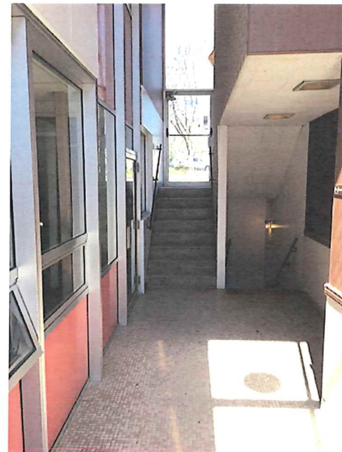
Office - Back Entry & Stairs
