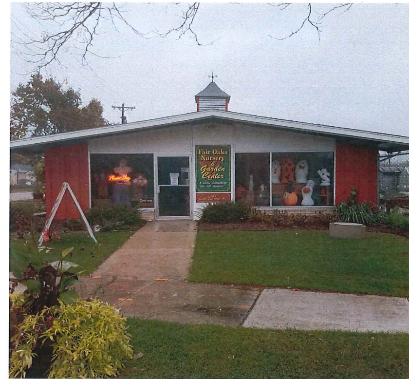
View from S. Fair Oaks Avenue
