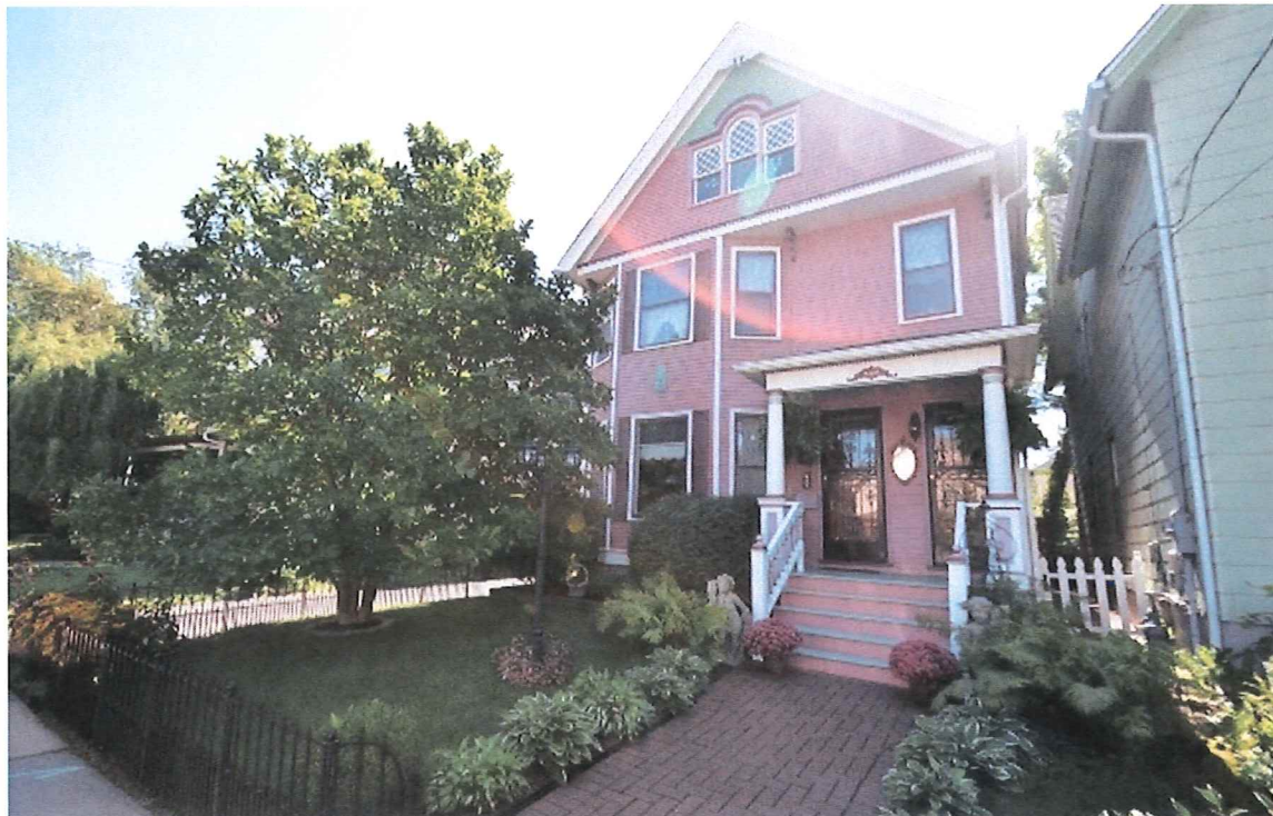
Street front view of home. This view also shows the close proximity of the neighboring property.
