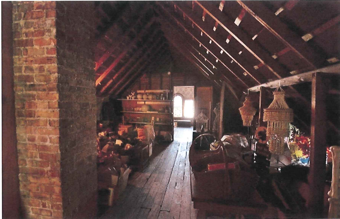
View of the existing unfinished attic space
