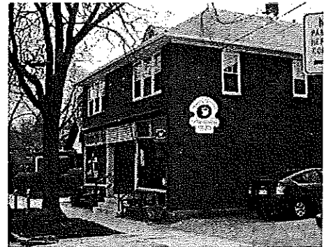
This coffee shop and cafe on Allen Street is part of a Neighborhood Mixed Use District at the corner of Regent and Allen Streets.
