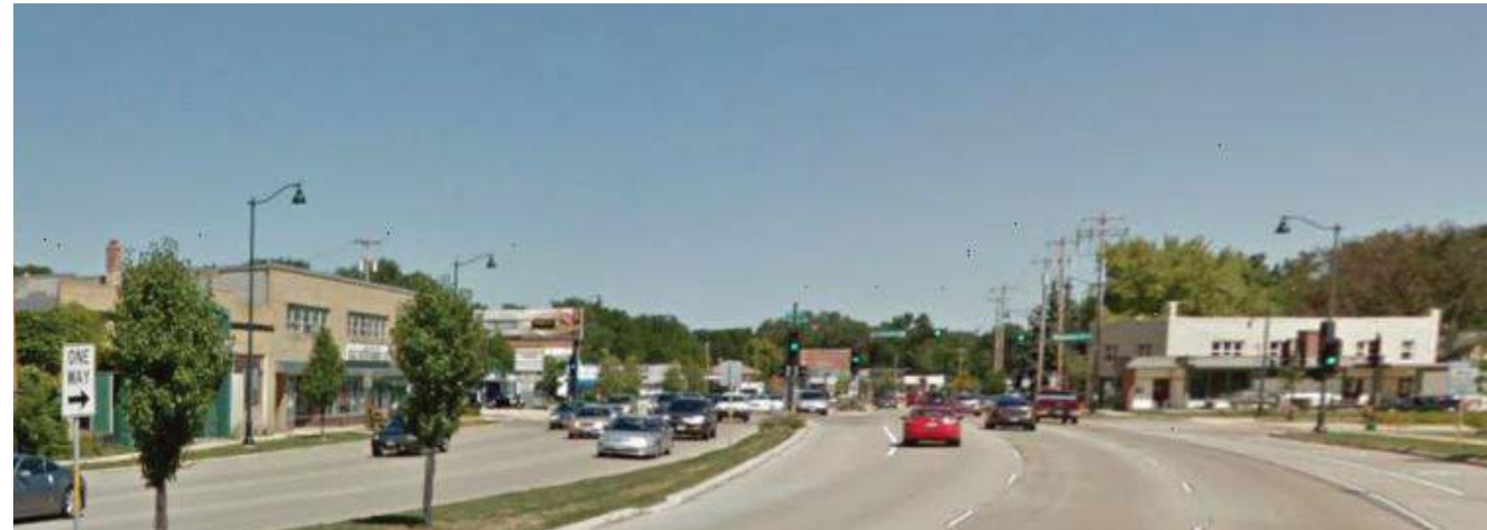
7th Street and E. Washington Ave. - Looking North
