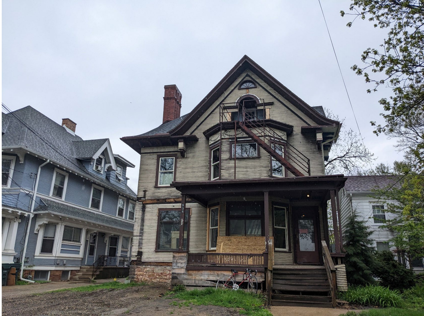
Front South Elevation – View from Spaight St
