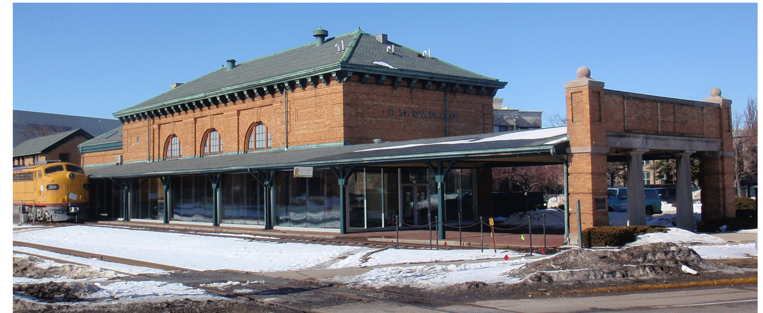
PHOTO OF EXISTING BUILDING
