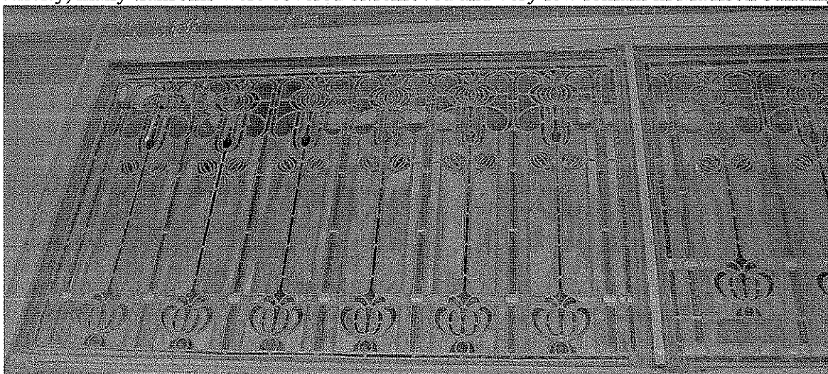
Fig. 4: the transom window at 120 W. Mifflin in 2006.
