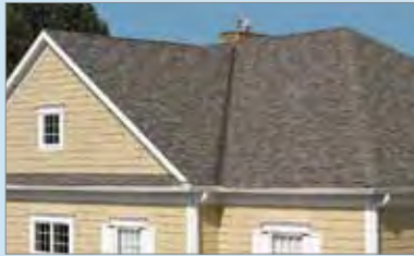
Roofing and Ventilation
