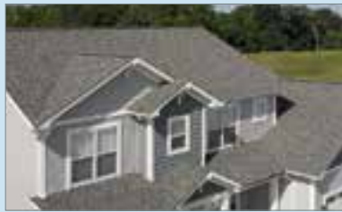
Roofing and Ventilation
