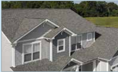
Roofing and Ventilation
