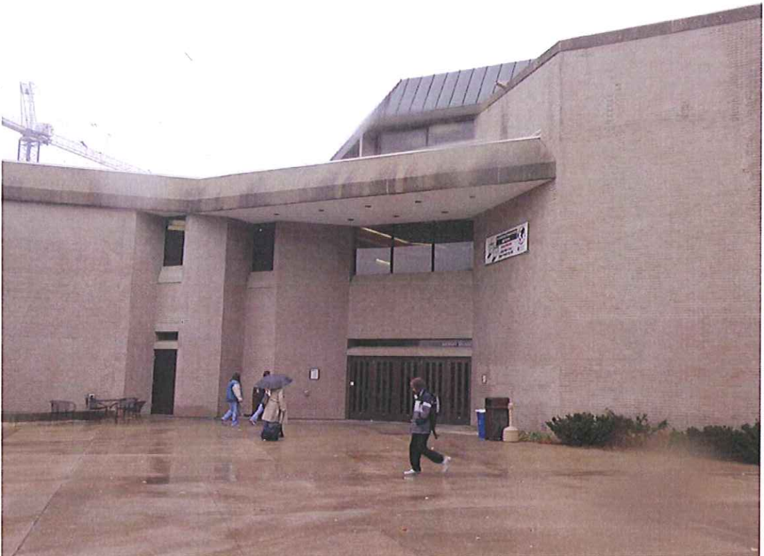
Union South West façade and entry from off N. Randall Avenue (main entry)
