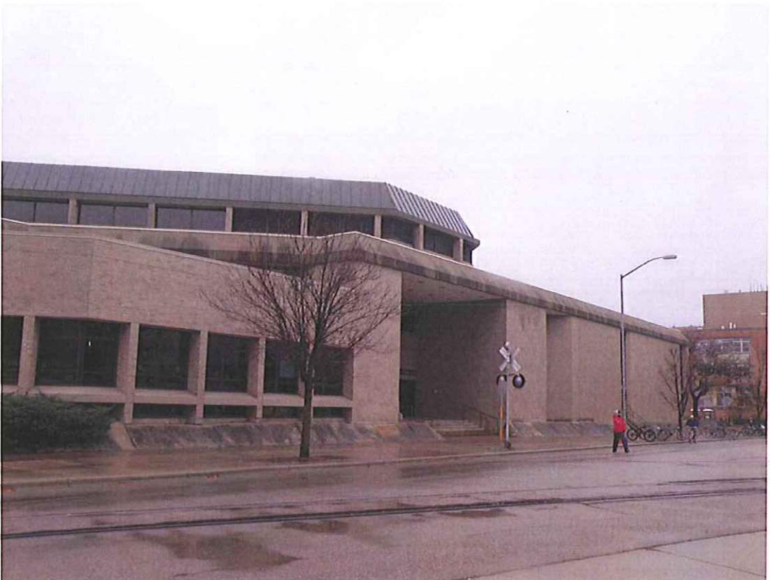
Union South North façade along W. Johnson Street and rail road tracks
