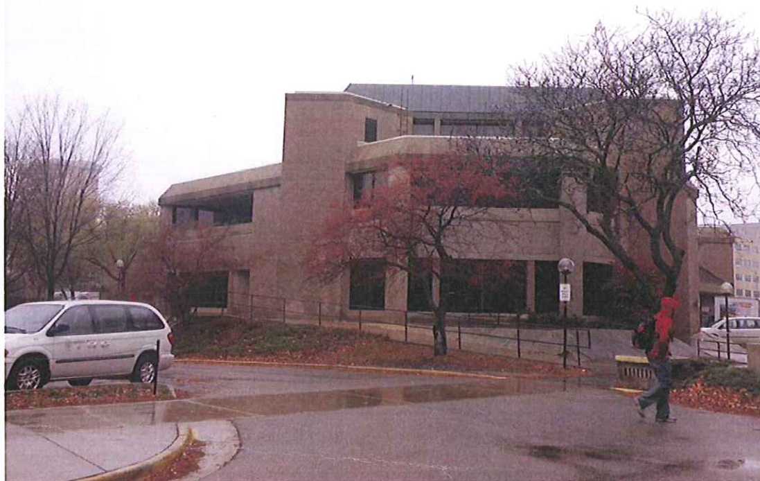
Union South View from southeast along vacated N. Orchard Street
