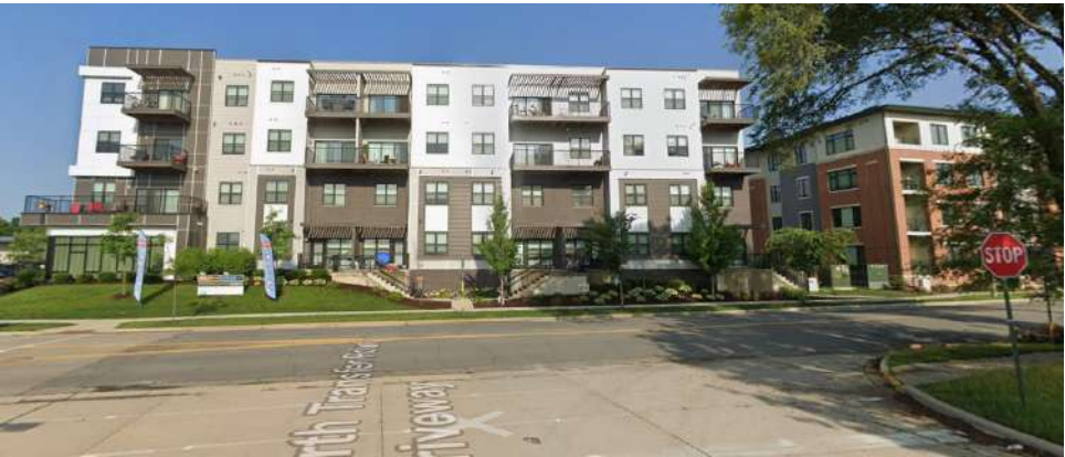
Building Across: 1201 Huxley St
