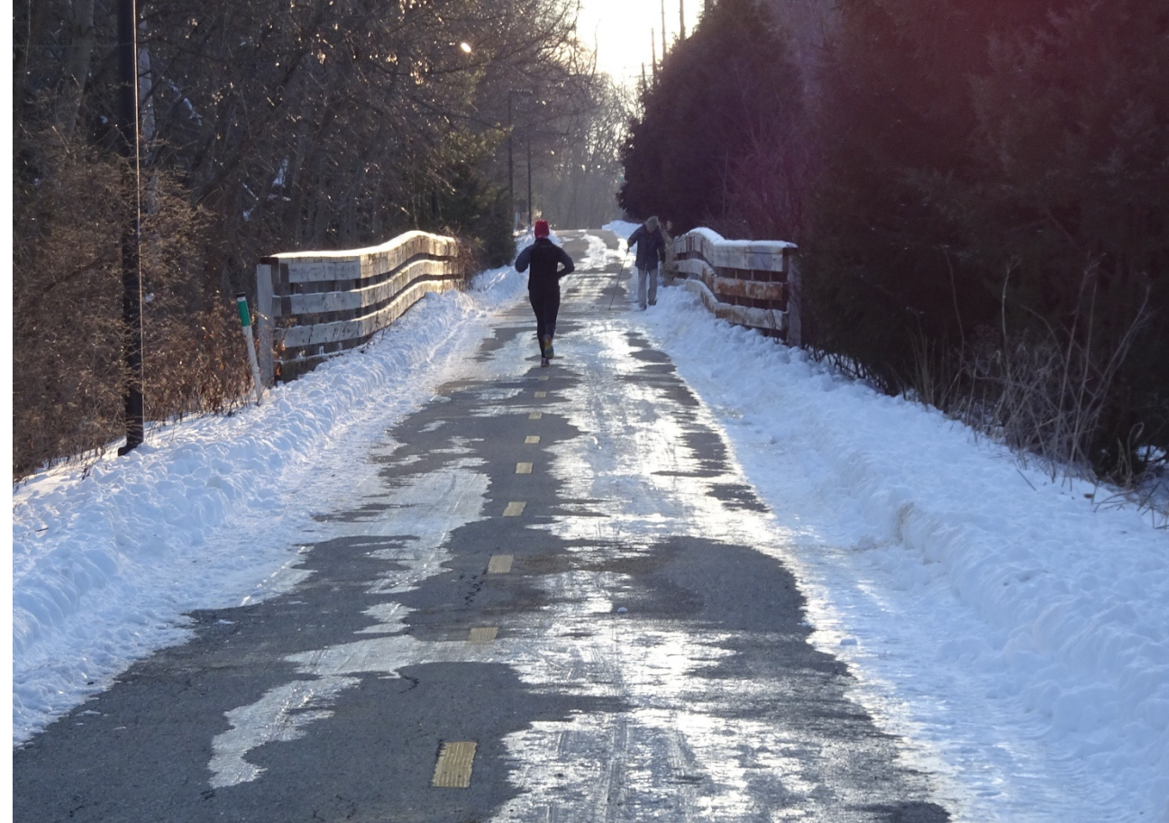
Dec 31- Treacherous glare ice on entire brine-treated span
