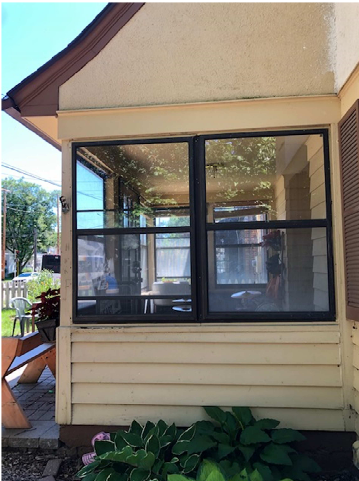
RIGHT SIDE VIEW OF ENTRY "BOX"
