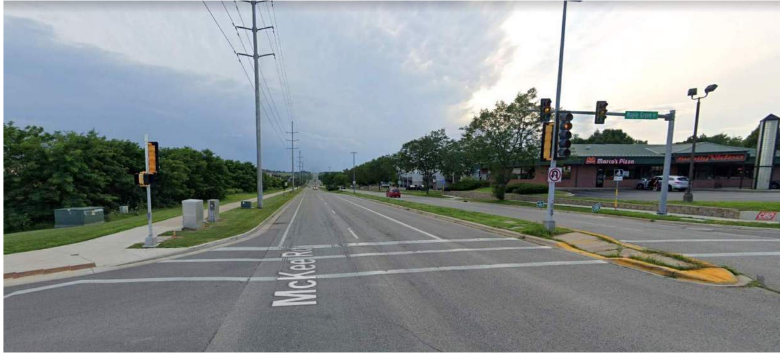
NORTHEAST CORNER - McKEE RD (LOOKING WEST)
