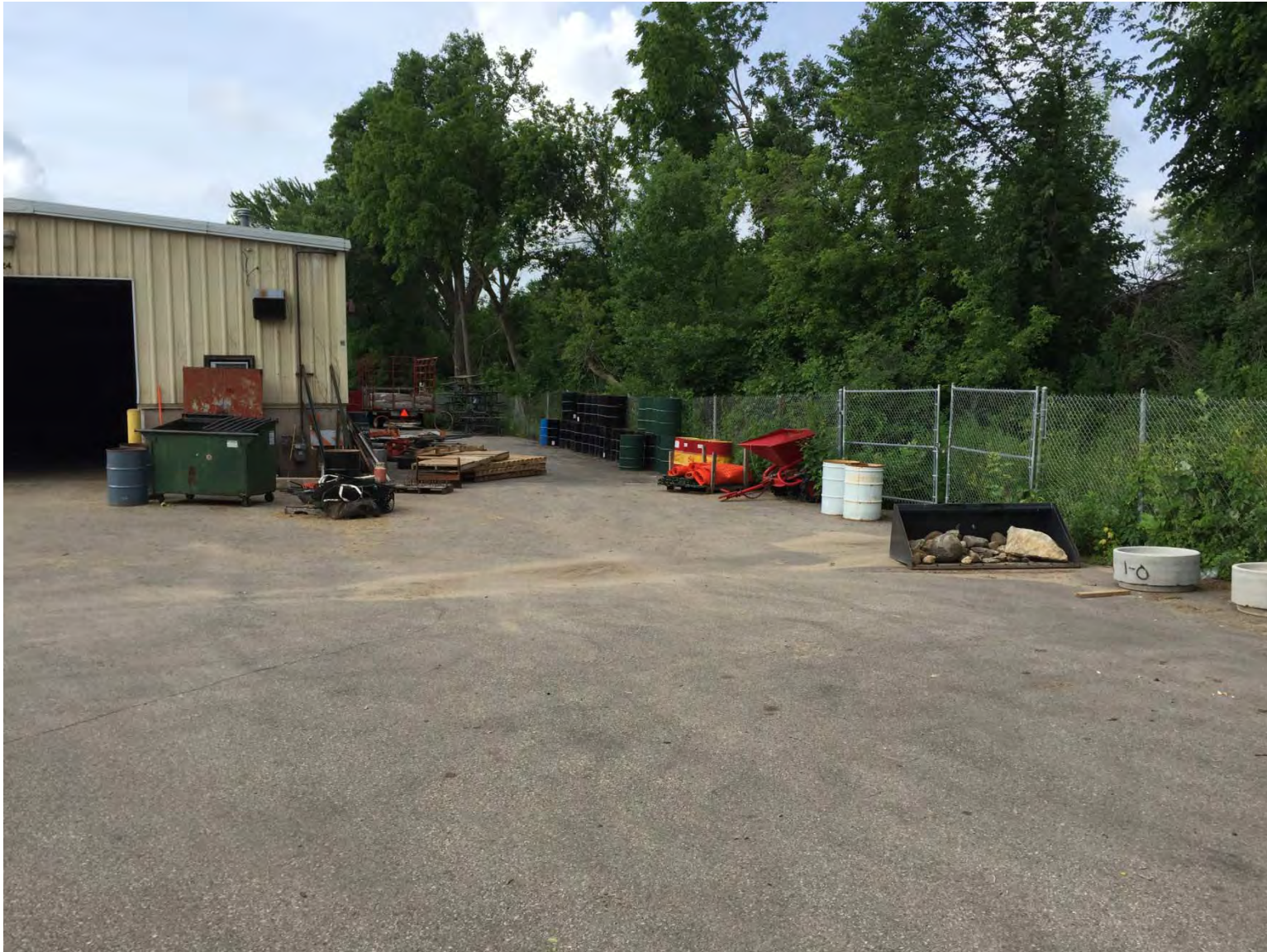
Parks Goodman Yard M-6: Parking Lot Drainage to Swale
