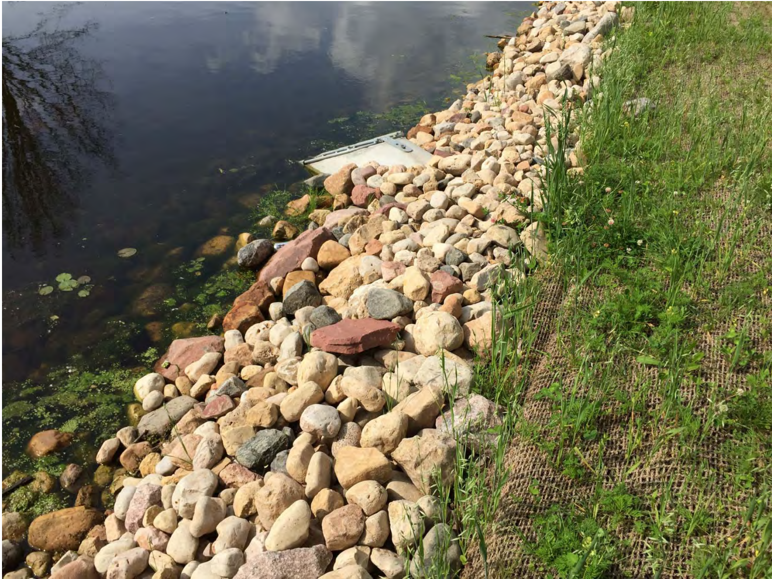
Parks Goodman Yard M-14: Outfall to Creek
