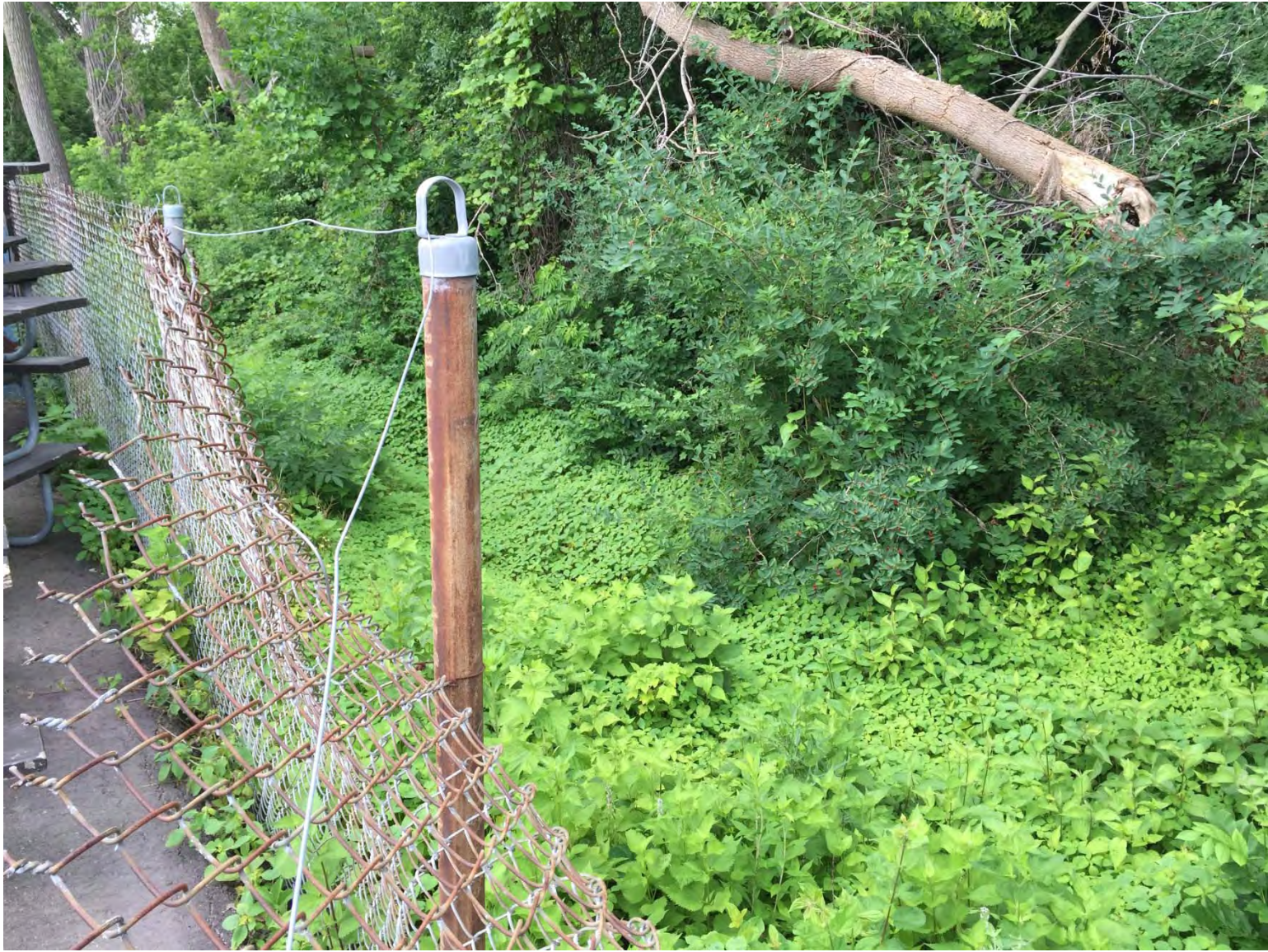
Parks Goodman Yard M-8: Drainage Ditch
