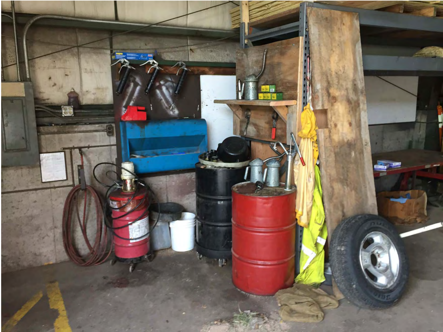
Parks Goodman Yard B3-1: Indoor Waste Oil Storage
