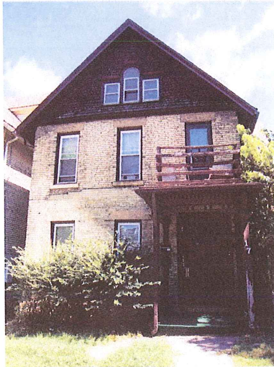
Front of 17 N. Webster Street. The rear portion of this house is the original section. The front addition was constructed sometime later.
