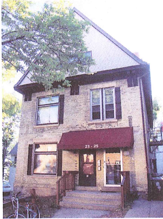
Front view 23/25 N. Webster Street. Original front porch and related details removed.
